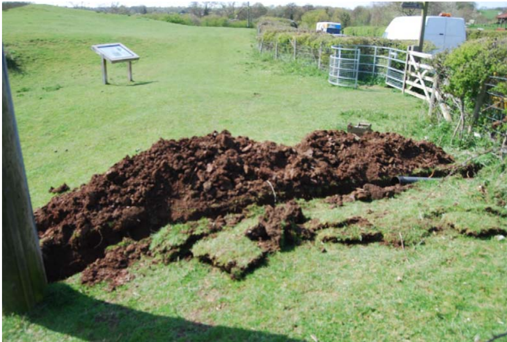
Plate 3 Excavation of service trench
