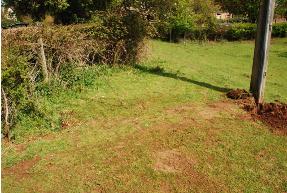
Plate 5 Service trench backfilled, facing north
