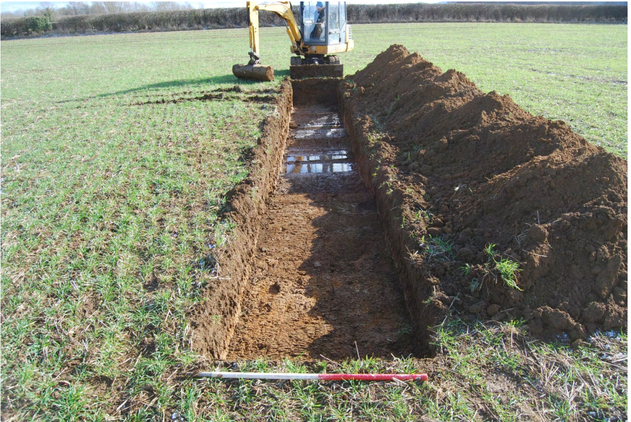
Trench 7 facing south-east (1m scale)
