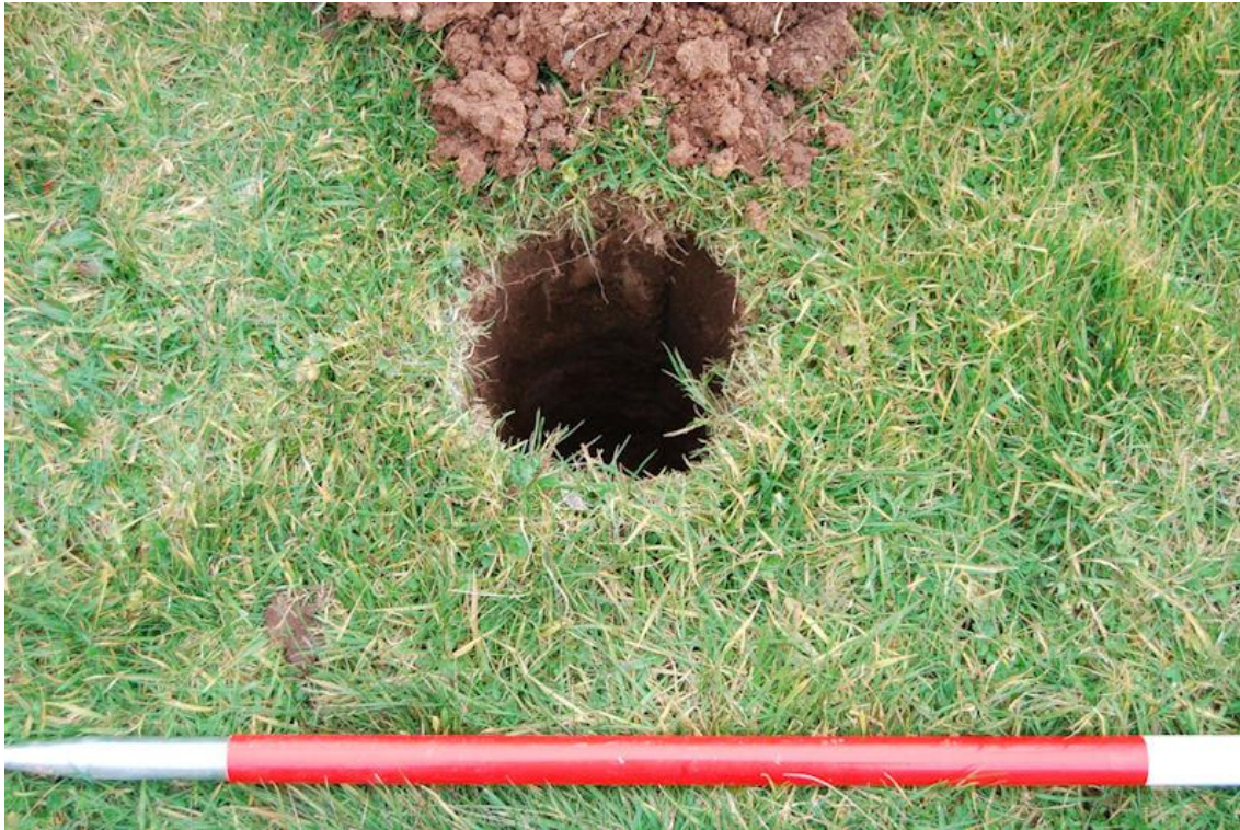
Plate 5: Posthole cut for new location of Panel 16, view east
