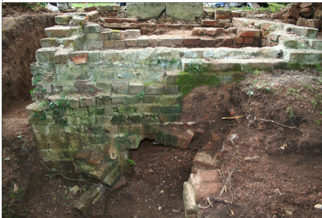
Figure 12. NW wall, with arched discharge from cess chamber above the ditch.
