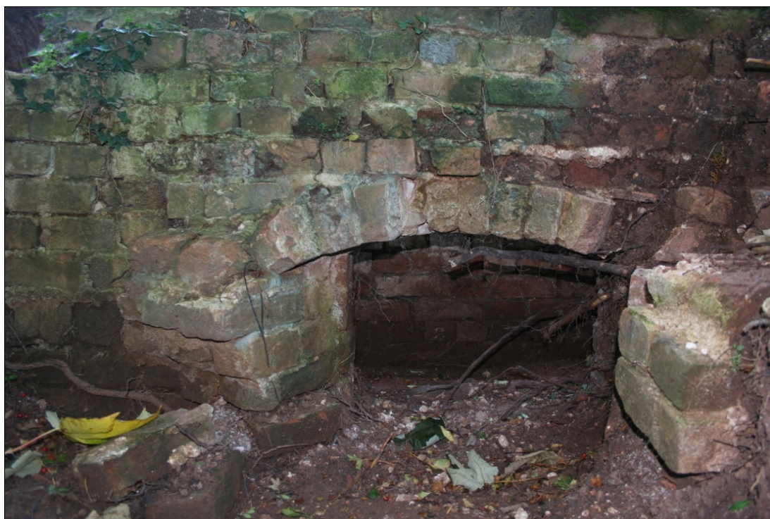
Figure 13. Brickwork around discharge from cess chamber.
