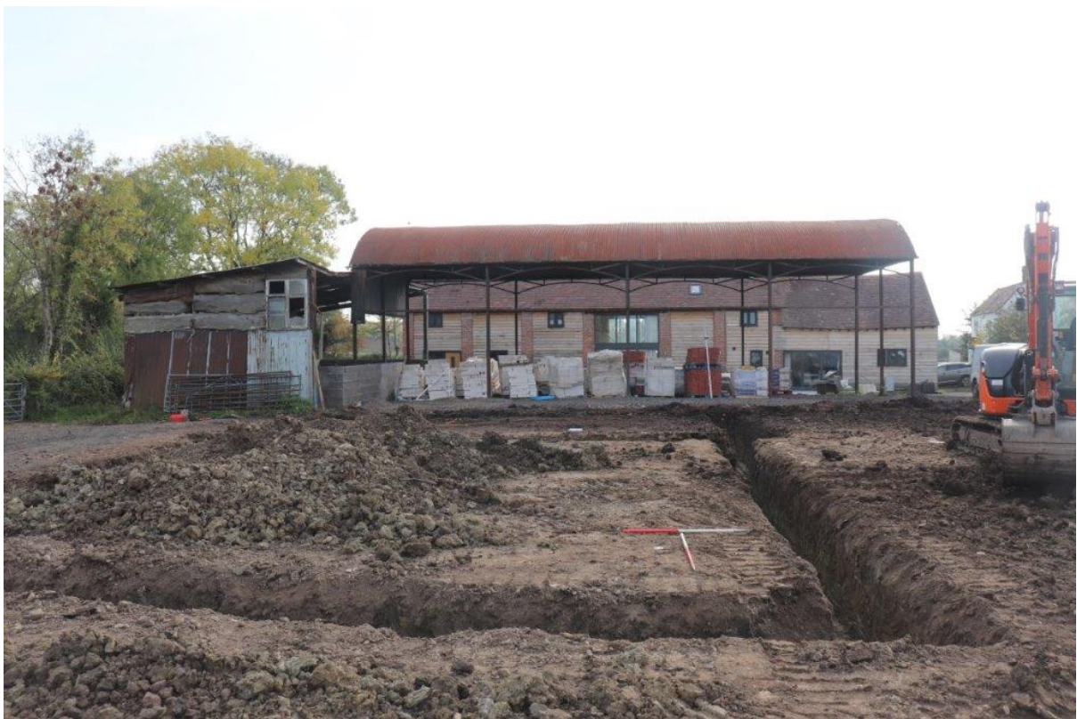
Plate 8: Foundation trenches complete, view south-east, 2x 1m scales
