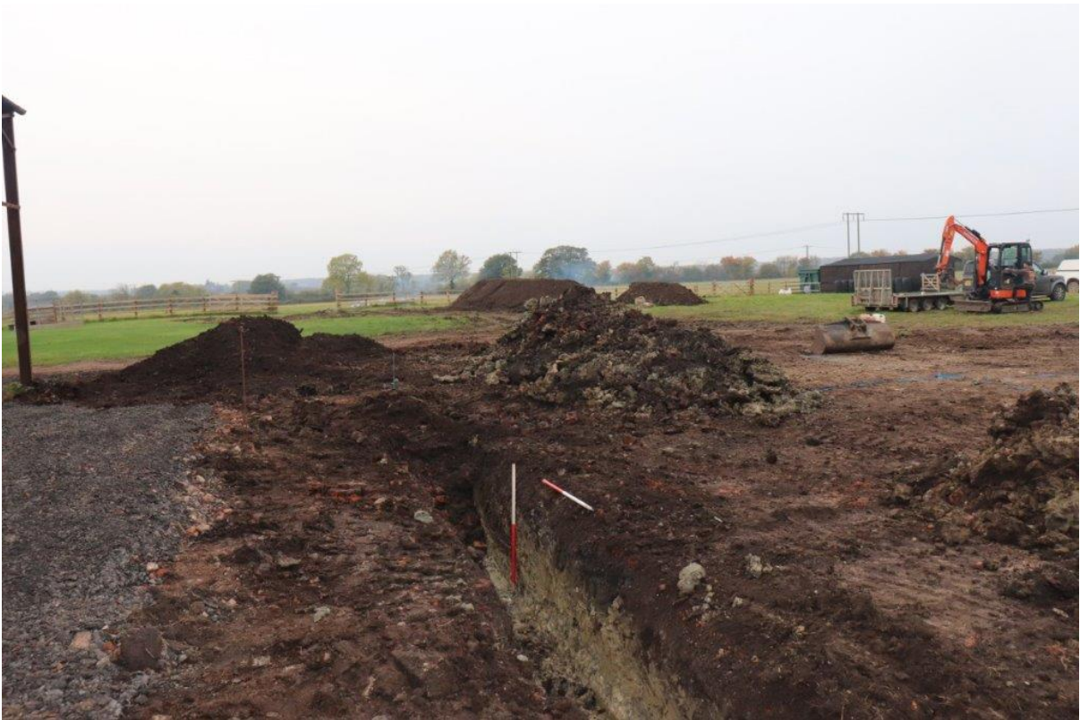
Plate 2: Southern trench showing made ground and brick surfacing, view west, 2x 1m scales
