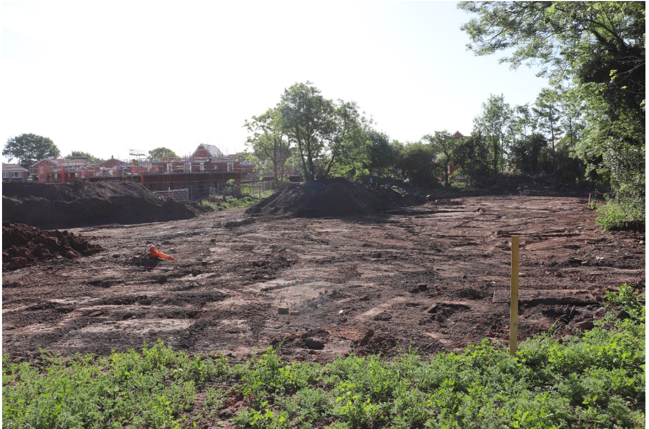
Plate 9: The watching brief stripped area, looking south-west, scale 1m
