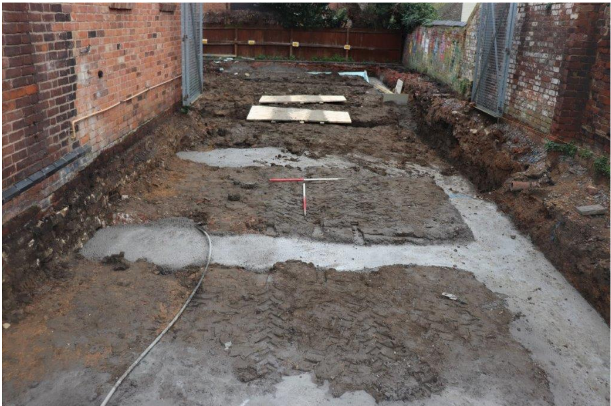
Plate 8: Foundation trenches excavated and concreted; view north, 2x 1m scales
