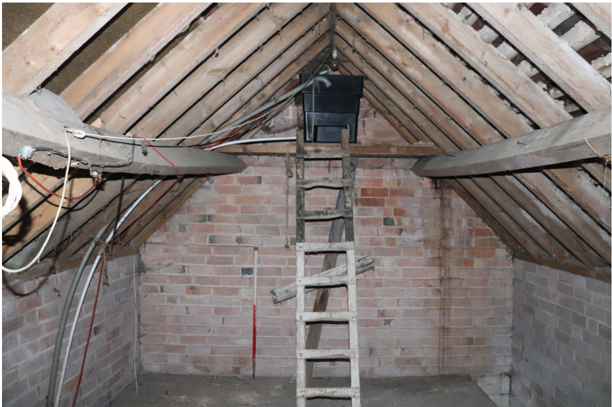
Plate 6 The first floor, view west, scale 1m
