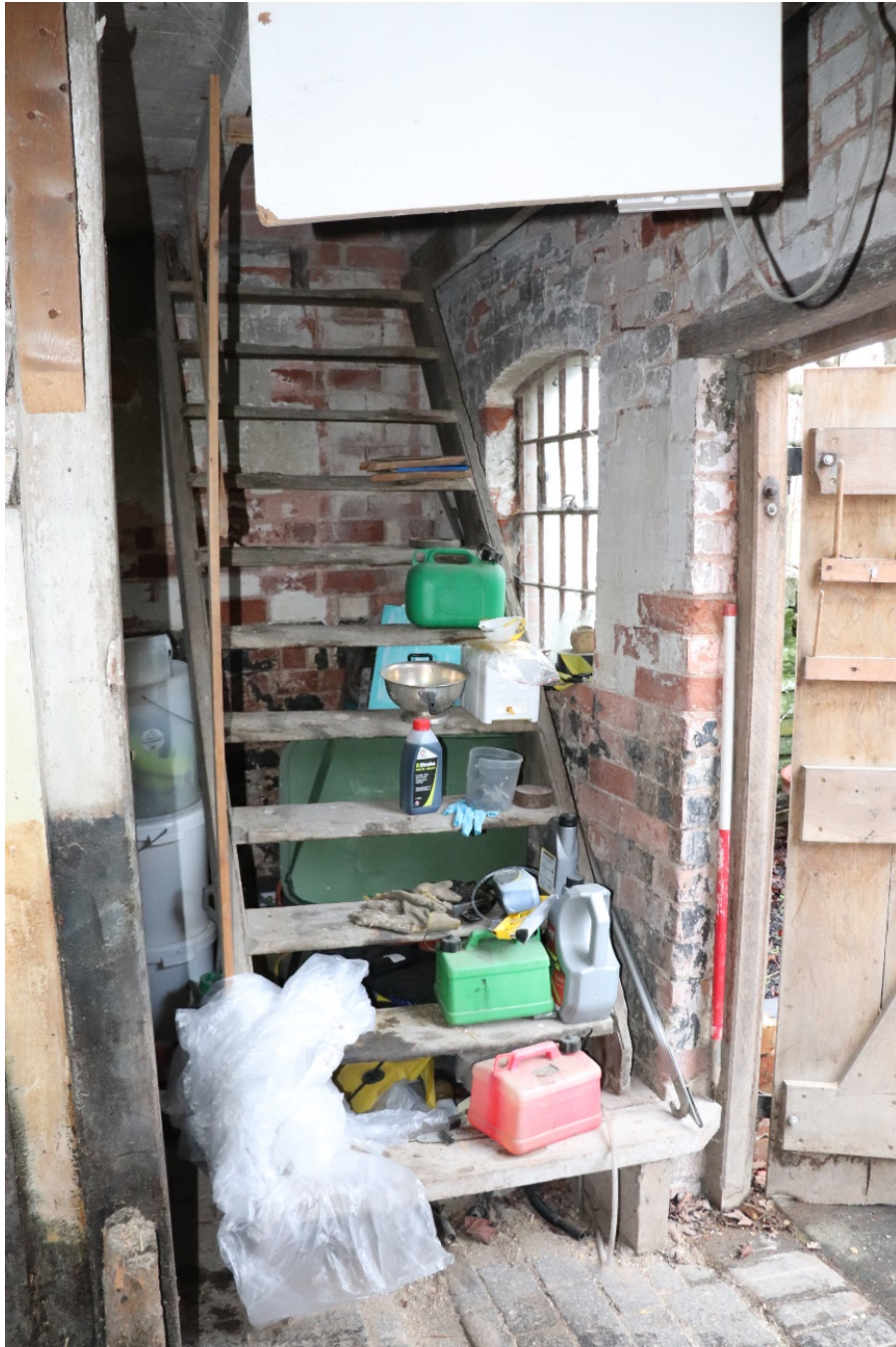
Plate 9 Phase 3 stairs, view east, scale 1m
