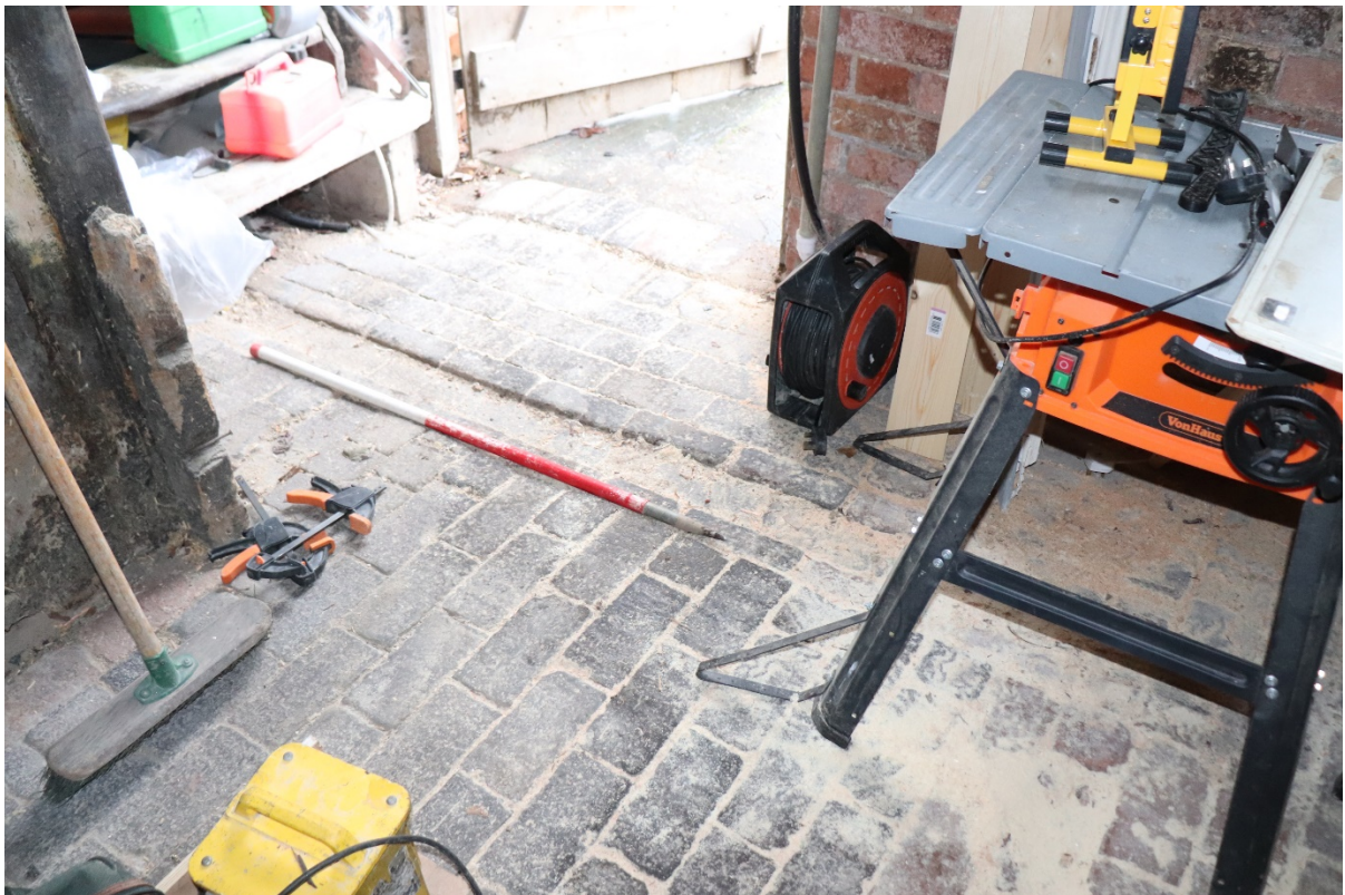
Plate 4 Internal drain, view south-east, scale 1m
