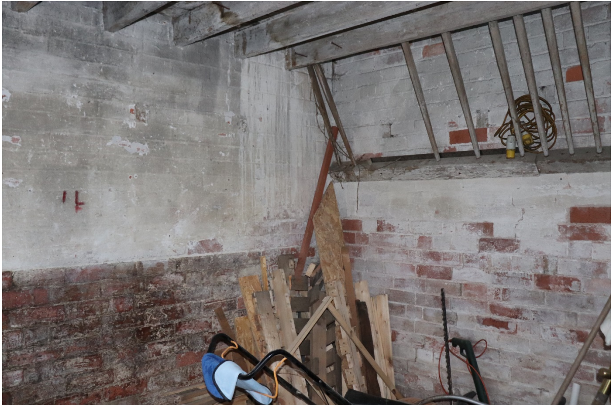
Plate 5 Timbers set into the wall, view north-west, no scale
