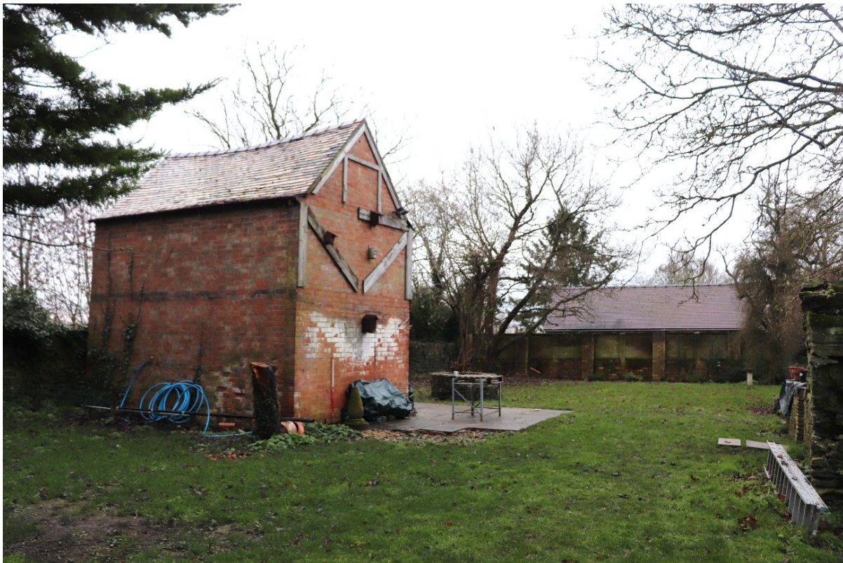
Plate 2 The building, general view south-west, scale 1m
