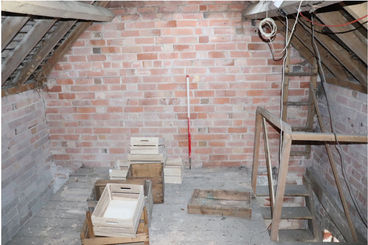
Plate 7 The first floor, looking east, scale 1m
