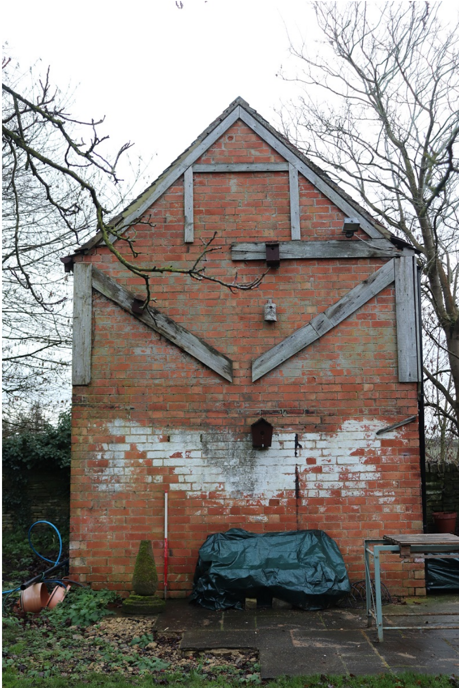
Plate 10 The building, west gable elevation, view east, scale 1m
