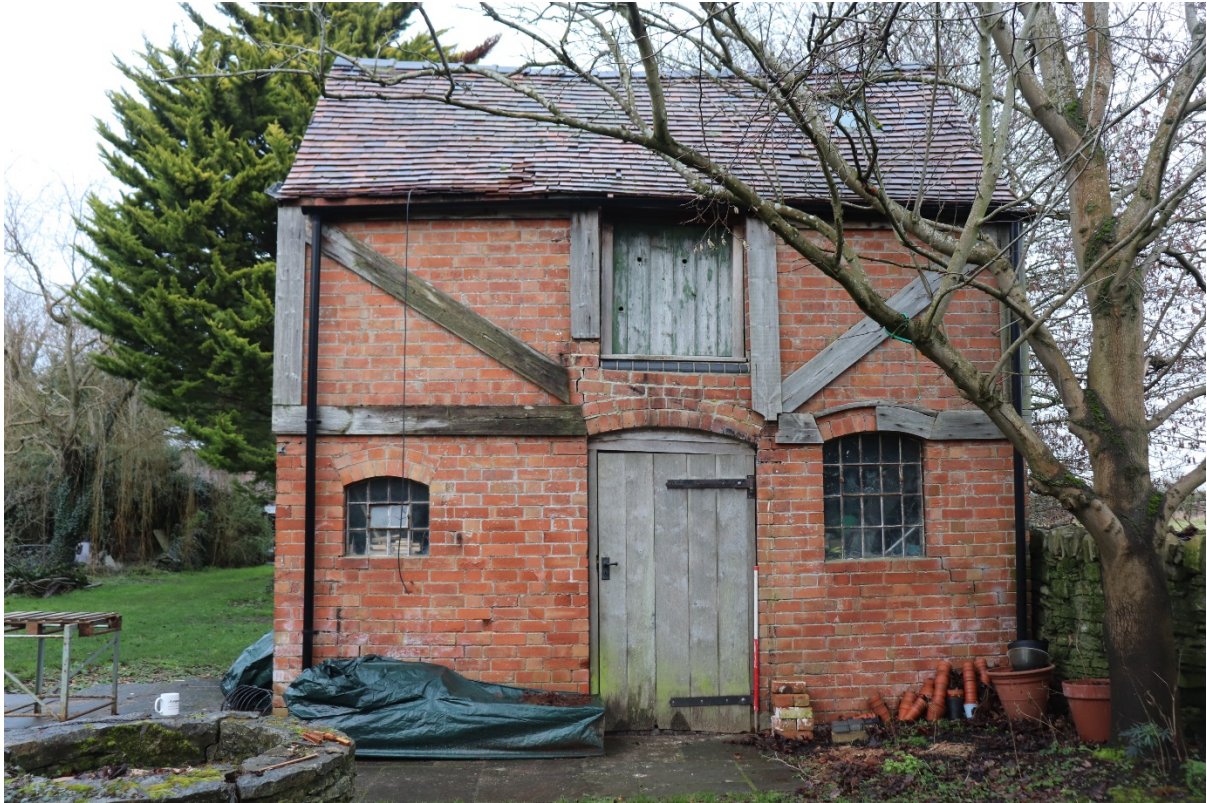
Plate 3 The building, south elevation, view north, scale 1m
