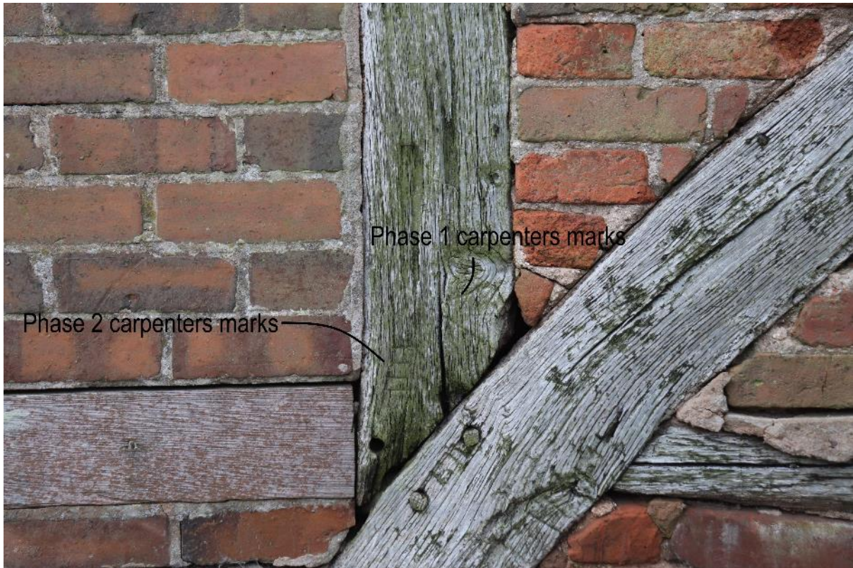
Plate 9 Phase 1 and 2 carpenters marks, looking south
