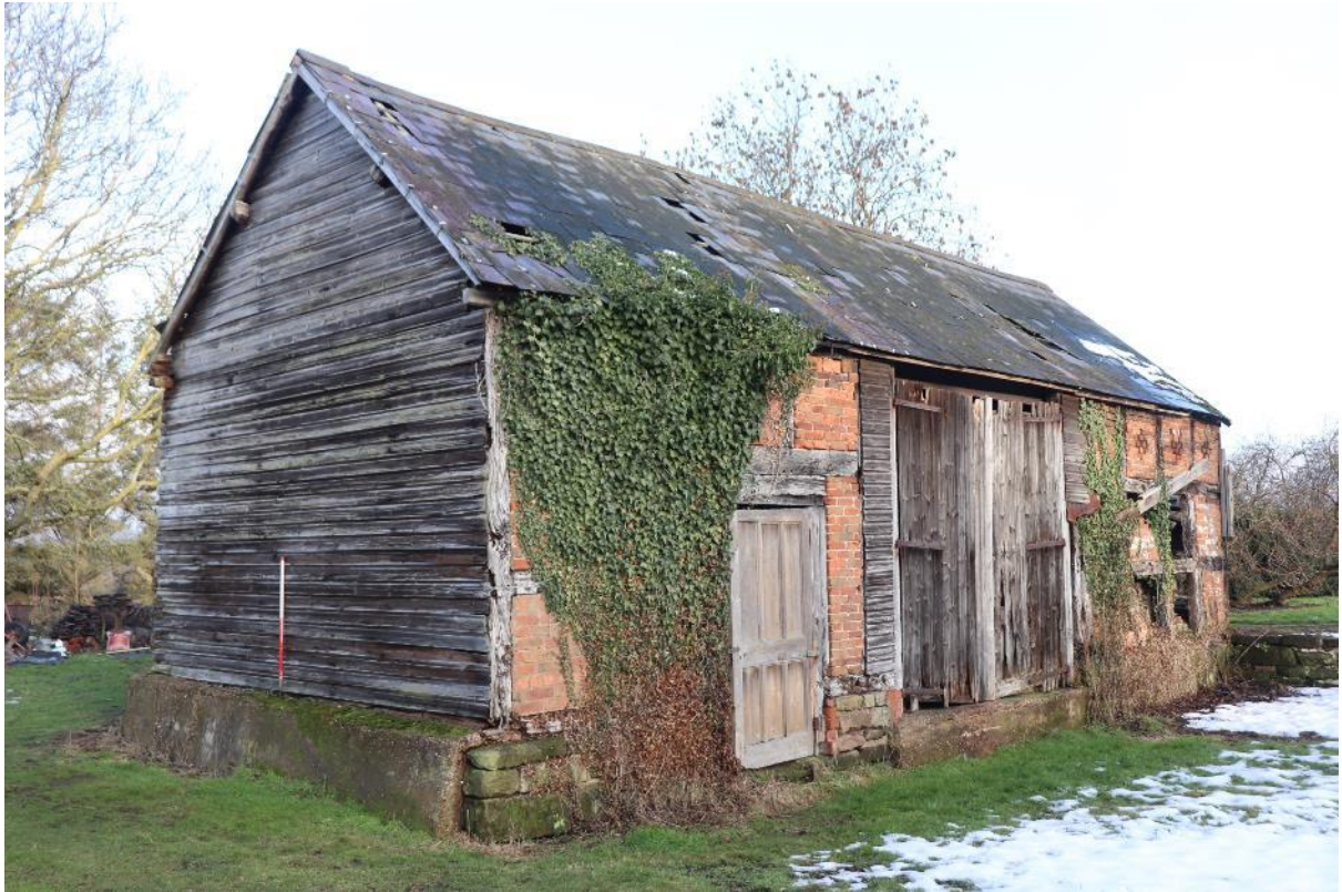
Plate 7 Phase 1 barn, looking north-east, scale 1m
