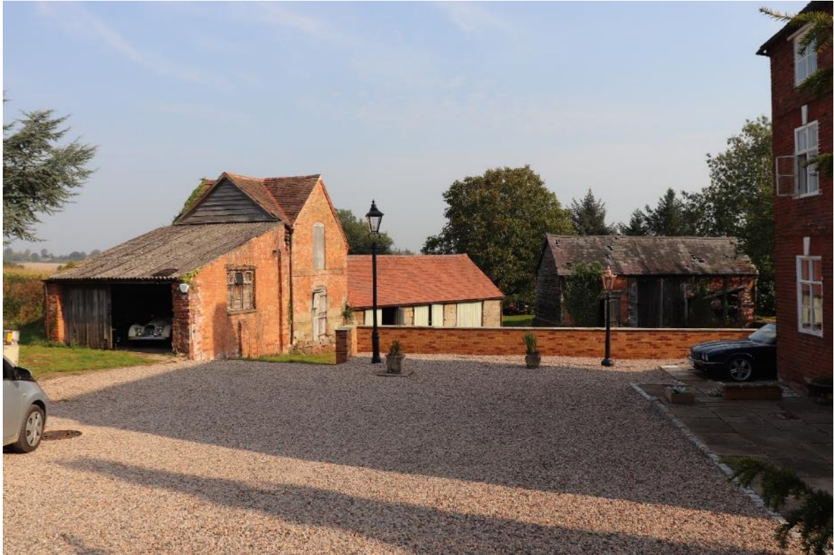
Plate 5 The buildings, looking north
