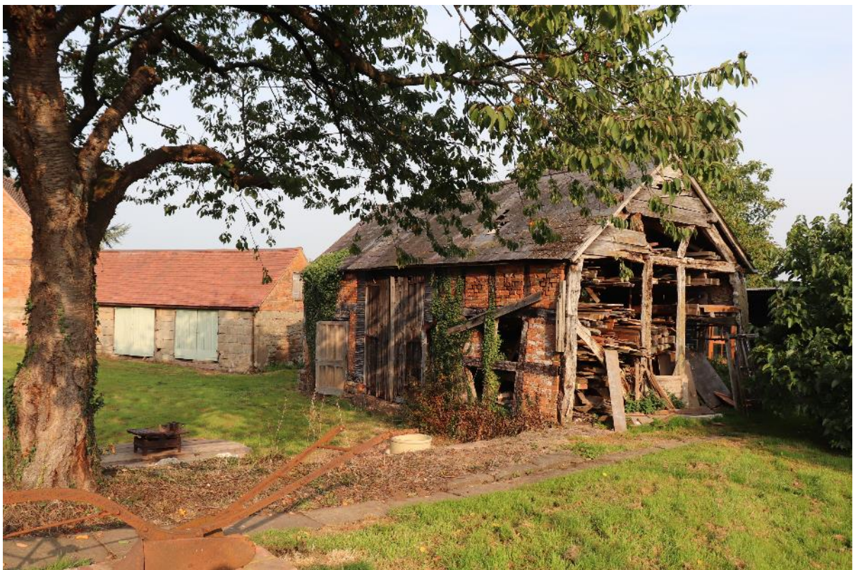
Plate 2 Phase 1 barn, looking north-west
