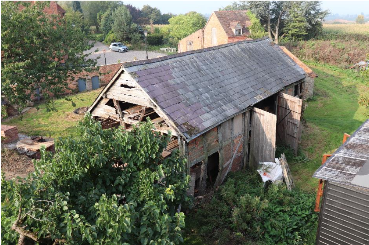
Plate 1 Phase 1 barn, looking south-west
