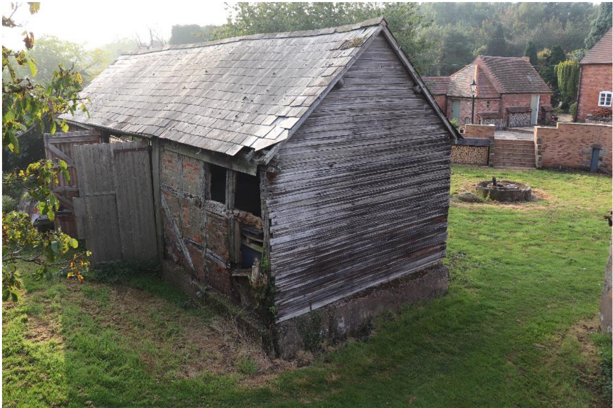
Plate 6 Phase 1 barn, looking south-east
