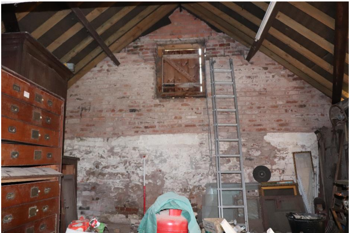
Plate 18 Phase 3b cow shed, looking north-east, scale 1m
