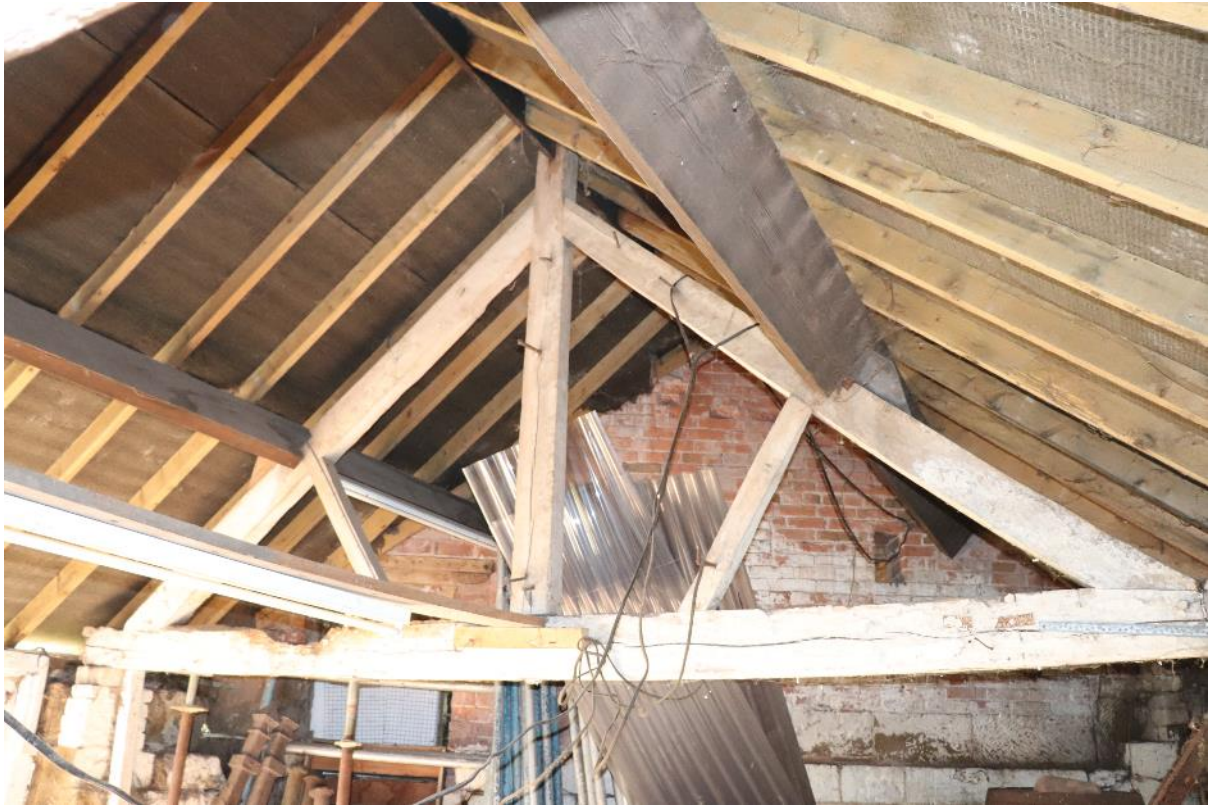
Plate 17 Phase 3b cow shed roof truss, looking south-west
