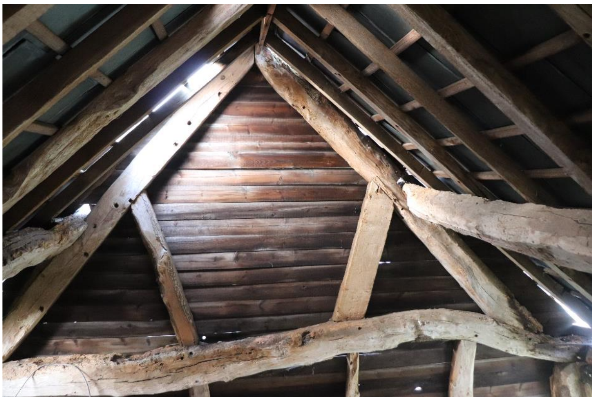
Plate 10 Phase 2 west end truss, looking west
