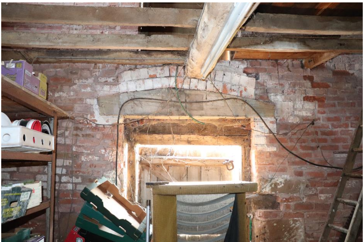
Plate 14 Phase 3a dovecote with evidence for the door and floor beam having been raised, looking south-east
