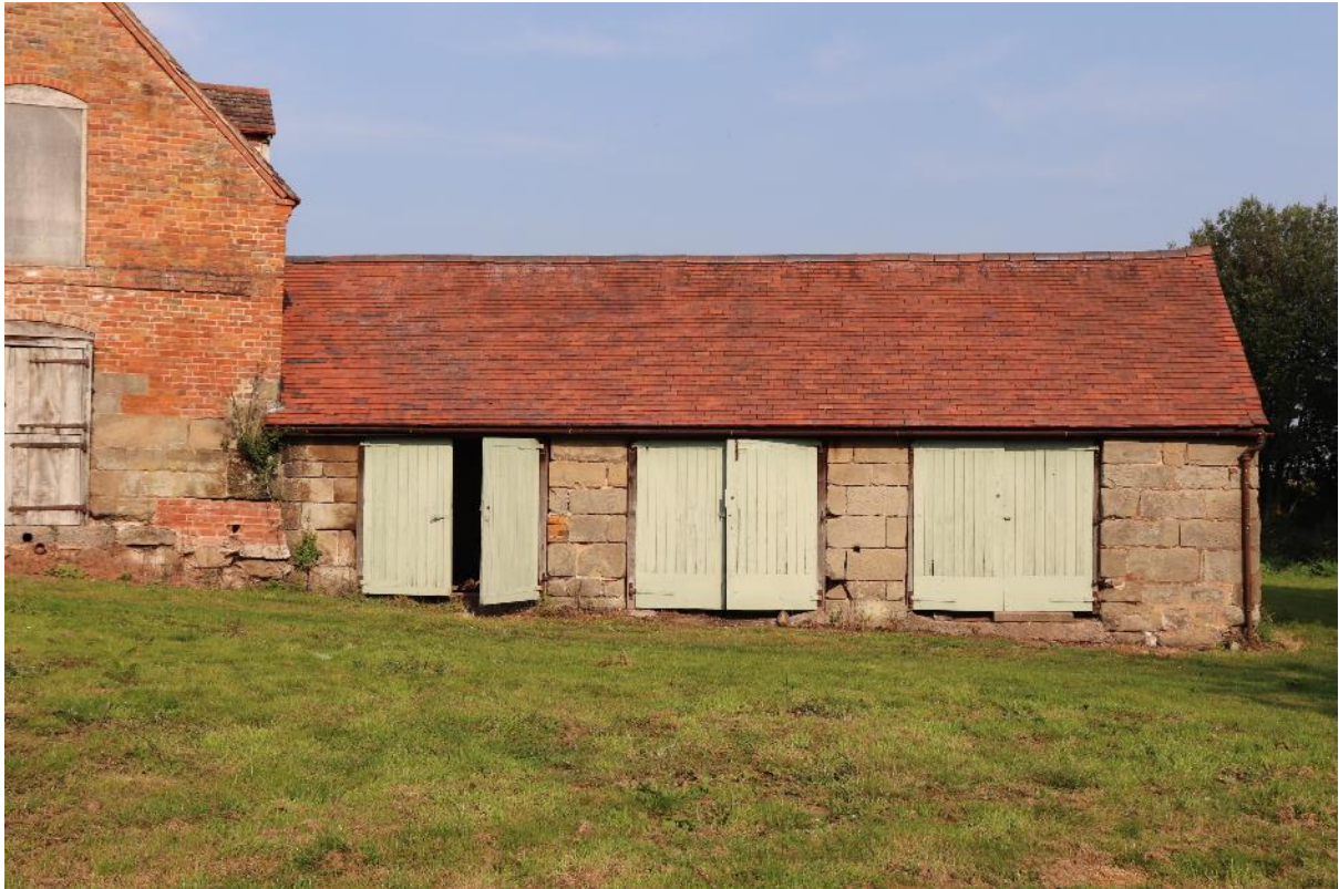
Plate 3 Phase 3b cow shed, looking north-west
