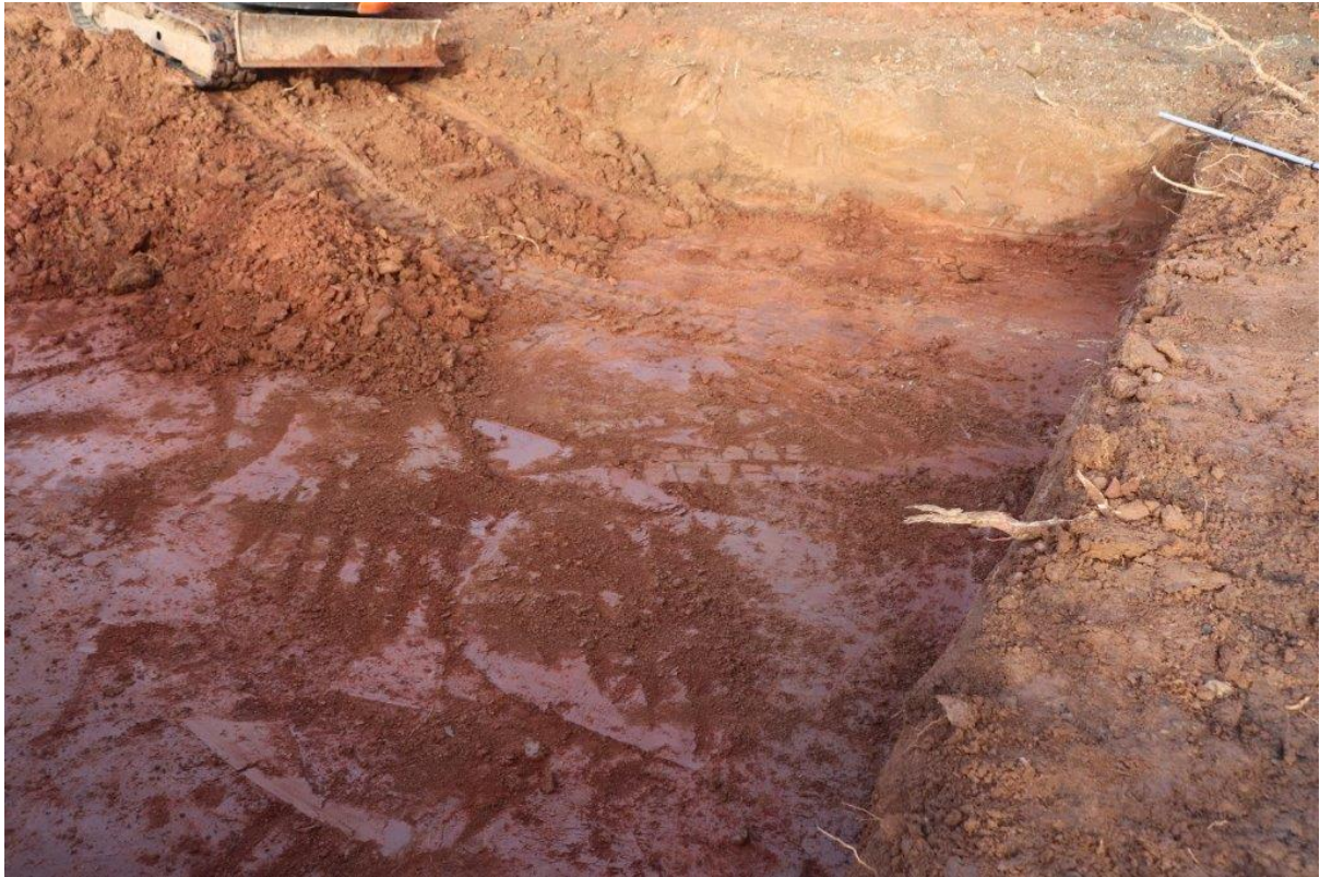
Plate 3: Trench 2, facing north. Showing exposed natural and colluvium (203) in section
