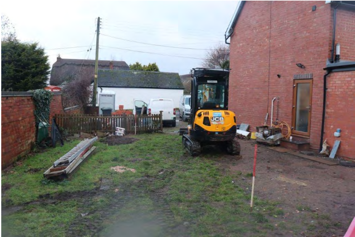
Plate 1: Trench location prior to excavations, view north with 1m scales
