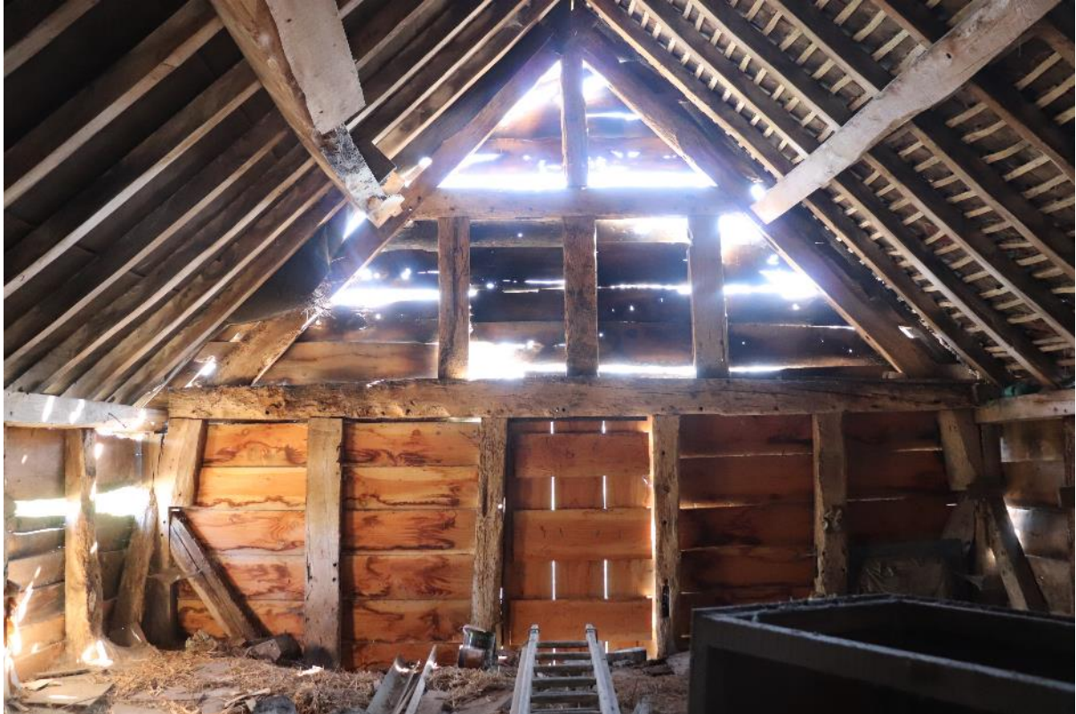
Plate 12 Phase 2 interior inserted first floor, looking east
