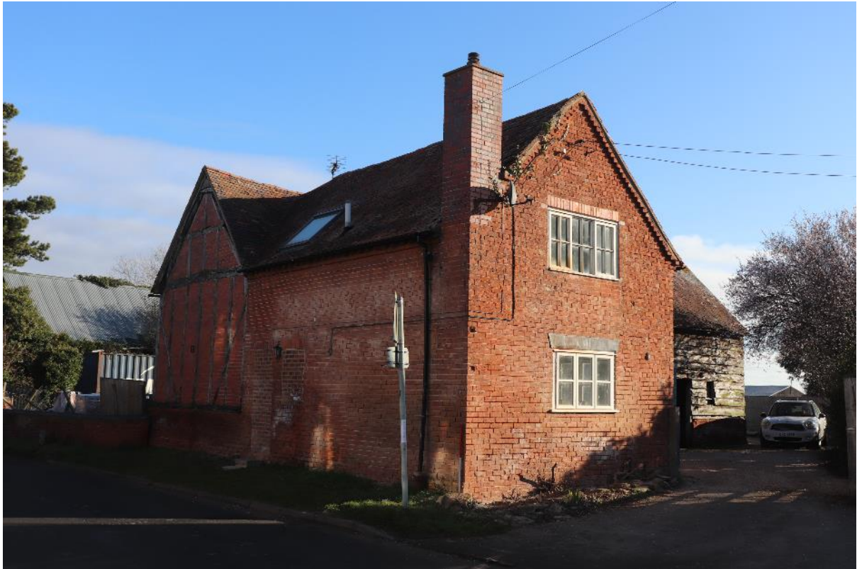
Plate 13 Phase 3 addition, looking north east, scale 1m
