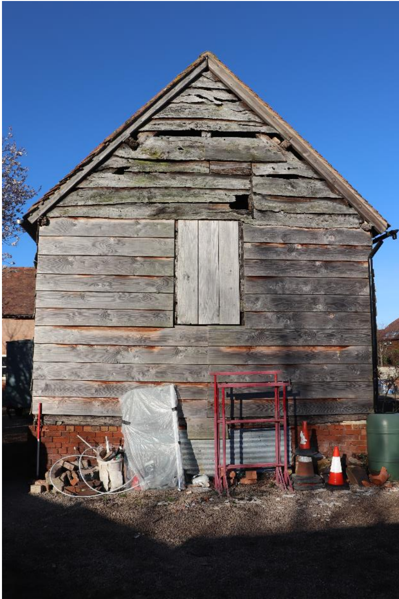
Plate 10 Phase 2 gable end, looking west, scale 1m
