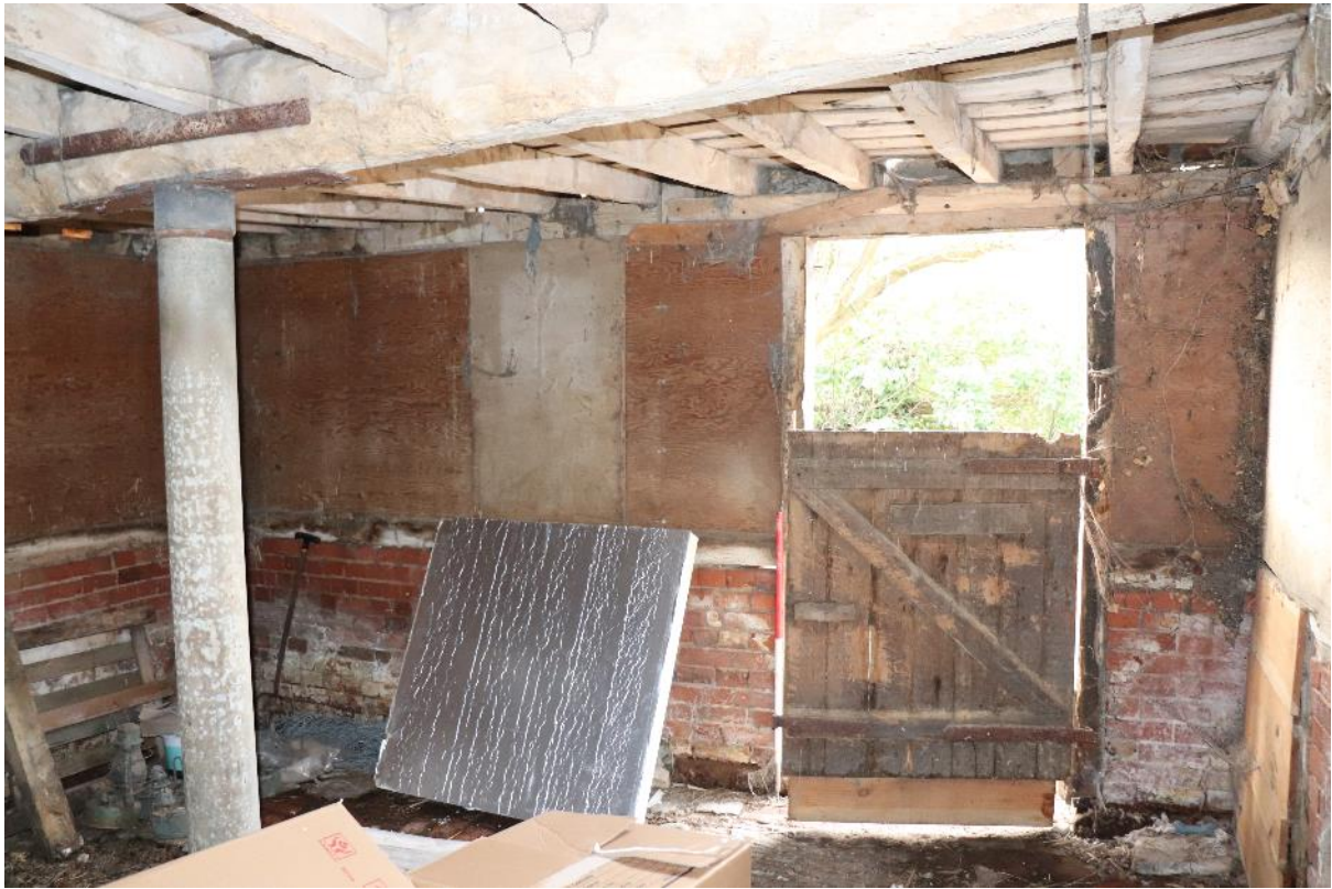
Plate 11 Phase 2 interior ground floor, looking south east, scale 1m
