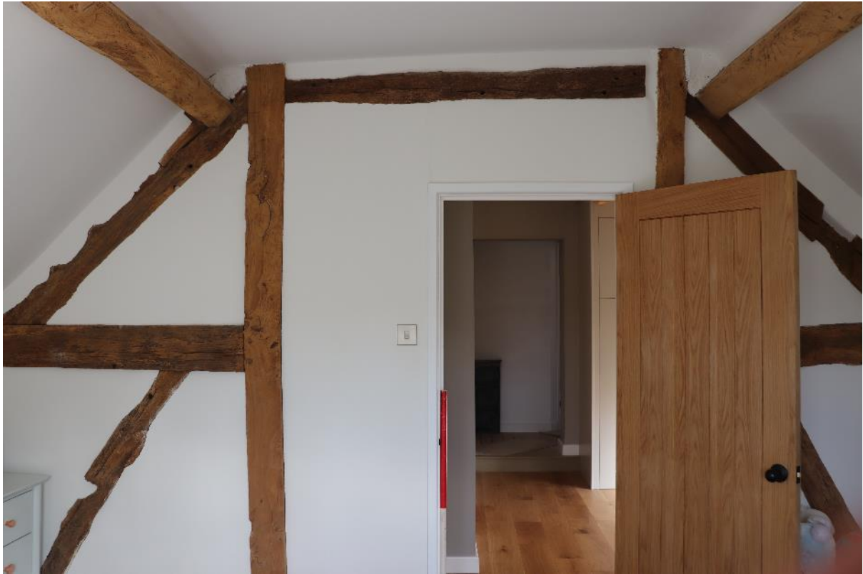
Plate 15 Phase 3 addition first floor roof truss, looking north, scale 1m
