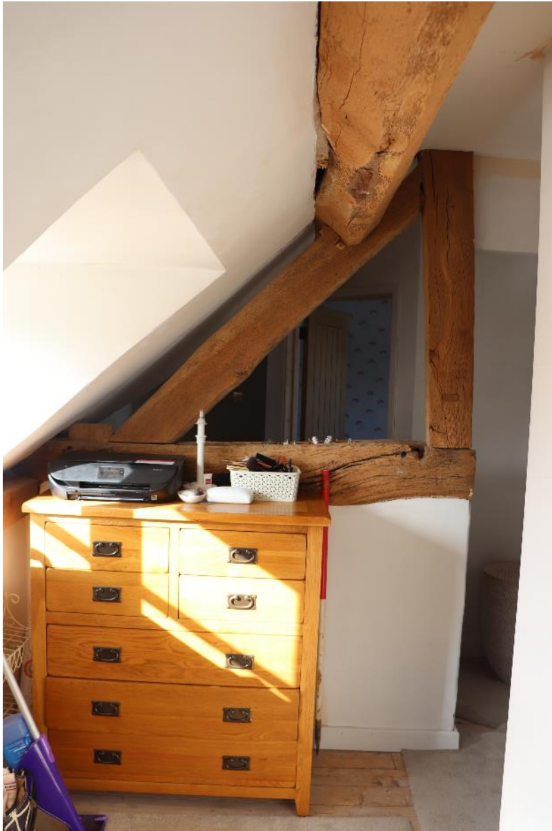
Plate 8 Phase 1 internal cross frame truss, looking west, scale 1m
