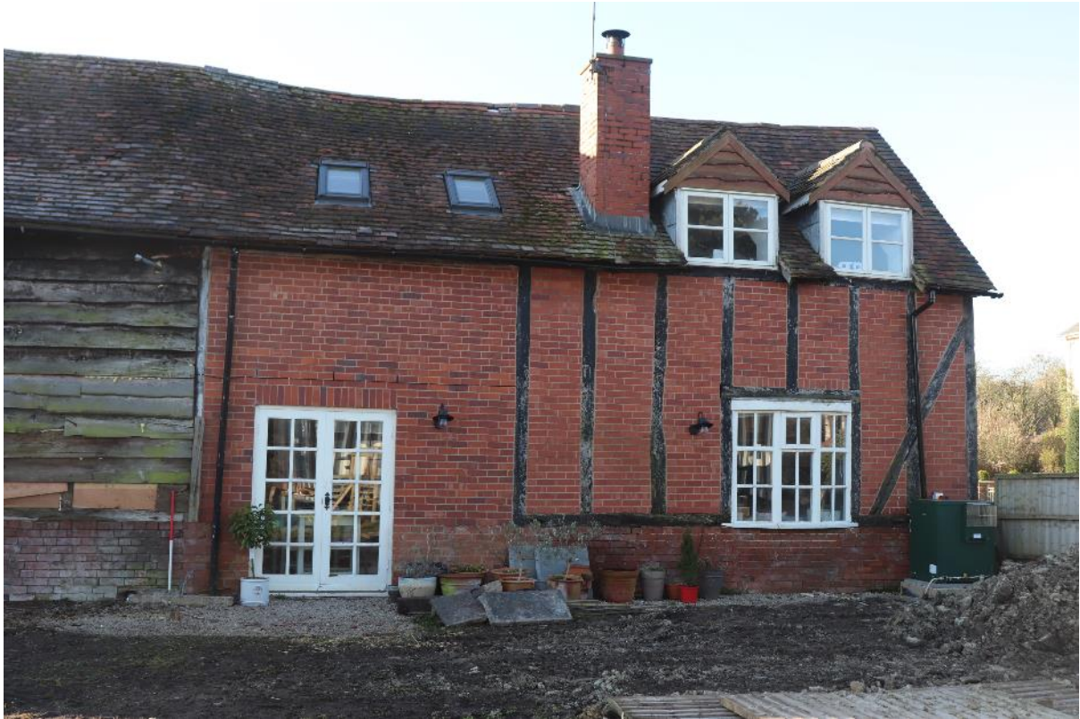
Plate 7 Phase 1 walling, looking south, scale 1m
