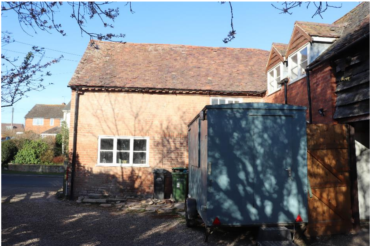
Plate 14 Phase 3 addition, looking west, scale 1m
