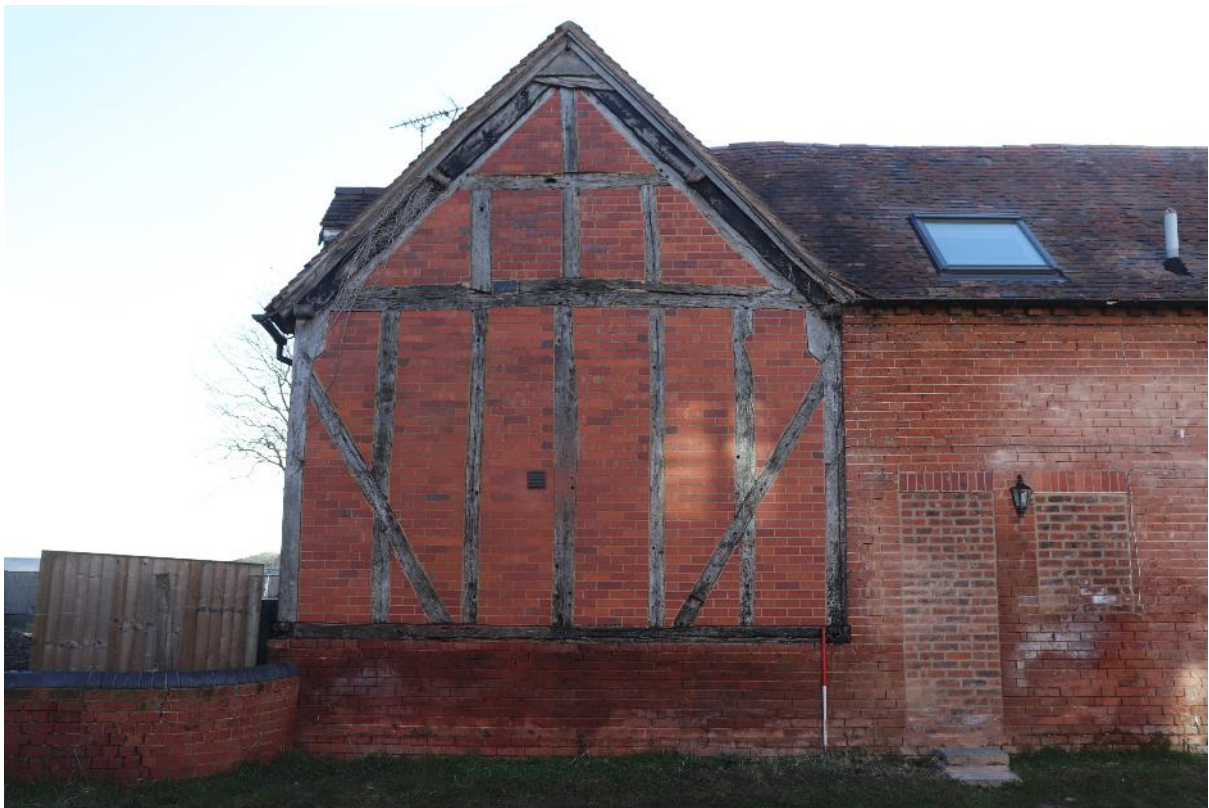
Plate 4 Phase 1 gable end, looking east, scale 1m
