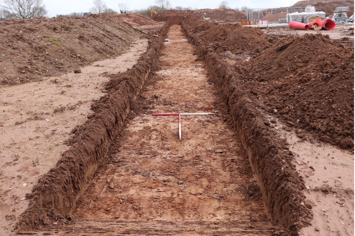
Plate 1: Tr 1, view east, 2x1m scales
