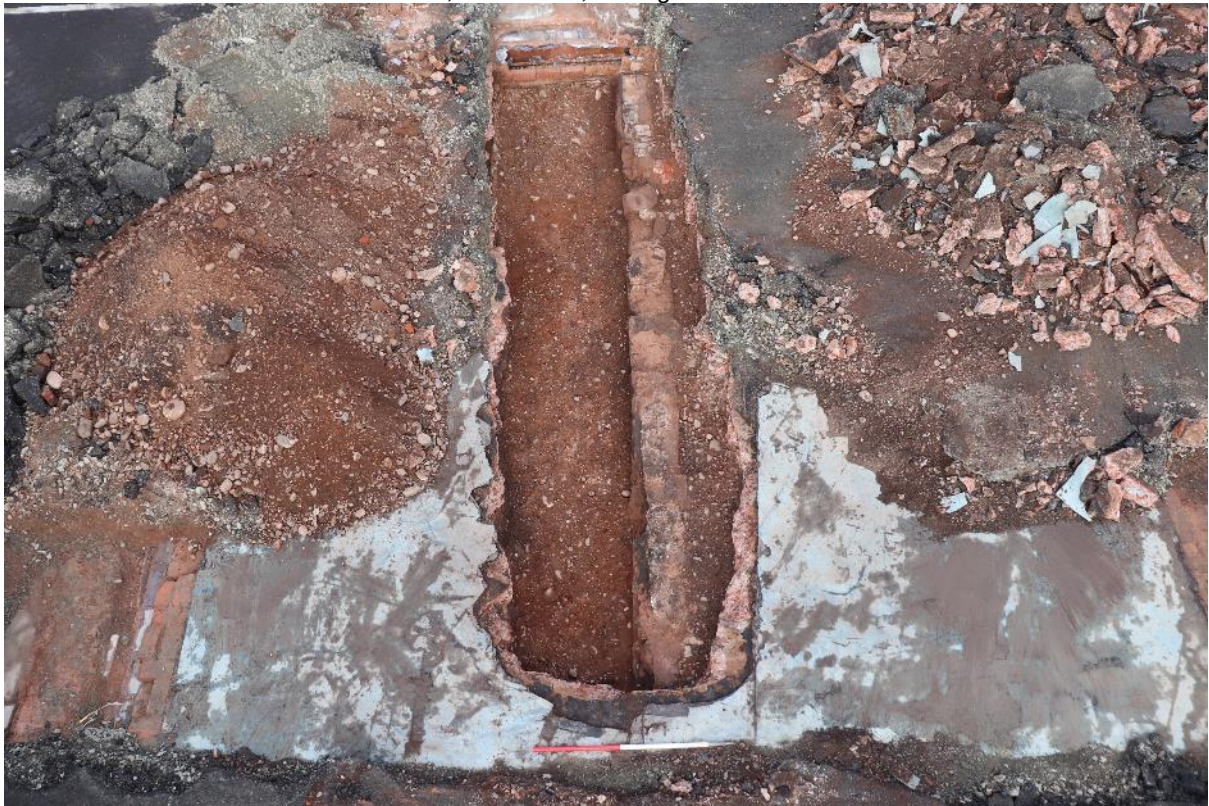
Plate 2: Tr 1 with wall foundation 109 exposed, scale 1m, looking north-west
