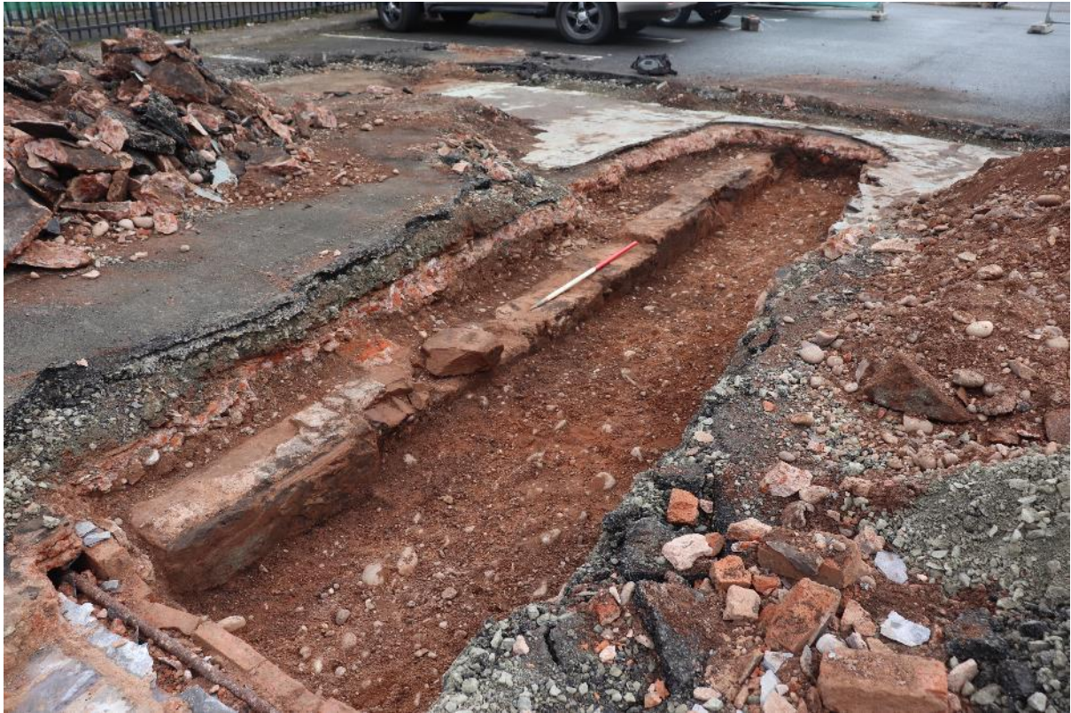
Plate 3: Tr 1 with wall foundation 109 exposed, scale 1m, looking north-east
