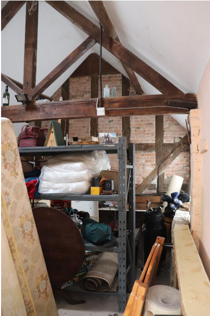
Plate 4 The 19 th century linking structure interior, looking south-west
