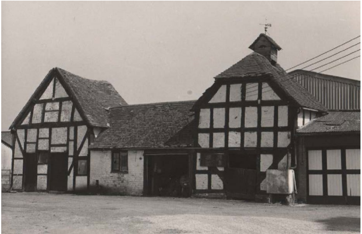
Plate 1 The building, linking structure and dovecote as photographed in 1978, looking south-east
