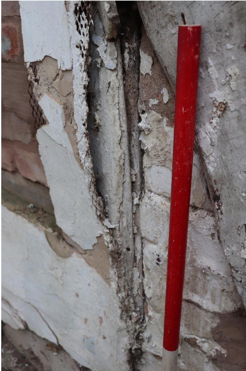
Plate 8 Split lathe and lime washed interior wall covering below 20 th century coverings, looking north-west, 0.50m of a 1m scale
