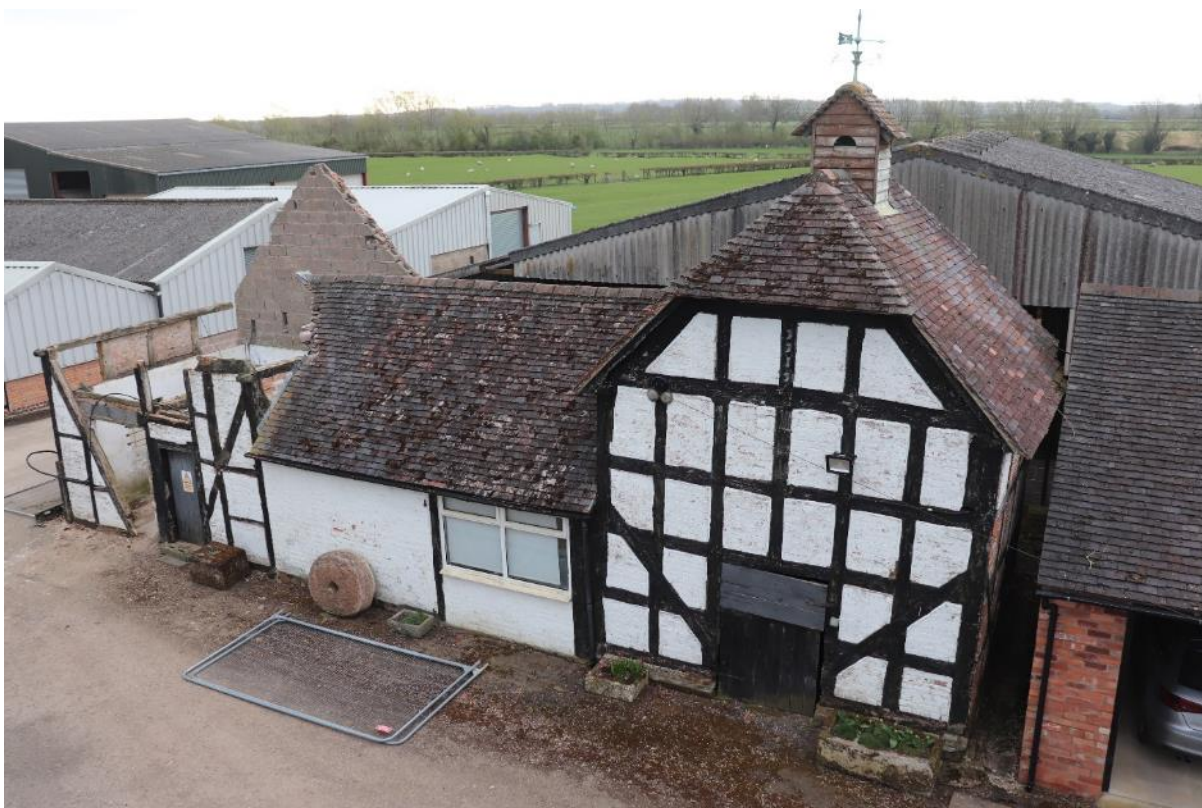
Plate 2 The building, linking structure and dovecote, looking south-east
