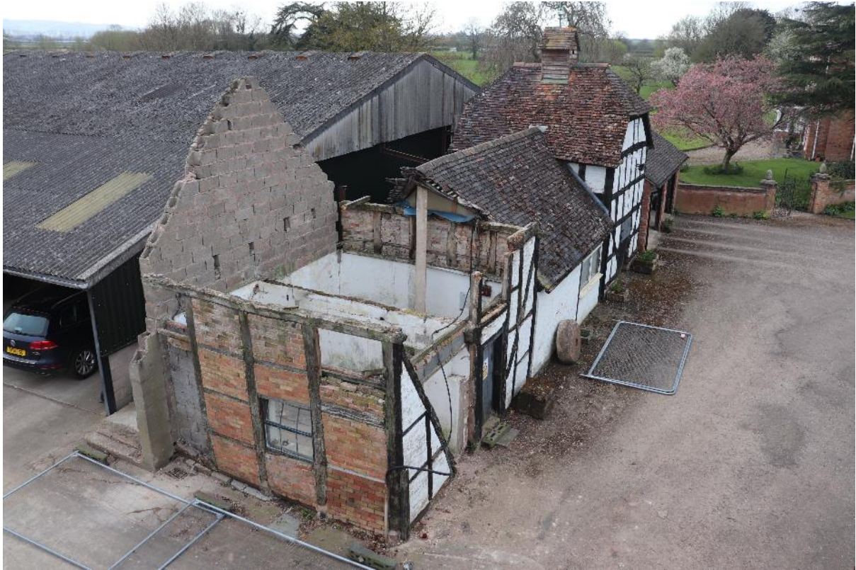
Plate 3 The building, linking structure and dovecote, looking south-west
