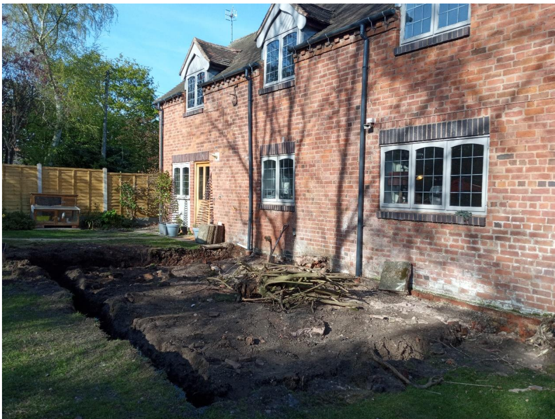
Plate 6: Completed watching brief area
