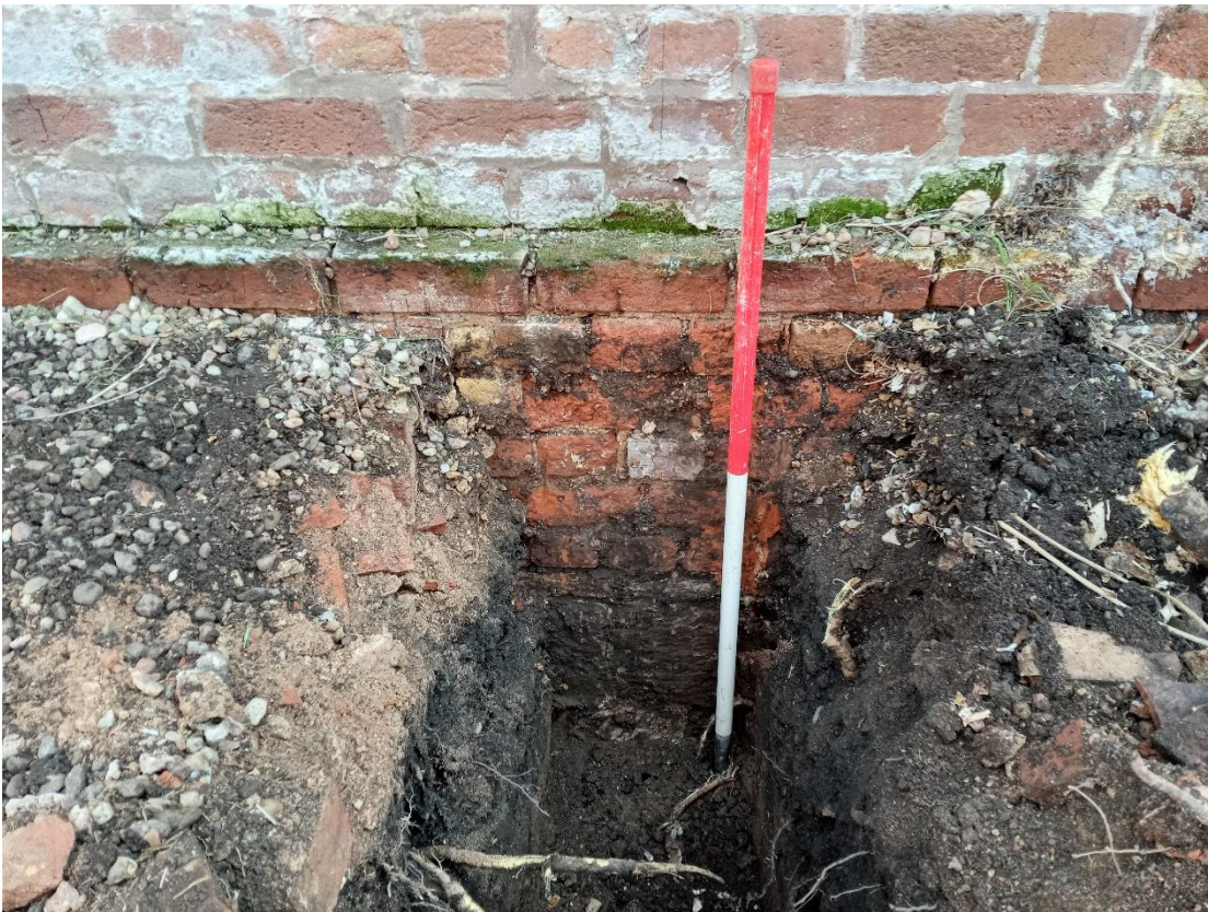
Plate 2: Detail of Oak house foundations
