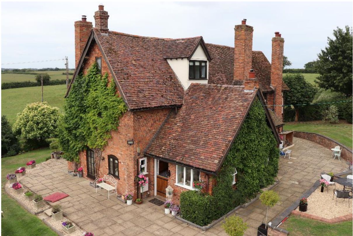
Plate 4 The house, looking south-west, scale 1m
