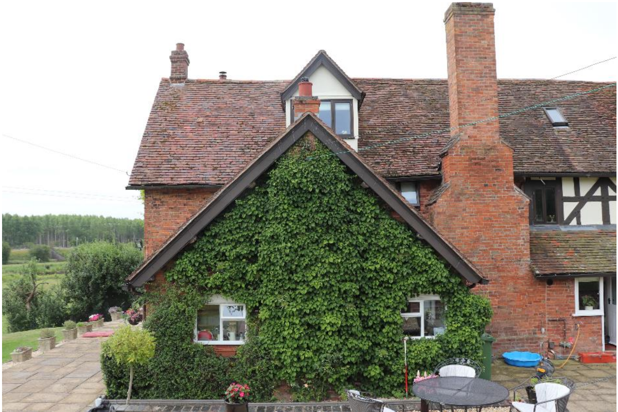
Plate 7 The rear extension exterior, looking south, scale 1m
