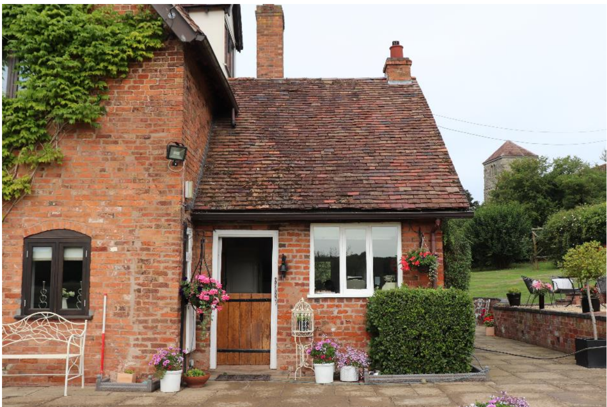
Plate 6 The rear extension exterior, looking west, scale 1m
