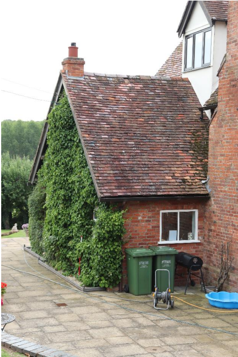
Plate 8 The rear extension exterior, looking south-east, scale 1m
