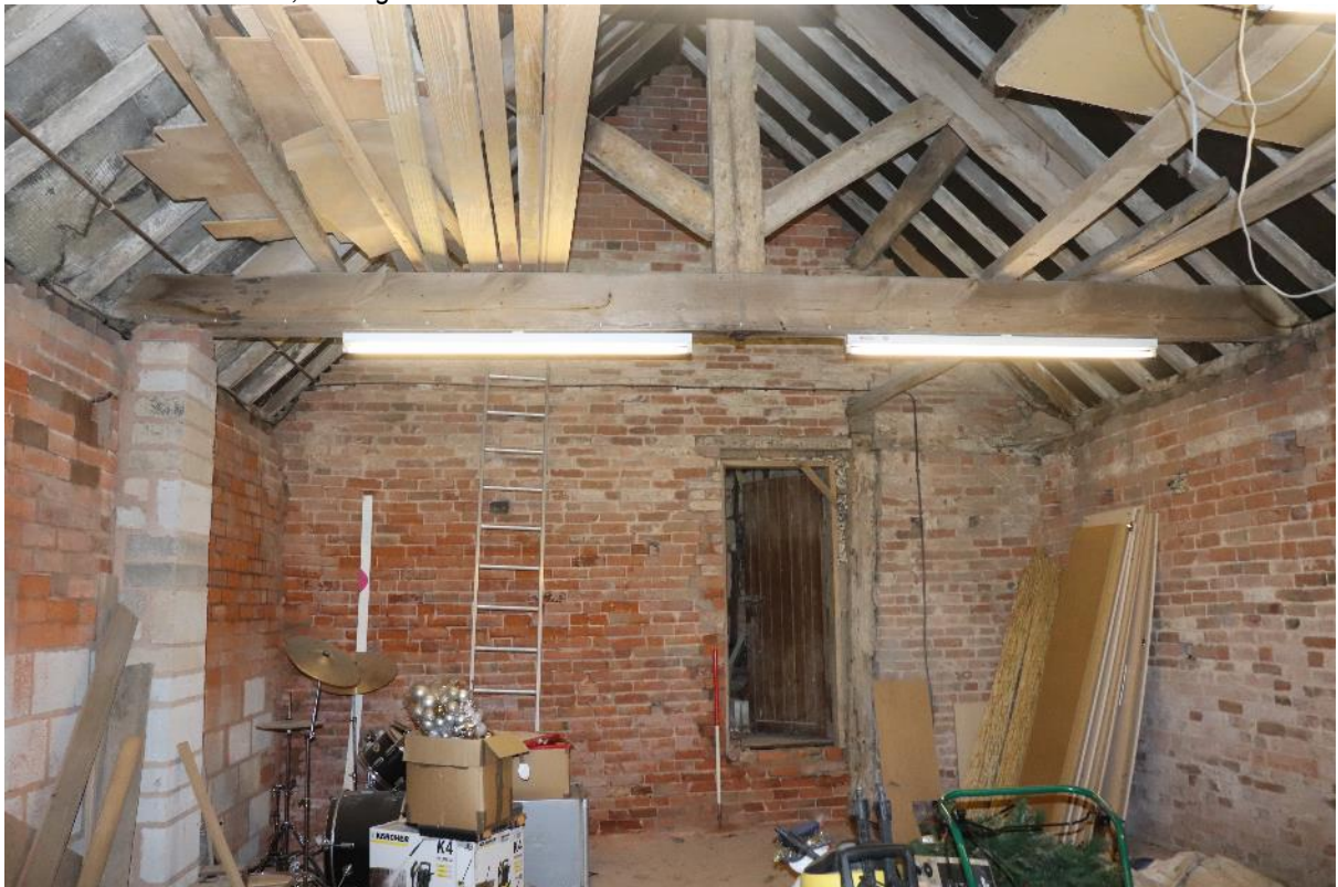
Plate 10 Phase 3 addition, looking north west, scale 1m
