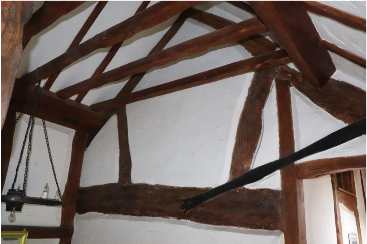
Plate 5 Phase 1 truss 3, looking north
