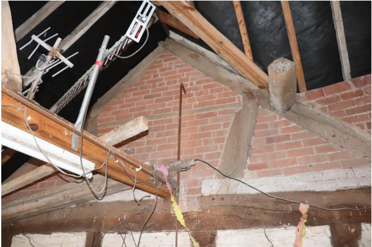
Plate 7 Phase 1 truss 1, looking north
