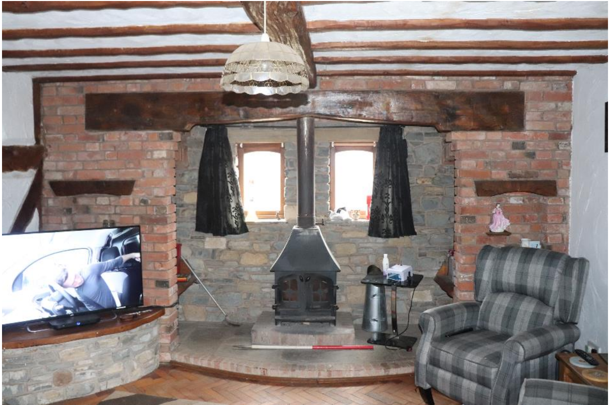
Plate 29 Phase 5 house conversion, looking north west, scale 1m
