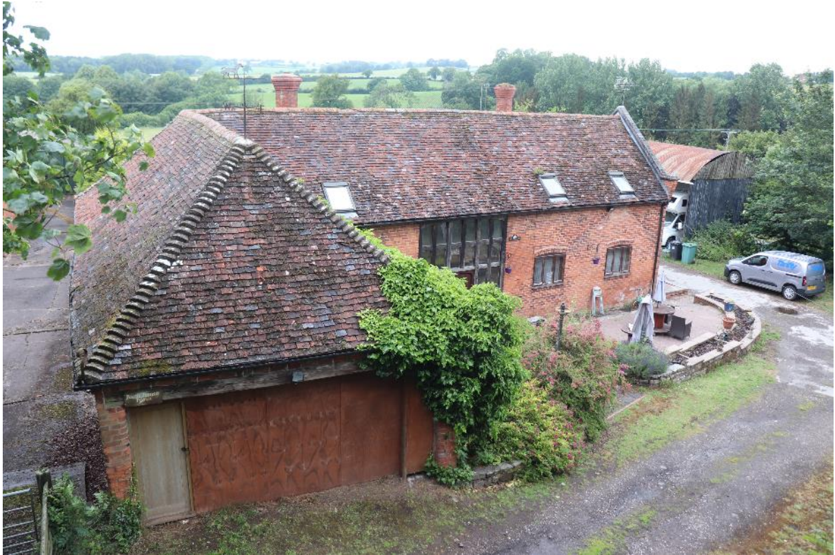
Plate 9 Phase 3 addition, looking west
