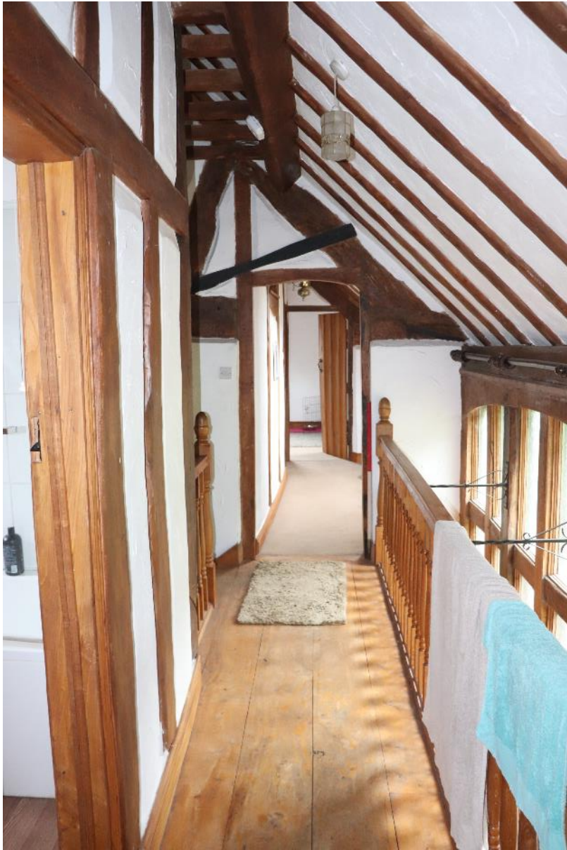
Plate 28 Phase 5 house conversion, looking north east, scale 1m
