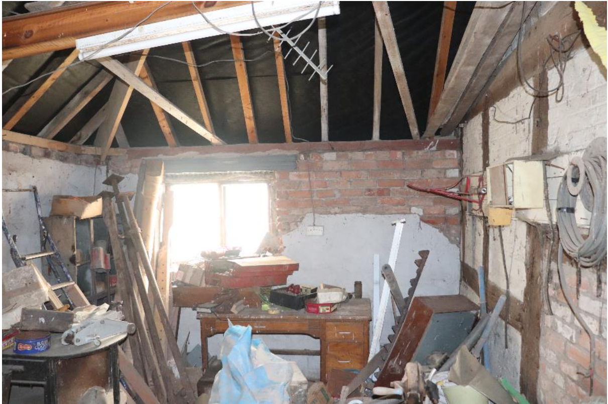
Plate 11 Phase 3 addition, looking north west, scale 1m
