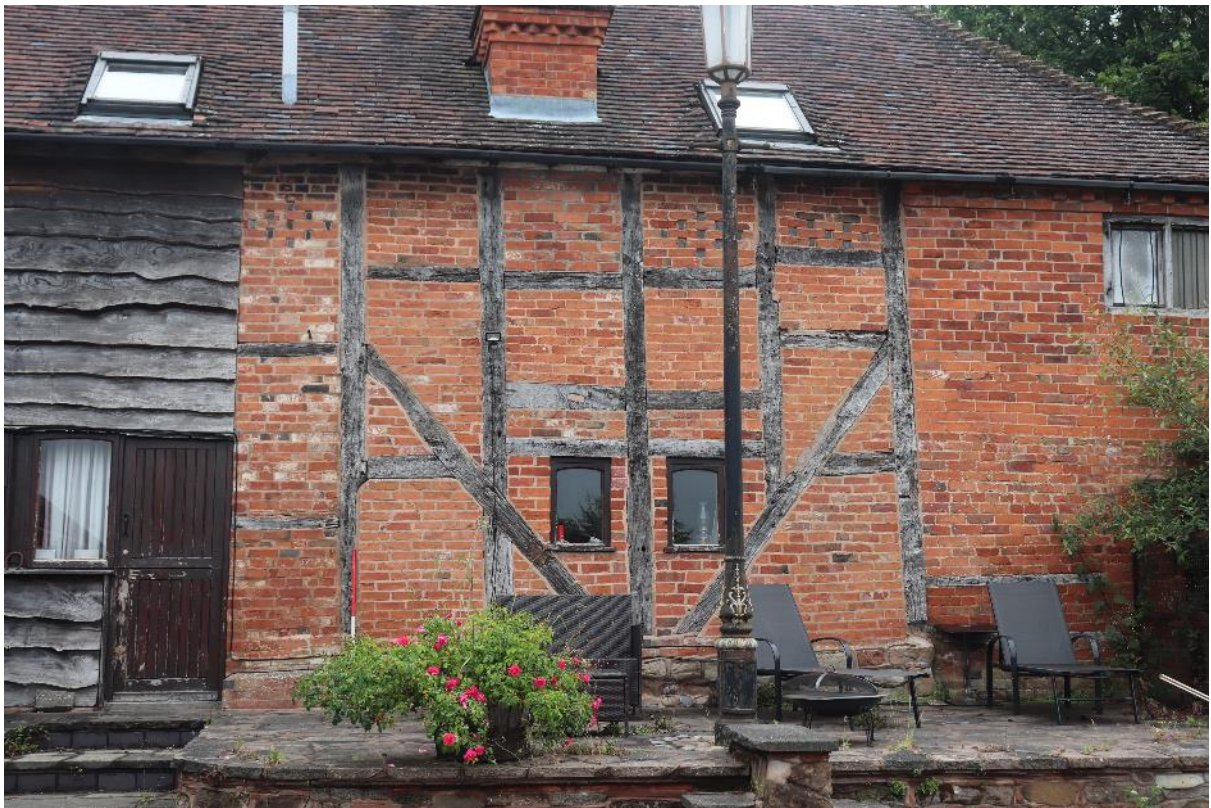
Plate 8 Phase 1 wall framing, looking south east, scale 1m
