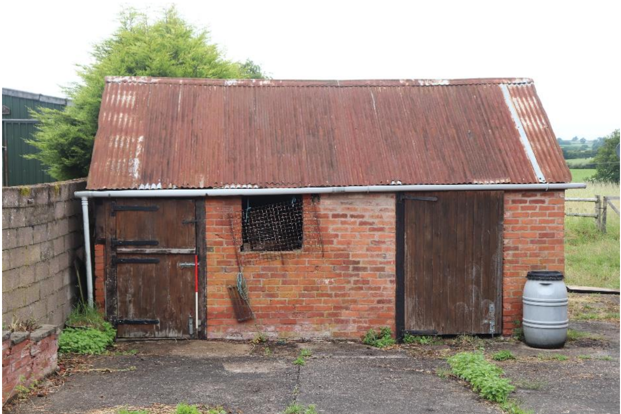
Plate 20 Phase 4 cow shed, looking north west, scale 1m
