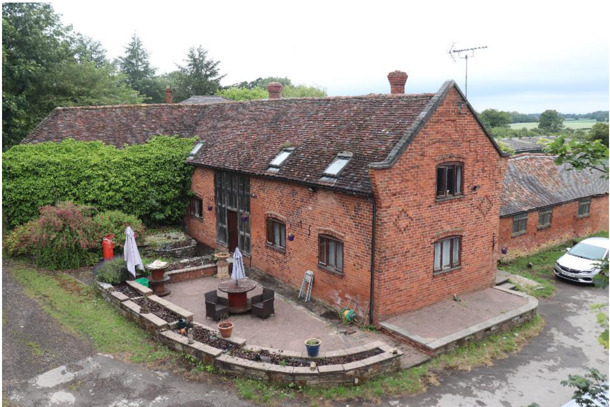
Plate 14 Phase 3 threshing barn, looking west
