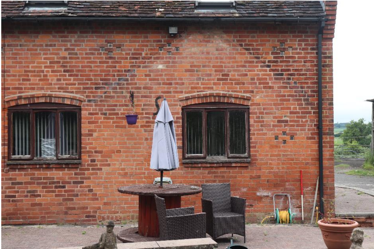
Plate 15 Phase 3 addition, looking north west, scale 1m
