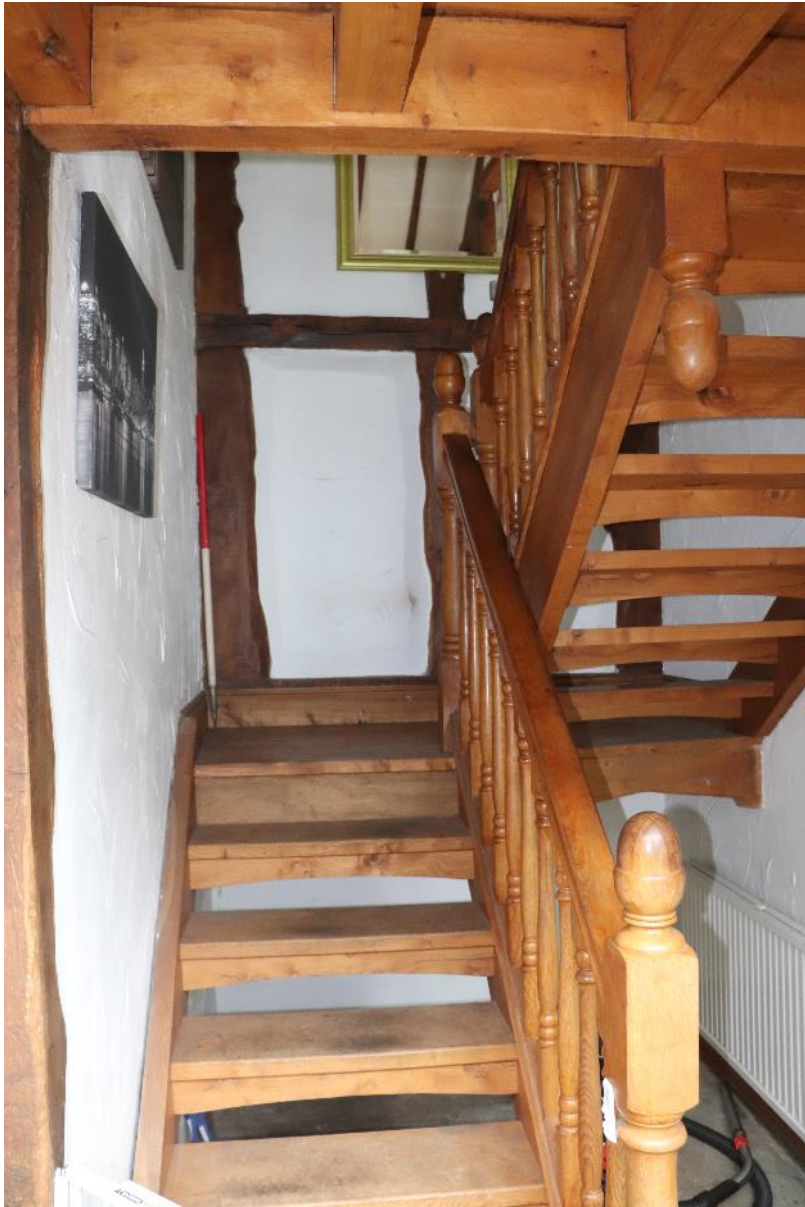
Plate 31 Phase 5 house conversion, looking north west, scale 1m
