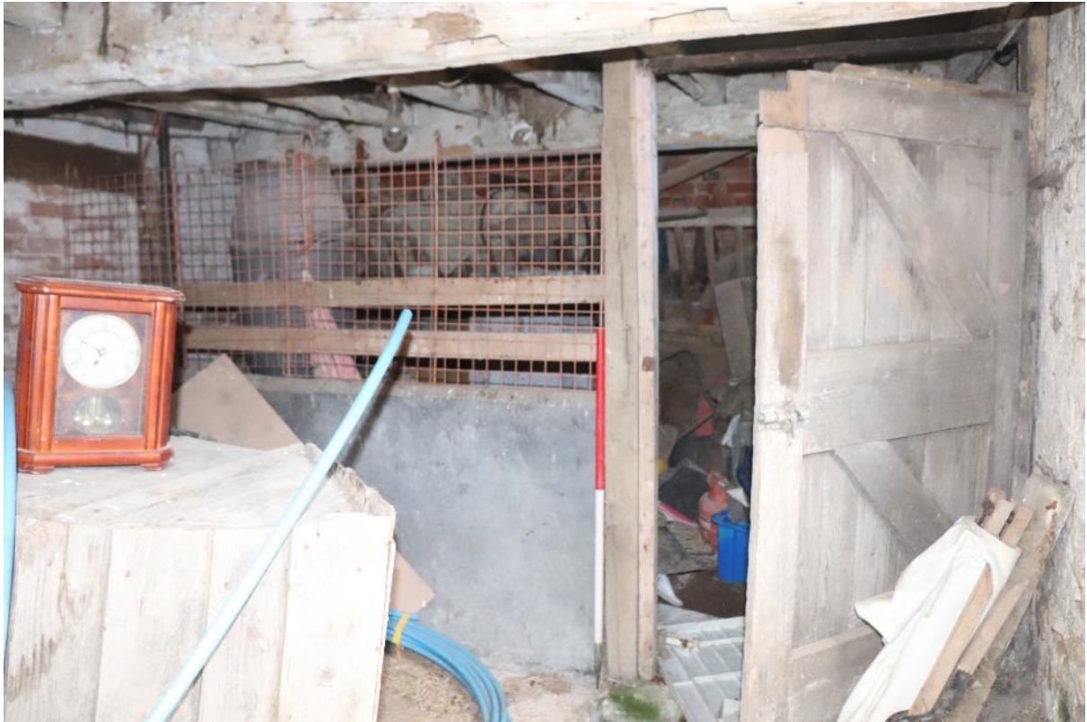
Plate 13 Phase 3 addition, looking north east, scale 1m
