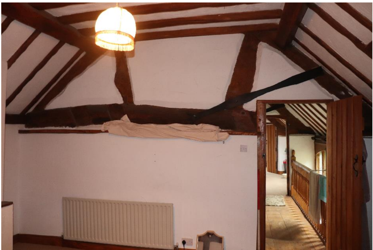
Plate 6 Phase 1 truss 2, looking north, scale 1m
