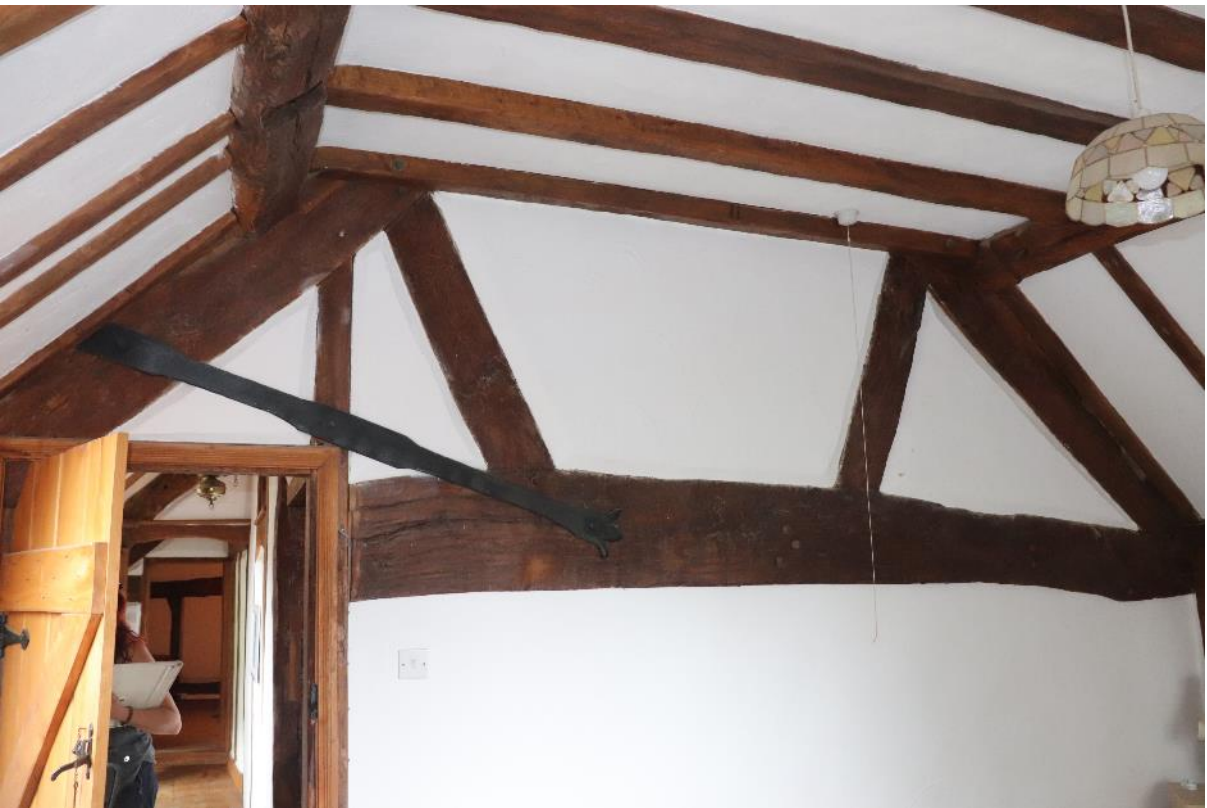
Plate 4 Phase 1 possible former gable end truss 4, looking south west
