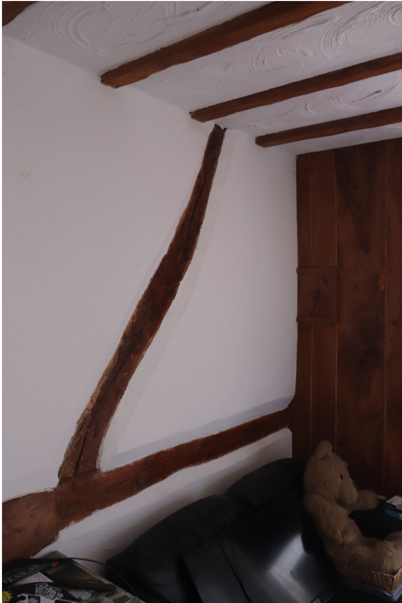
Plate 33 Phase 1 lower part of cross frame 2, looking west
