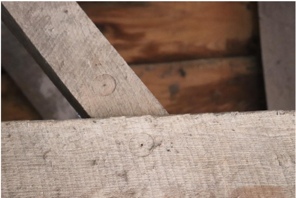
Plate 24 Phase 4 cow shed, looking north east
