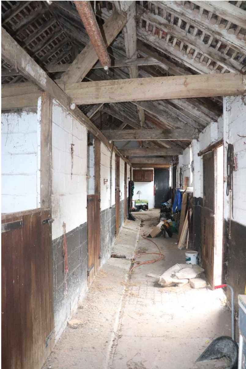
Plate 18 Phase 3 cow shed, looking south east, 1m scale
