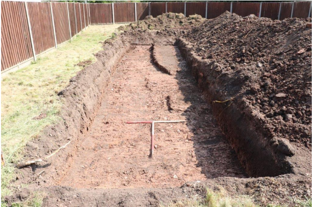
Plate 1: North west side of Trench 1, 2 x 1m scales
