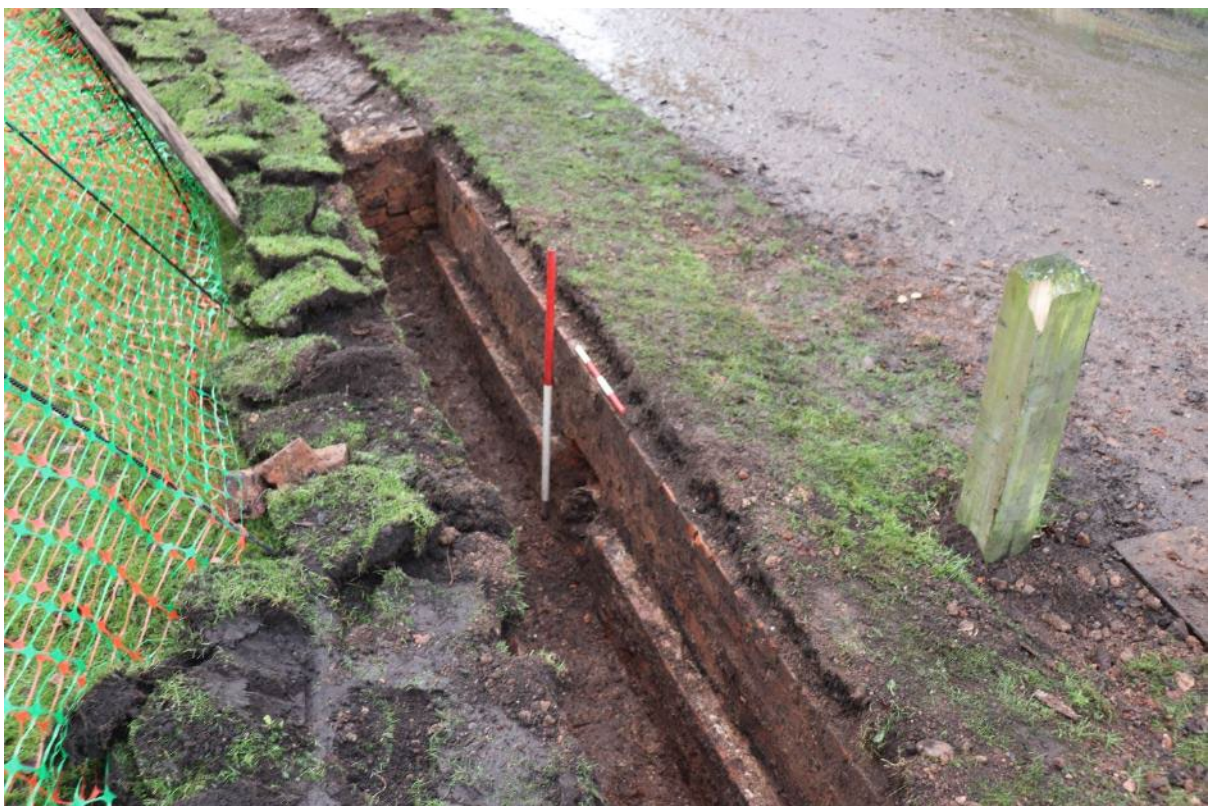
Plate 14: External wall and footing (204) of former stable block, cut by modern drain, with internal wall (206), brick and cobble surface (205) in background, view south-west; 1m scale
