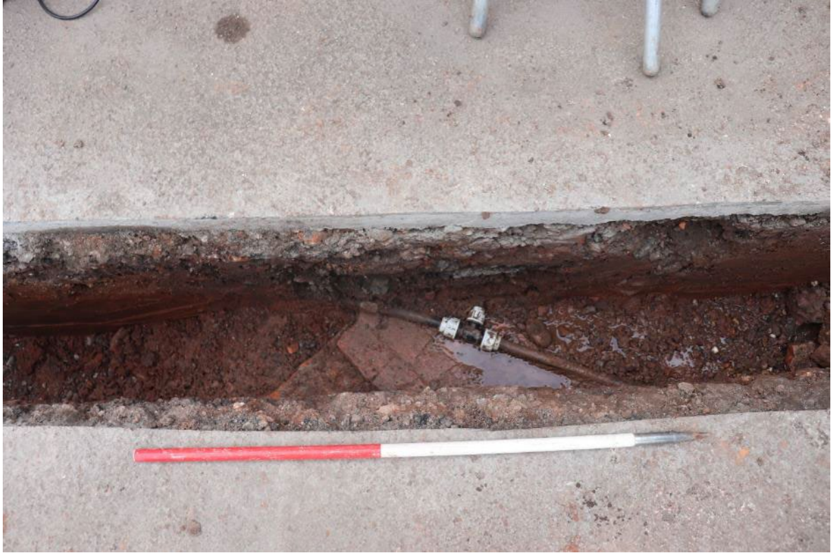
Plate 21: Trench 4 across Service Yard, wall (412) overlaid by modern water pipe, view south; 1m scale
