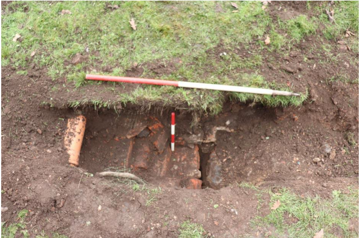
Plate 25: Trench 5, top of brick culvert arch (503), overlain by modern drainage and turf, view south-east; 0.40m and 1m scales
