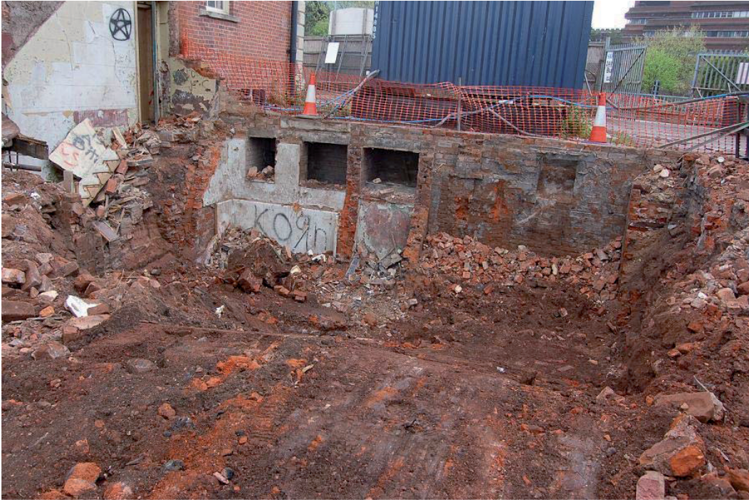
Plate 5, North-West Range, demolition in progress, view east
