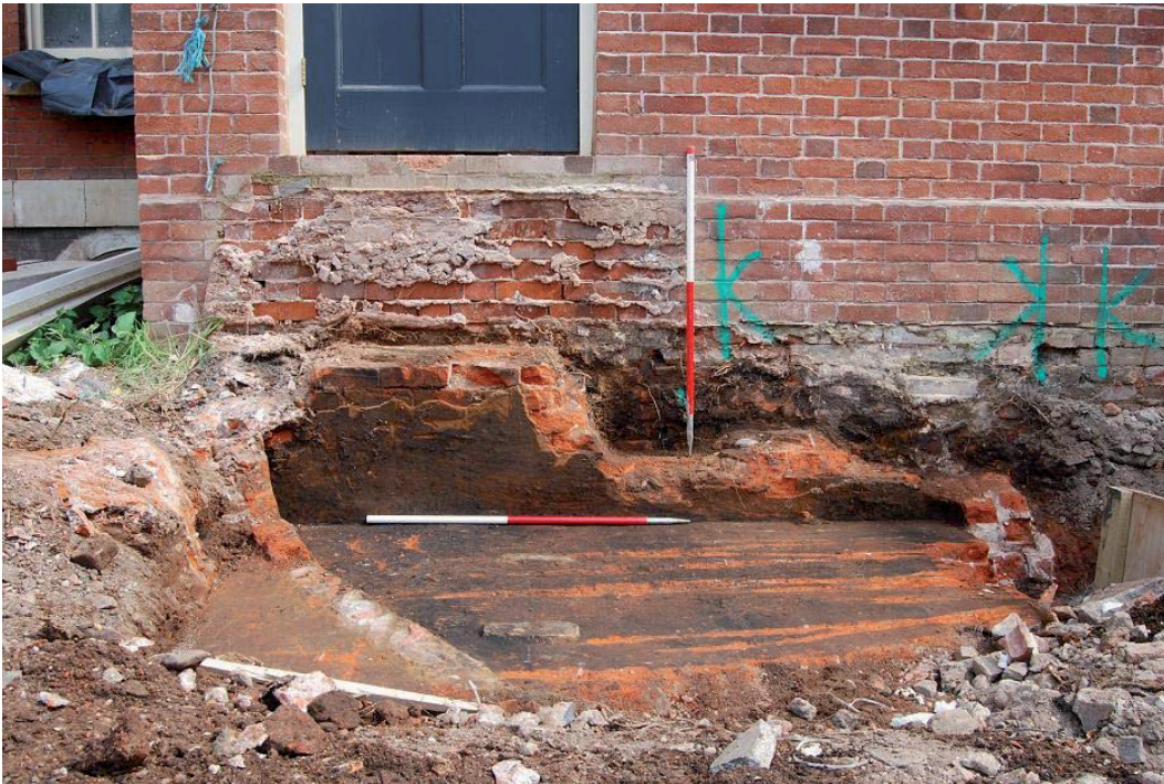
Plate 13, Brick foundation, 114, for staircase, north corner of West Range, view southeast
