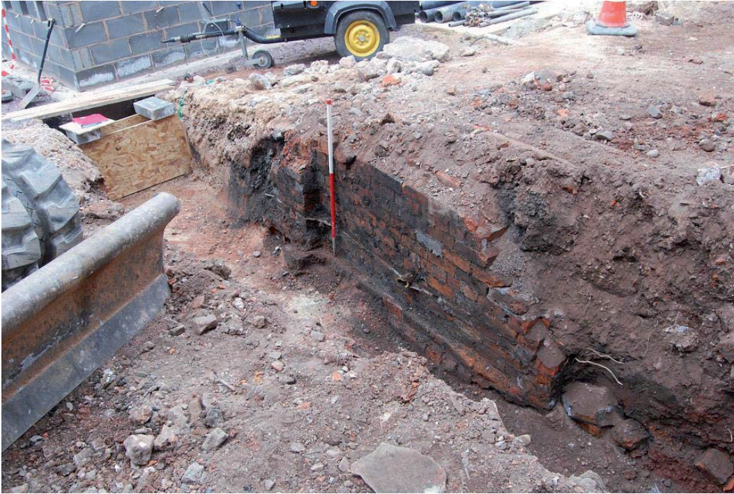
Plate 15, Wall, 115, north of West Range, view north
