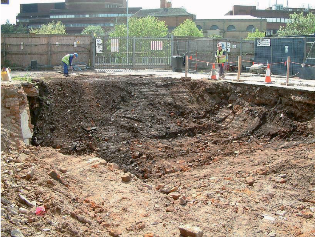
Plate 8, North-West Range, demolition in progress, view south
