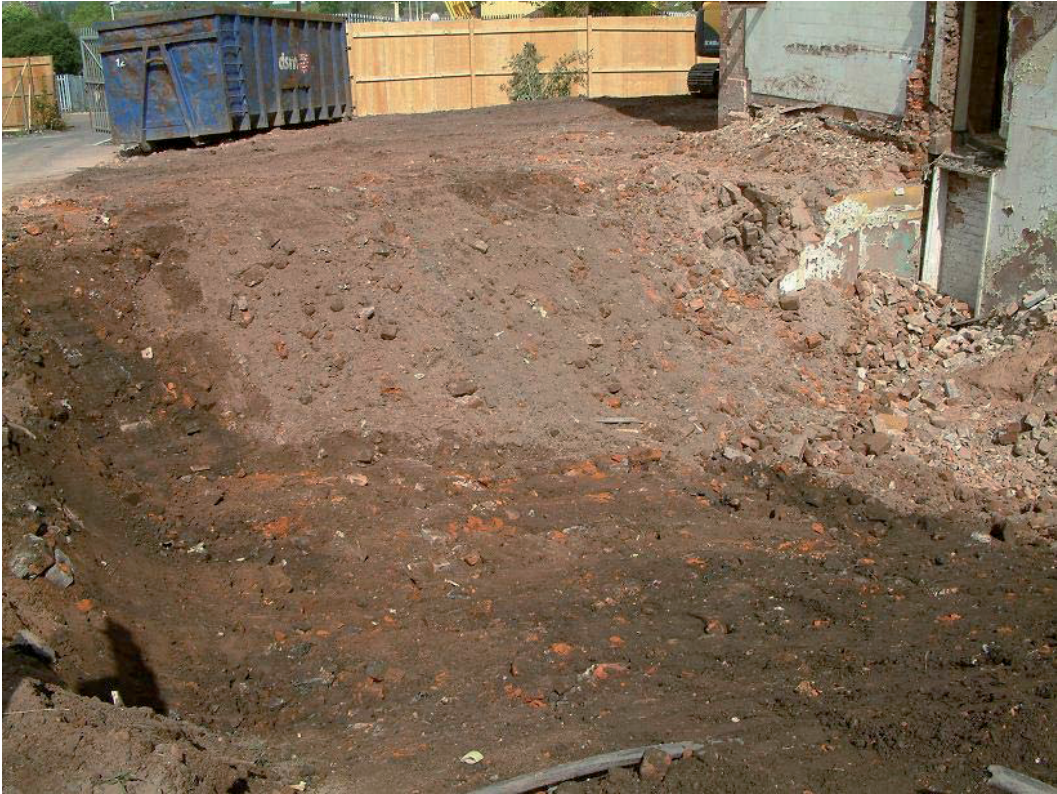
Plate 7, North-West Range, demolition in progress, view north
