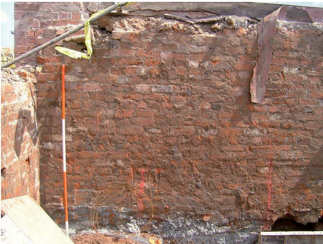
Plate 12, Foundation wall, 112, below southwest wall of West Range, view northeast
