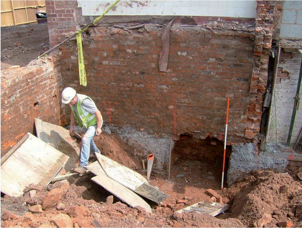
Plate 11, Foundation wall, 112, below southwest wall of West Range, view northeast
