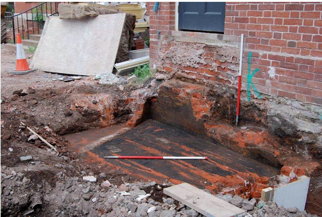
Plate 14, Brick foundation, 114, for staircase, north corner of West Range, view east
