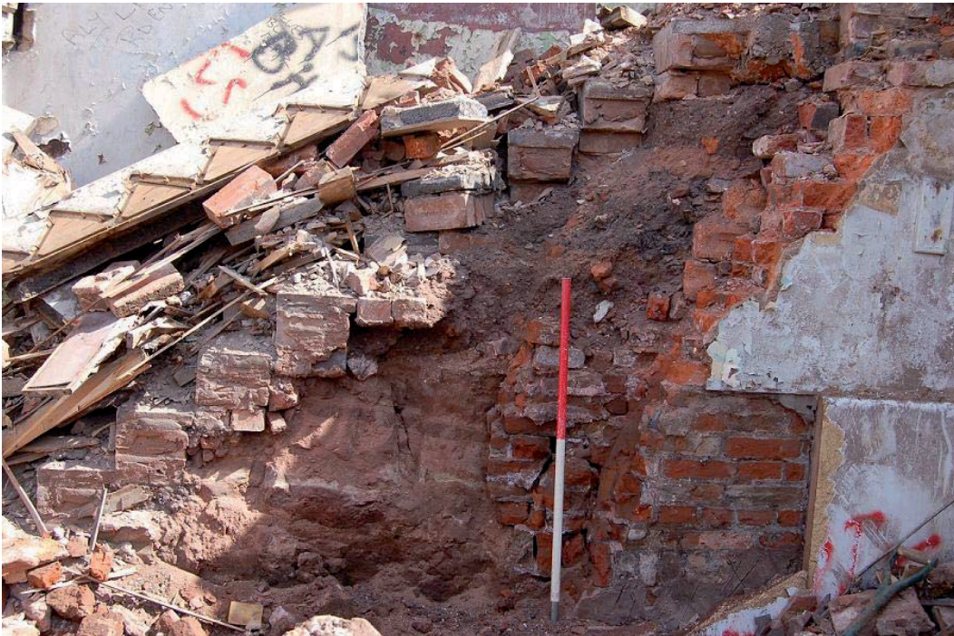
Plate 6, Cellar stairs, 106, and wall, 107, below North-West Range, view northeast
