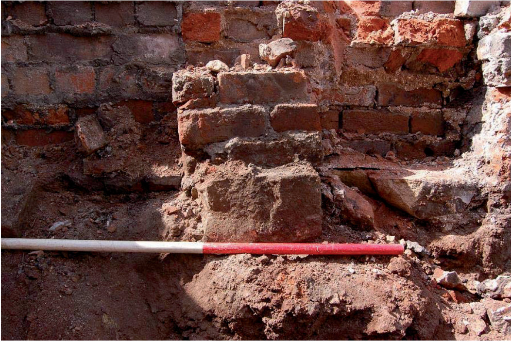
Plate 3, Southwest foundation wall and buttress, 109 and 110, below North-West Range, view southwest
