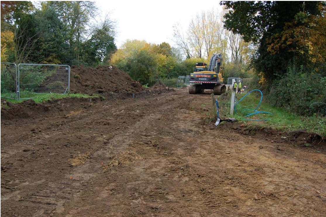
Plate 12, Field 5, general shot of easement strip, view southwest
