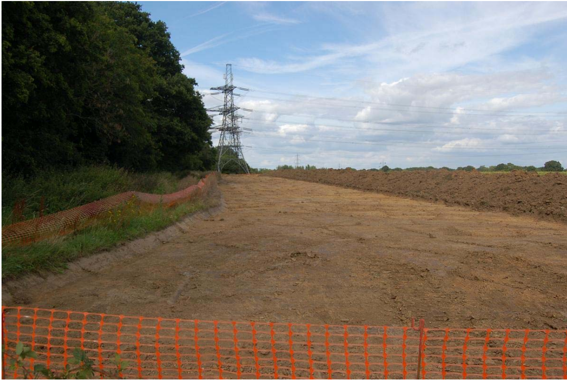
Plate 1, Field 1, general shot of easement strip, view north
