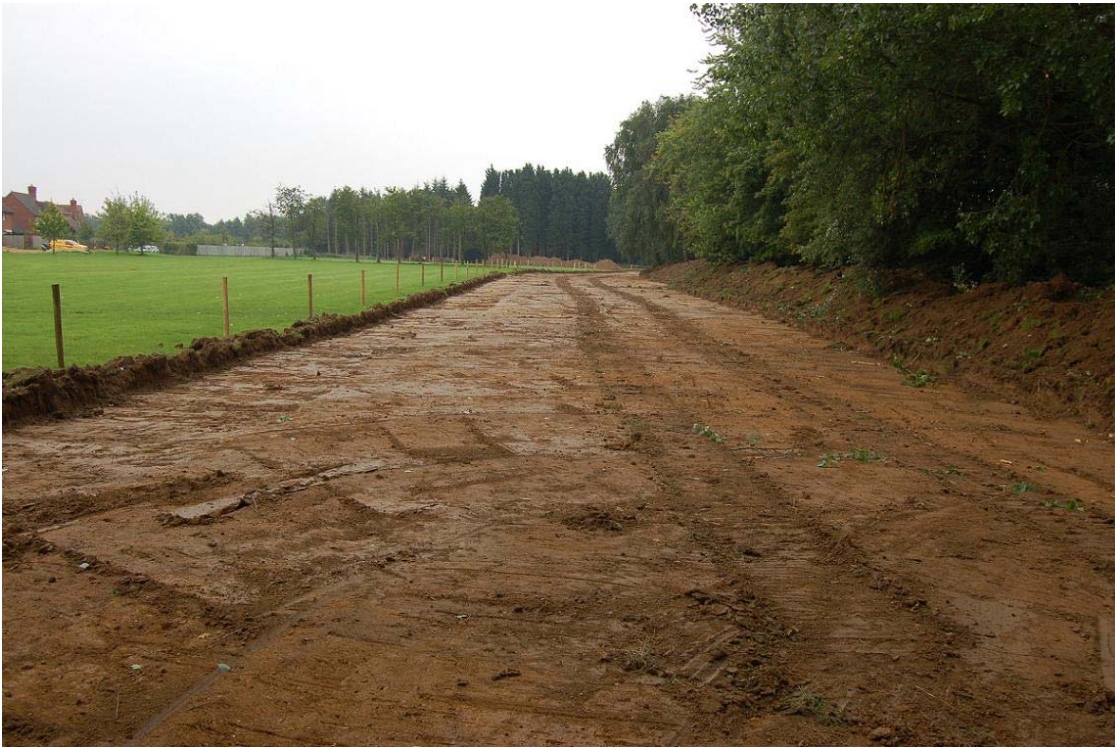
Plate 17, Field 6, general shot of easement strip, view south
