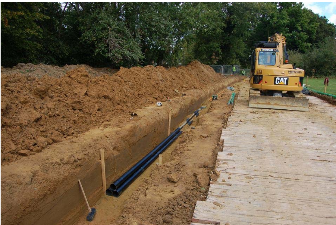
Plate 18, Field 6, general shot of cable trench, view north
