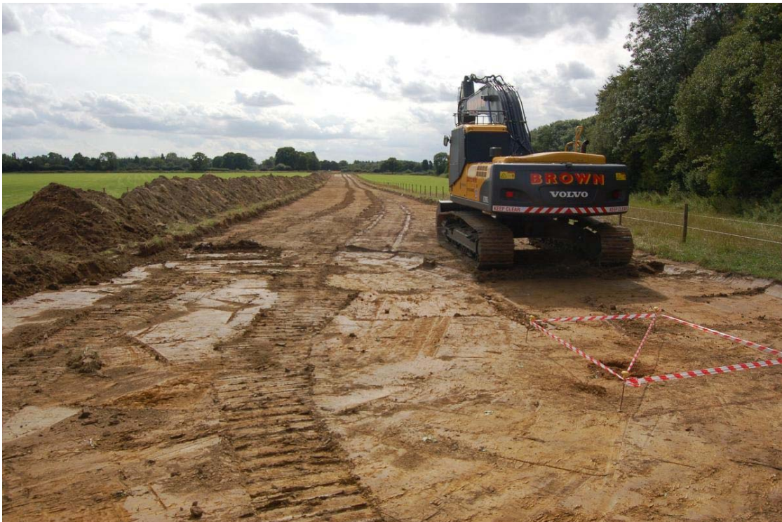
Plate 2, Field 2, general shot of easement strip, view south
