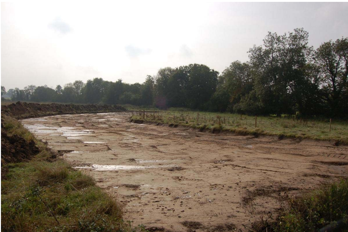
Plate 20, Field 10, general shot of easement strip, view south
