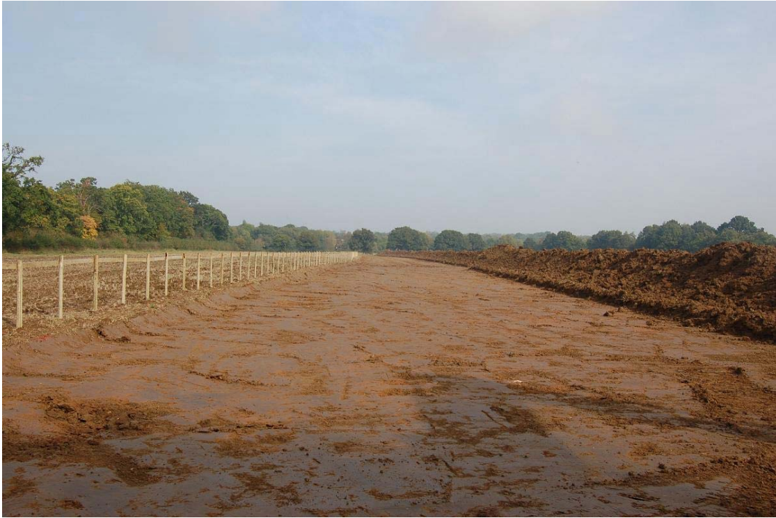
Plate 23, Field 12, general shot of easement strip, view north
