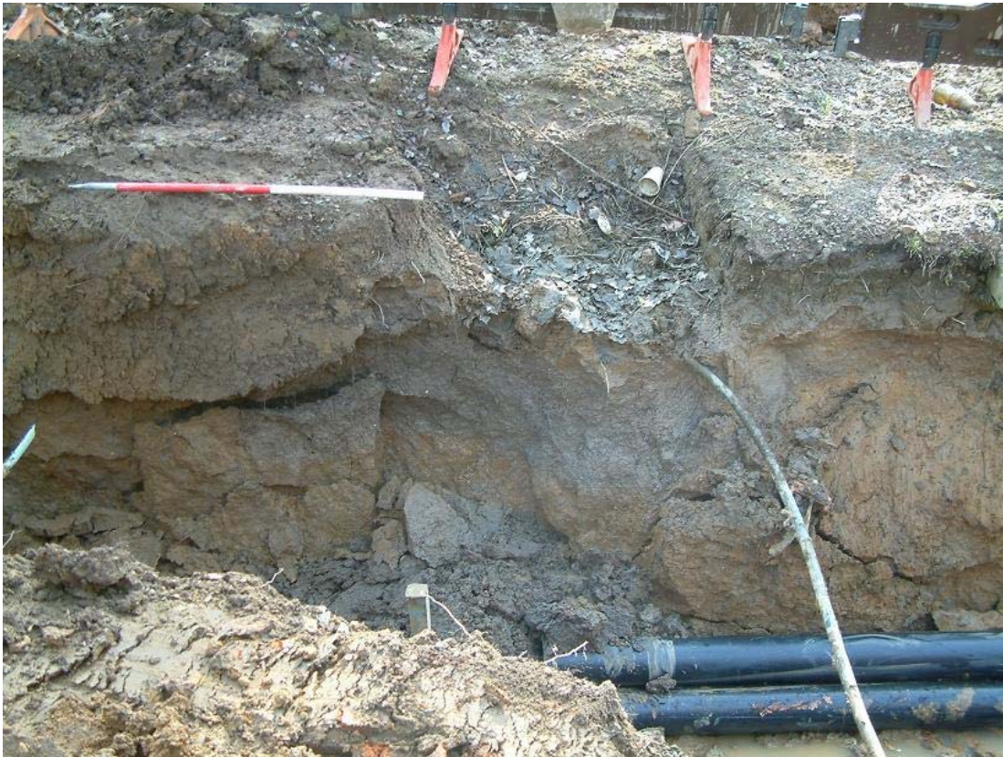
Plate 13, Field 5, ditch 5004 in cable trench, view south
