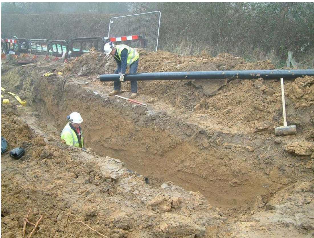
Plate 14, Field 5, cable trench, view north
