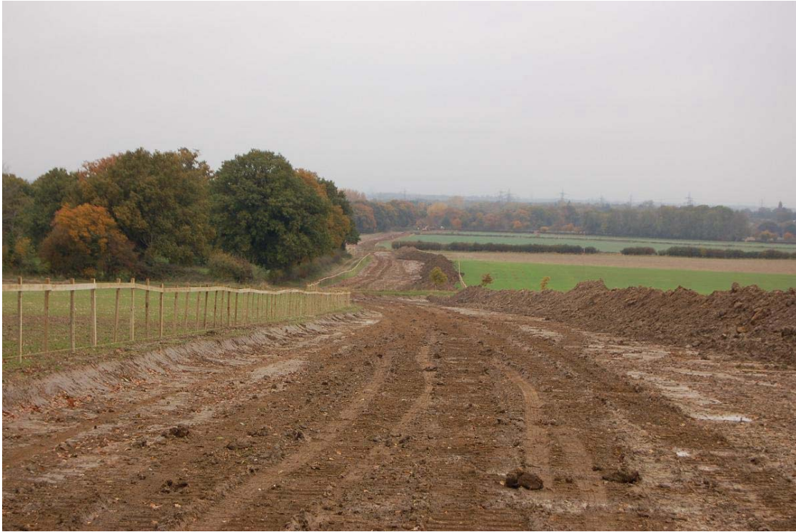
Plate 25, Field 15, general shot of easement strip, view north
