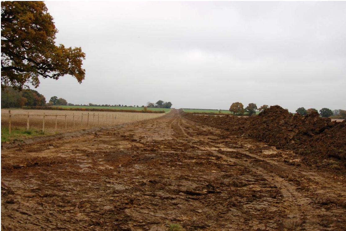
Plate 26, Field 17, general shot of easement strip, view north
