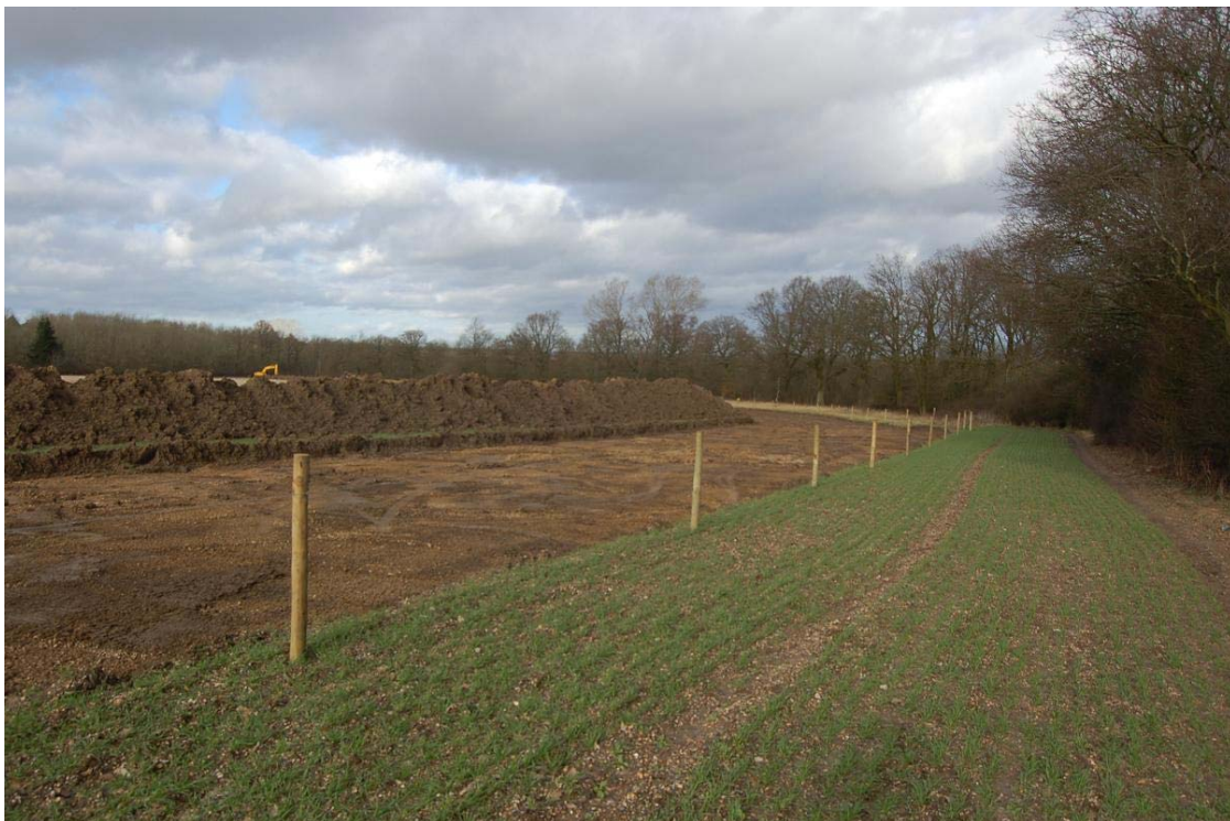
Plate 28, Field 19, general shot of easement strip, view northwest
