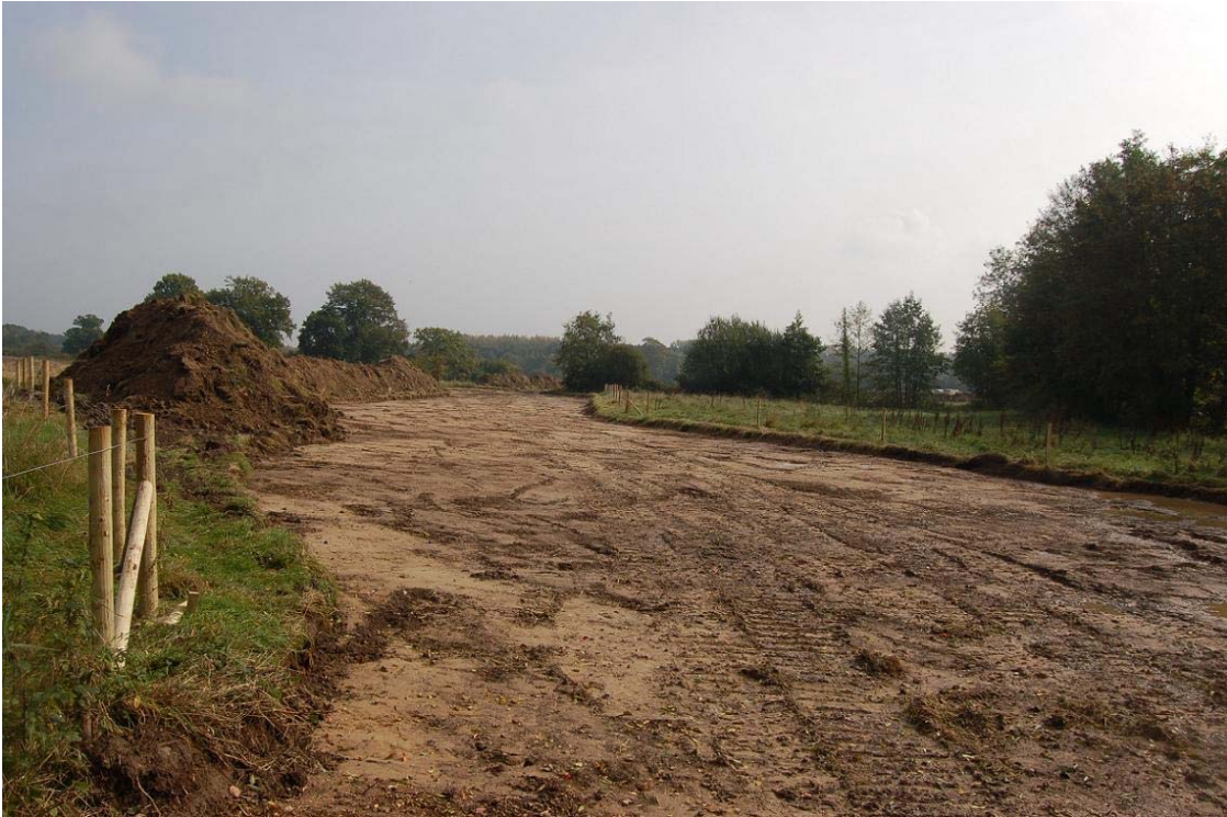
Plate 19, Field 9, general shot of easement strip, view east
