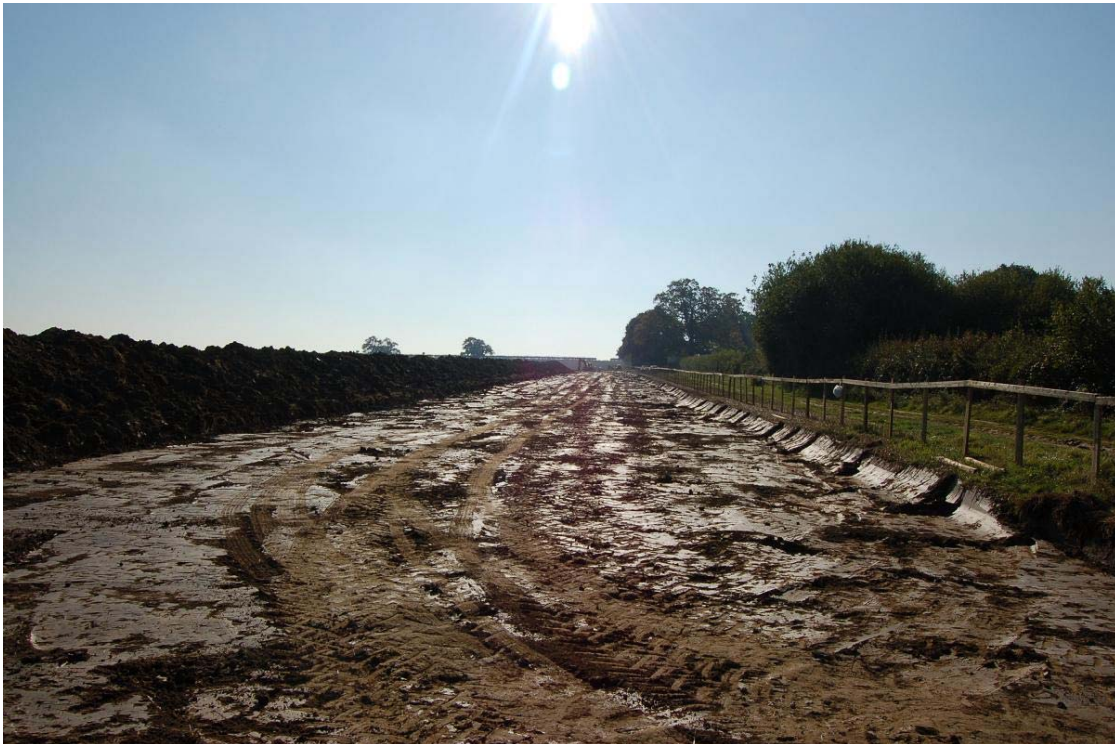
Plate 24, Field 14, general shot of easement strip, view south
