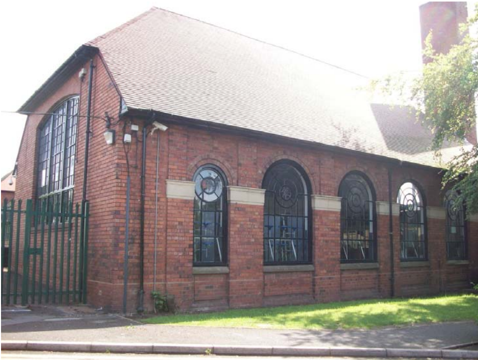
Plate 6, 1931 school building, detail of south-west elevation, view east
