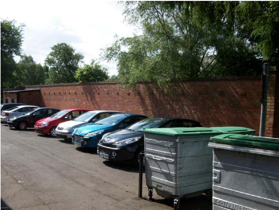
Plate 8, Former cycle shed and brick boundary wall with School Cottage, view south
