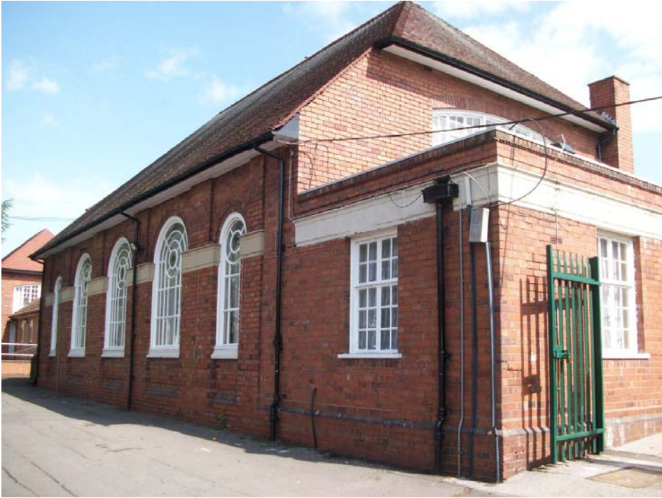
Plate 5, 1930 school building, detail of south-west elevation, view north
