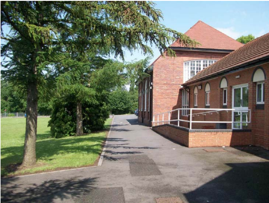
Plate 14, General view north-west along front of school buildings
