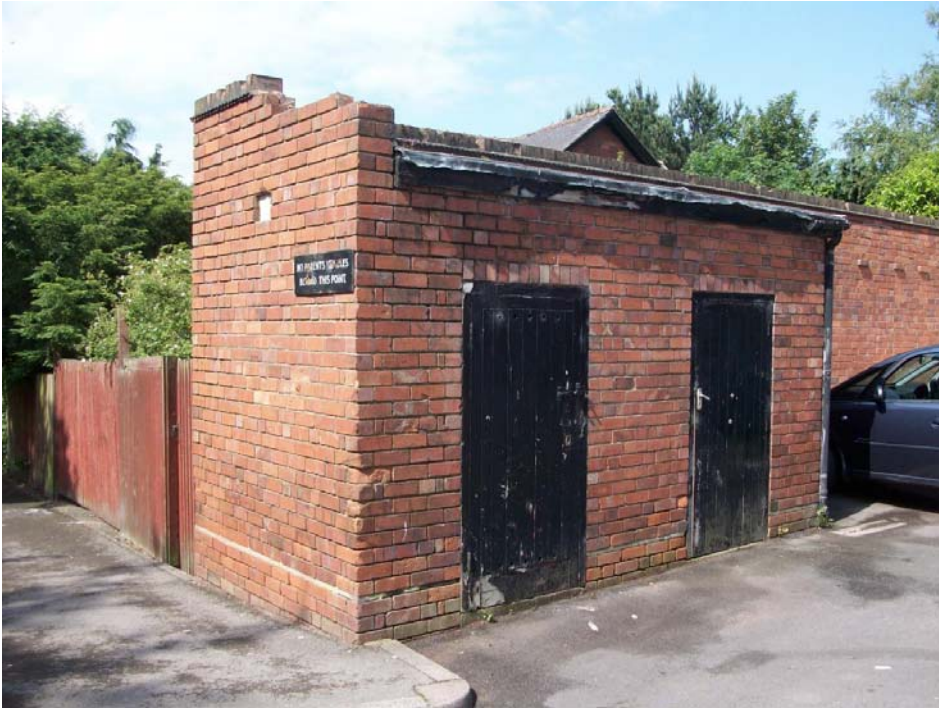
Plate 7, Outbuilding to south-east end of former cycle sheds, view west
