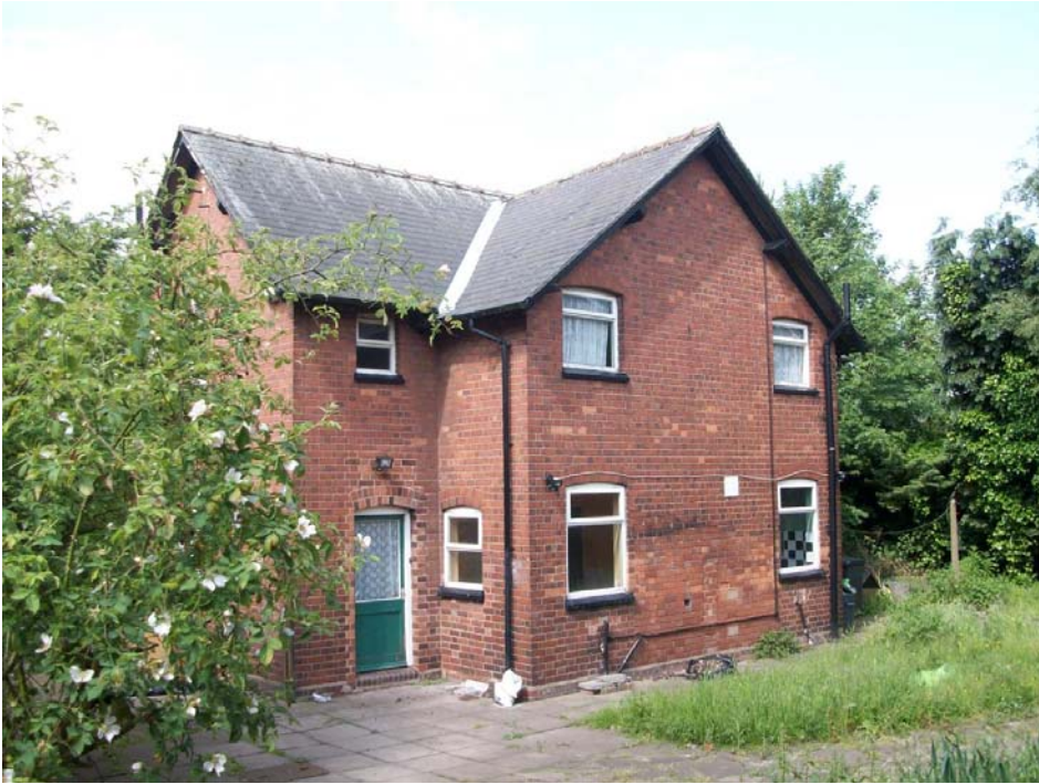
Plate 9, School Cottage, north-east elevation, view west
