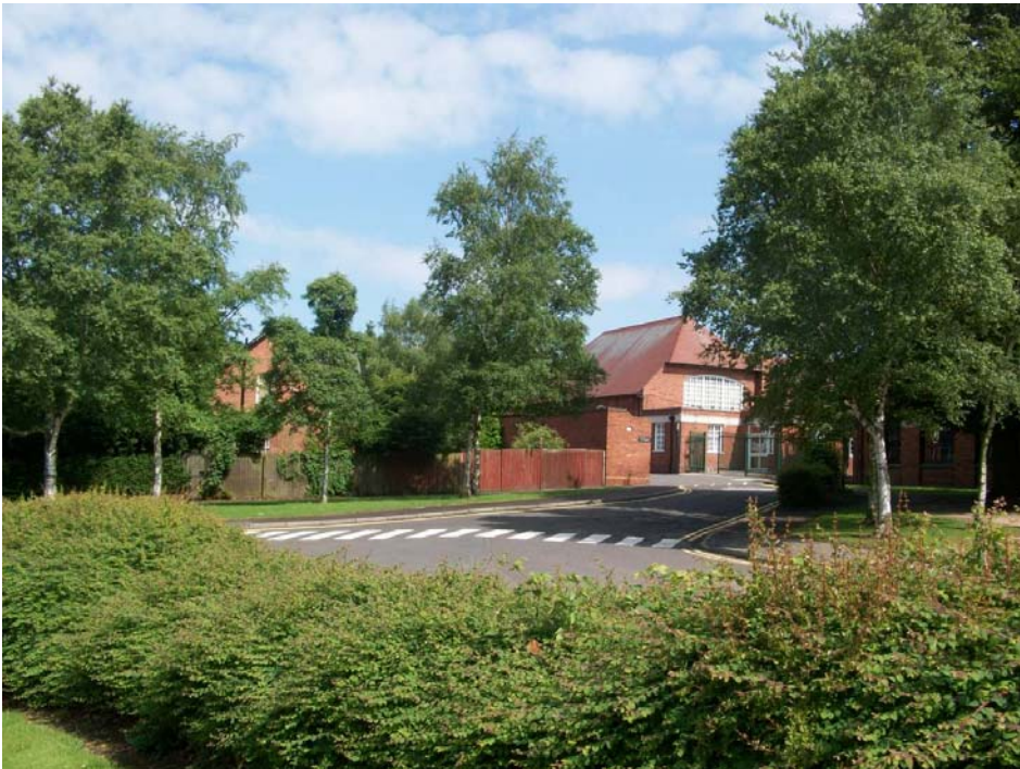
Plate 12, General view north toward 1930 school building and south access from south car park
