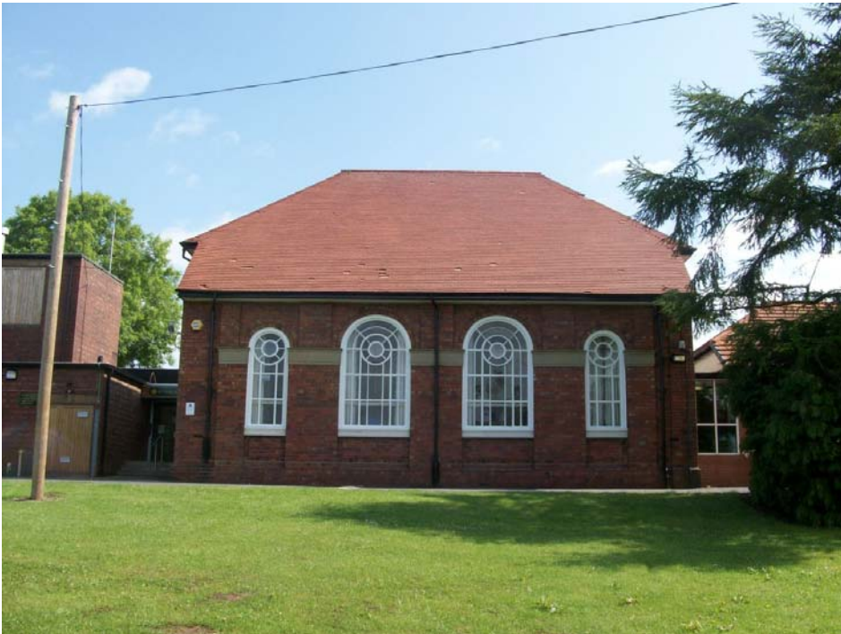
Plate 4, 1933 school building, detail of south-west elevation, view north-east (see Fig 12)
