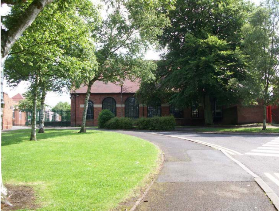
Plate 11, General view north-east toward 1931 school building, alongside south access
