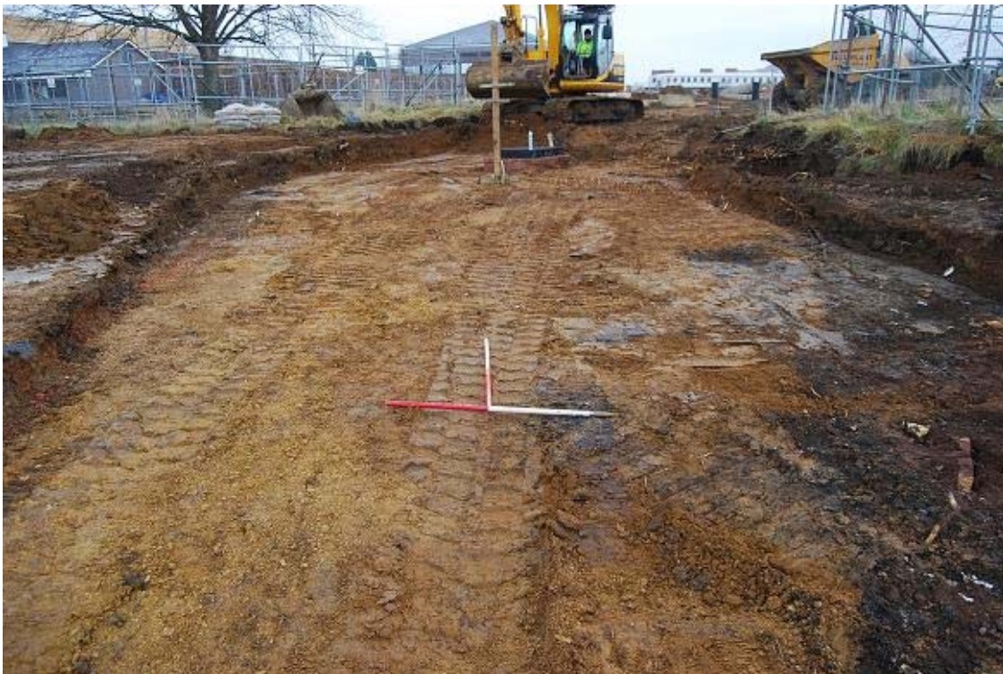
Plate 6, Area 1, road strip, view north
