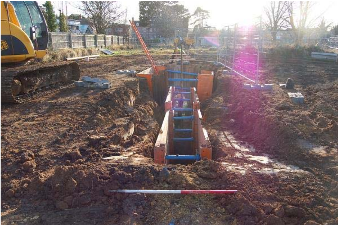
Plate 16, Area 2, Trench 1 during excavation, view south-west
