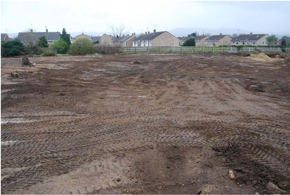
Plate 13, Area 2, general view of strip, view south-east
