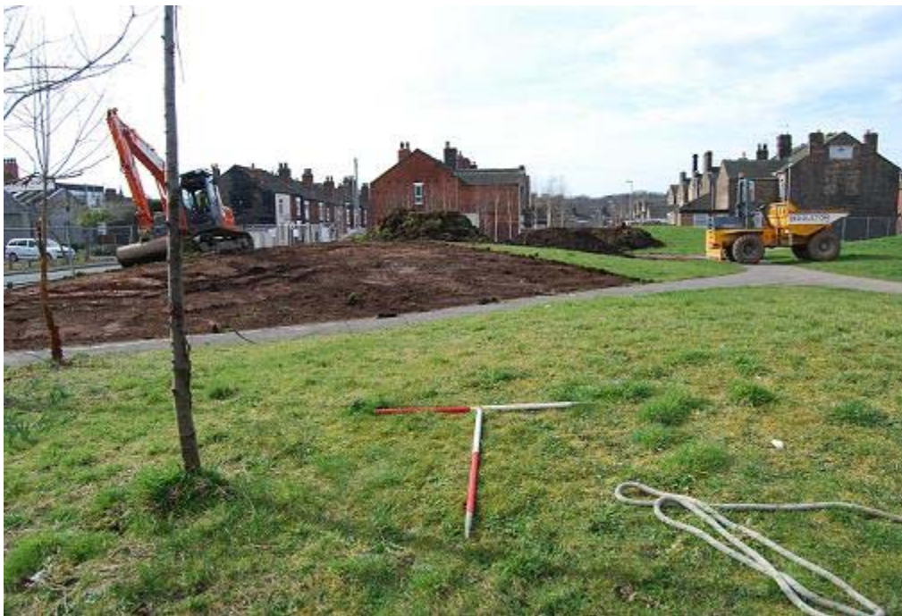
Plate 2: The site prior to the removal of the vegetation, view west
