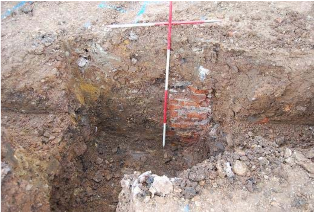
Plate 9: North-east facing section of foundation trench including wall 1007
