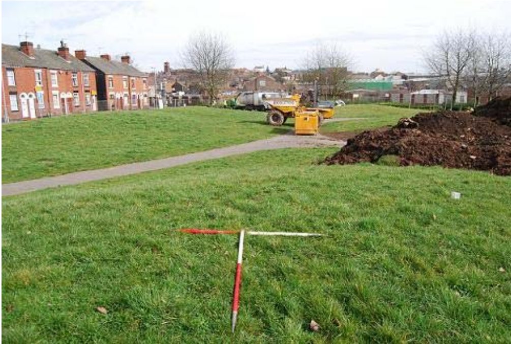
Plate 1: The site prior to the removal of the vegetation, view south-east
