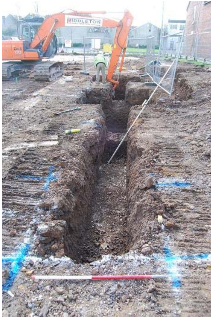
Plate 13: The site during excavation of Trench 31 and 32, view south-east
