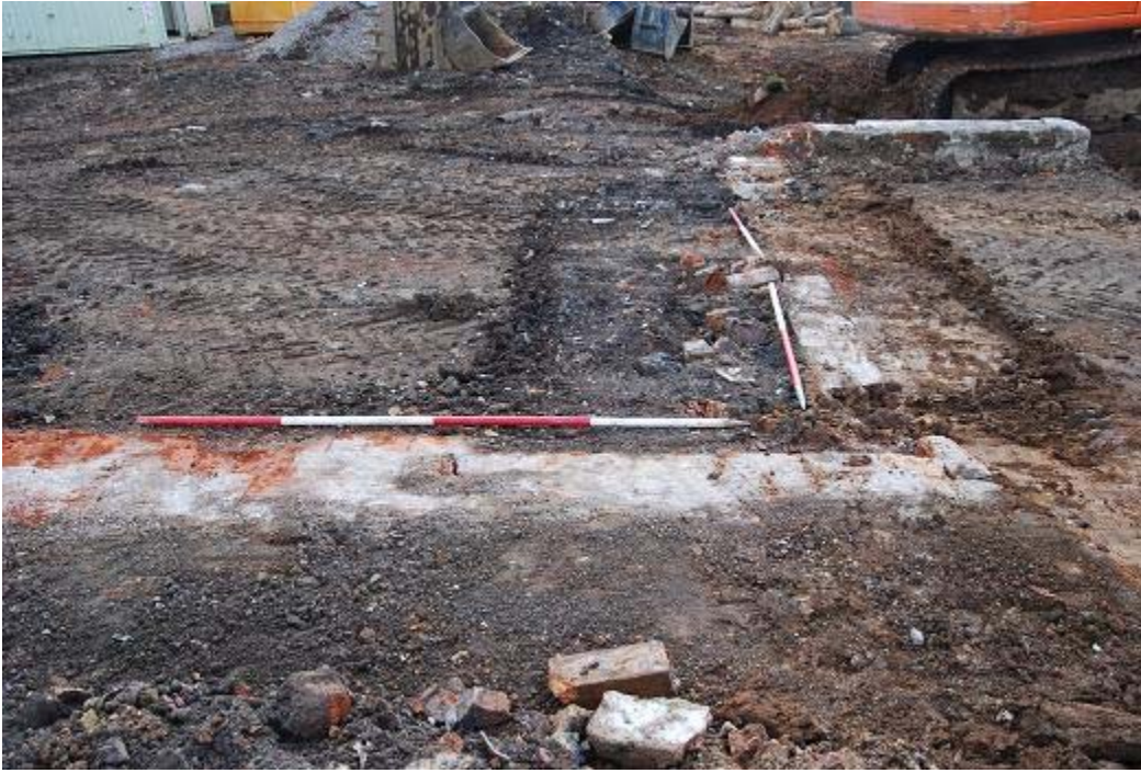
Plate 8: Wall 1007 in foreground and 1005 in right of shot, view north-west
