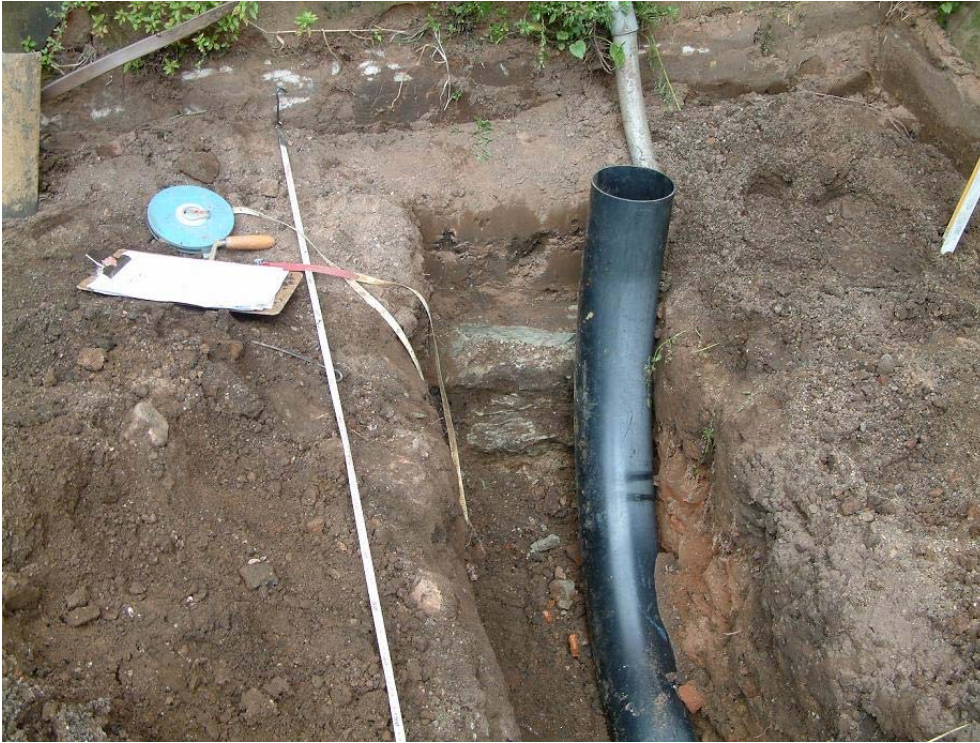
Plate 13, Area 7: sandstone foundation, 702, for south wall of church west tower, view north
