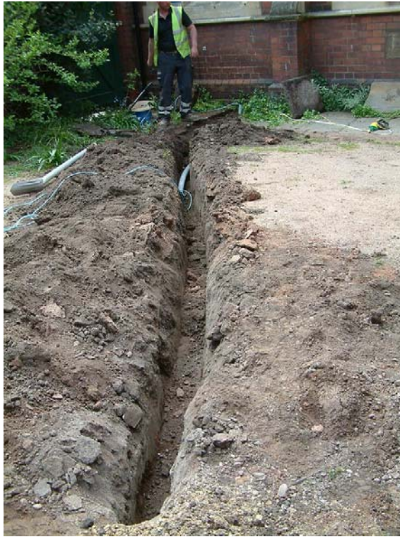
Plate 1, Area 1: trench excavation in progress; view south-west
