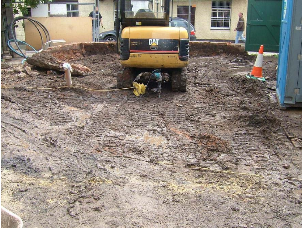
Plate 11, Area 6: reduced area in front of School House, view south
