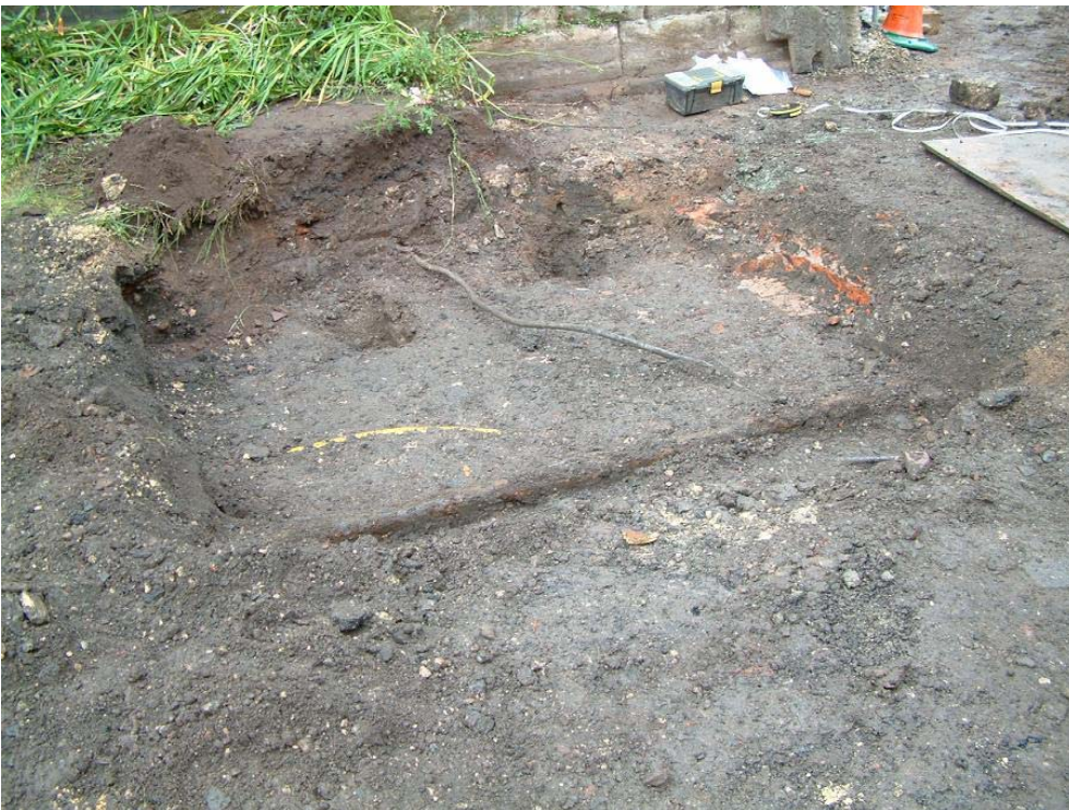
Plate 16, Area 8: general view over north brick vault, 806; brick wall 805 to south, view south-east
