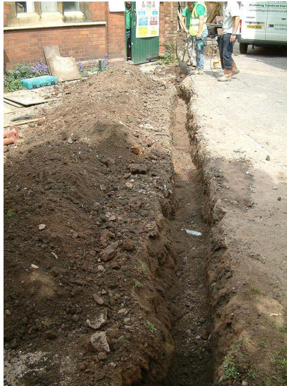
Plate 9, Area 5: General view of trench, view north-west
