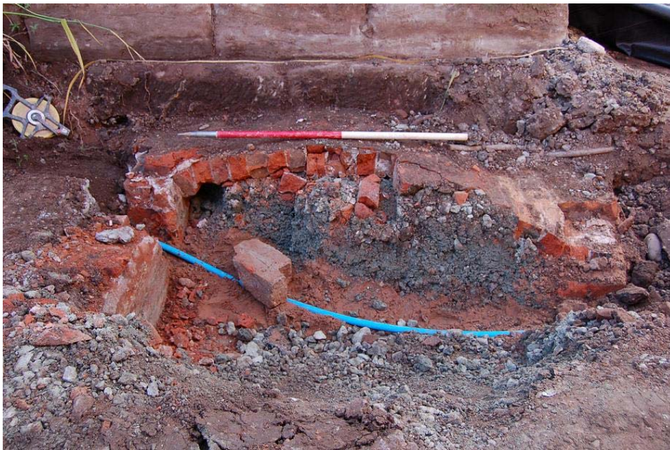
Plate 20, Area 9: south brick vault, 900, as excavated for service pipe, view east
