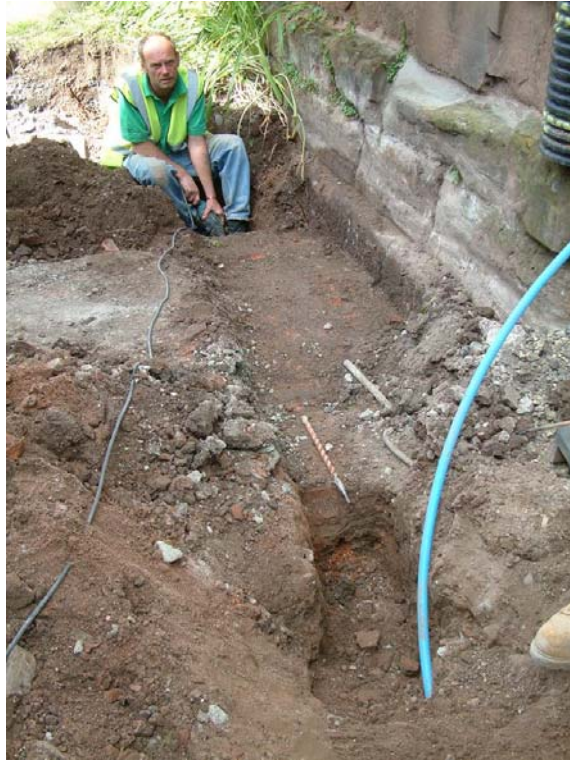
Plate 19, Area 9: south brick vault, 900, as exposed, view north
