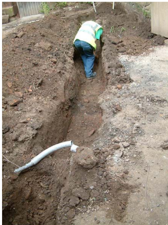
Plate 14, Area 7: work in progress, view north
