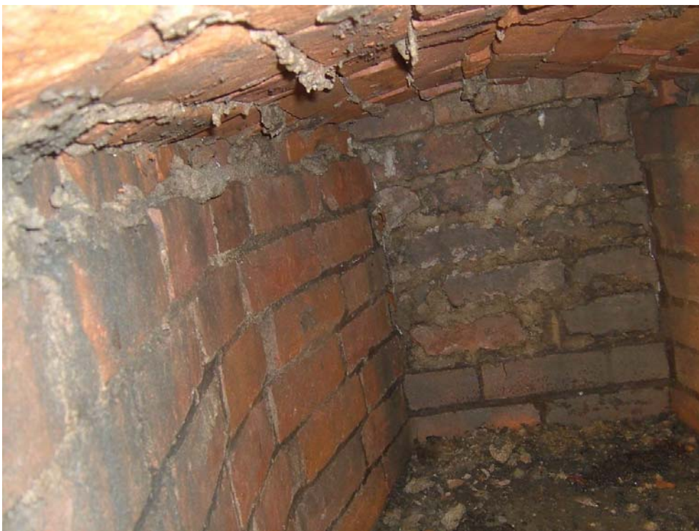
Plate 18, Area 8: brick vault, 806, interior, west end with rough mortared access
