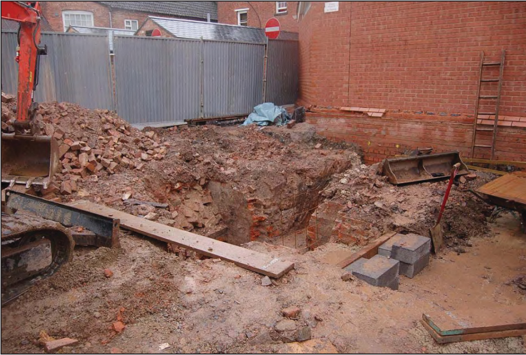
Plate 4, General view of foundation trenches facing south-west
