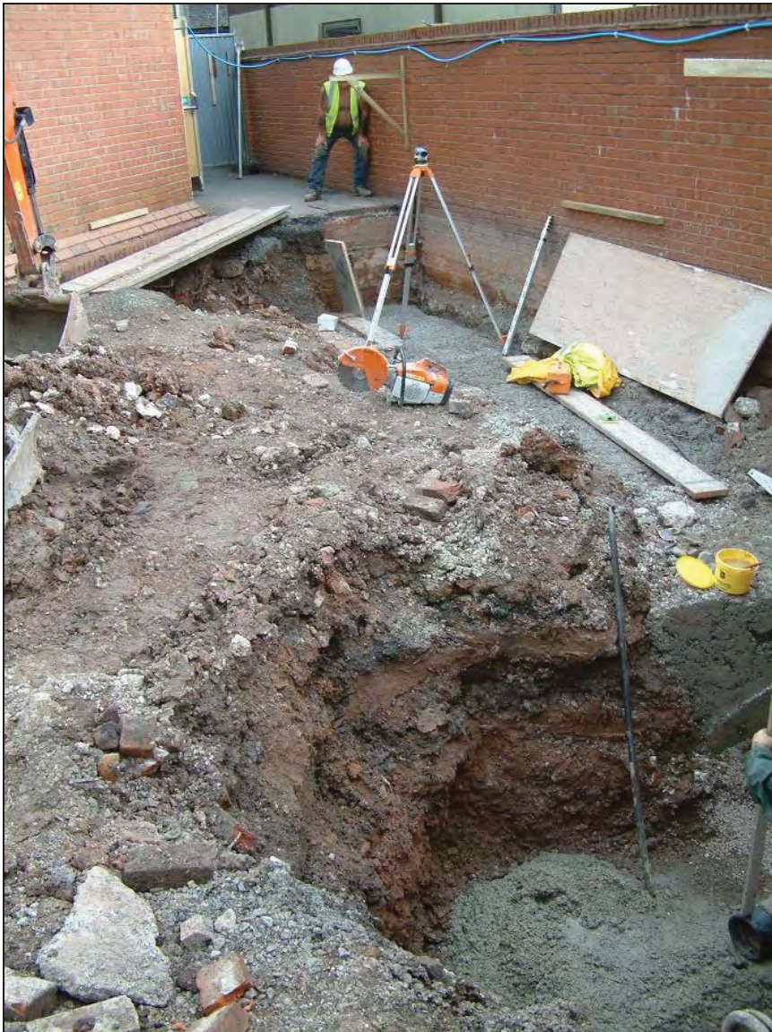
Plate 1, General view of (backfilled) sewer trench and manhole
