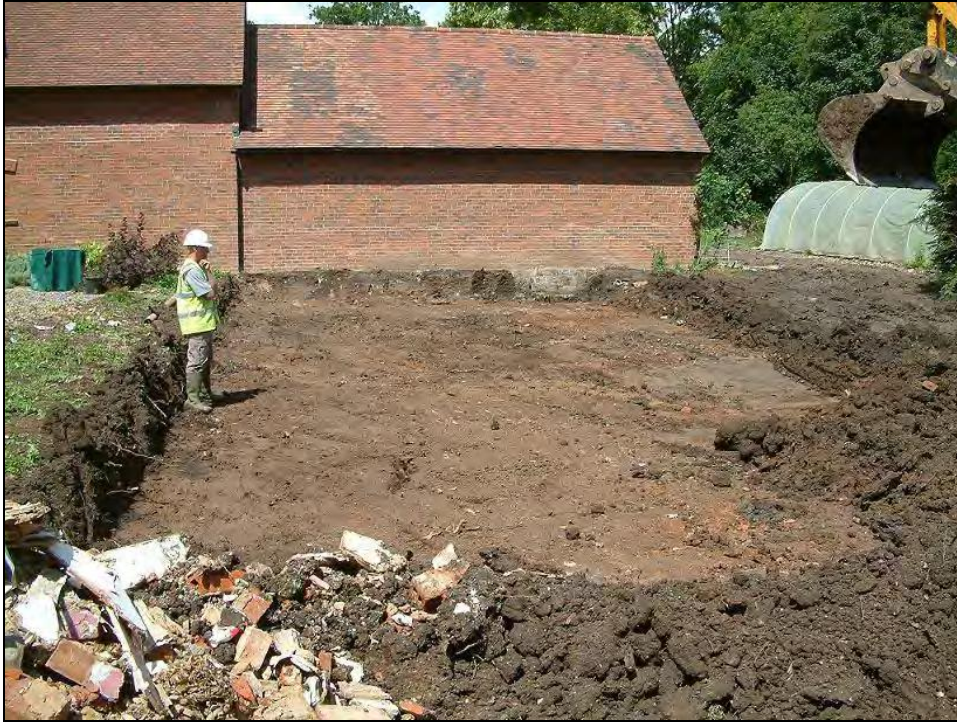
Plate 1, General view north of the site after excavation of initial spit
