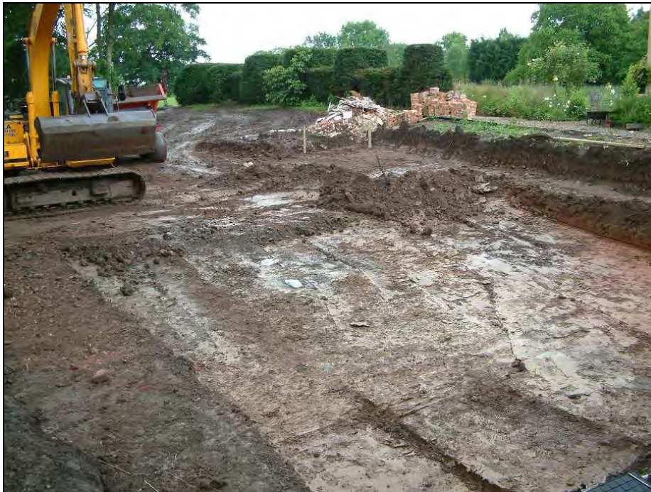
Plate 8, View south-west of excavation of lower level in progress
