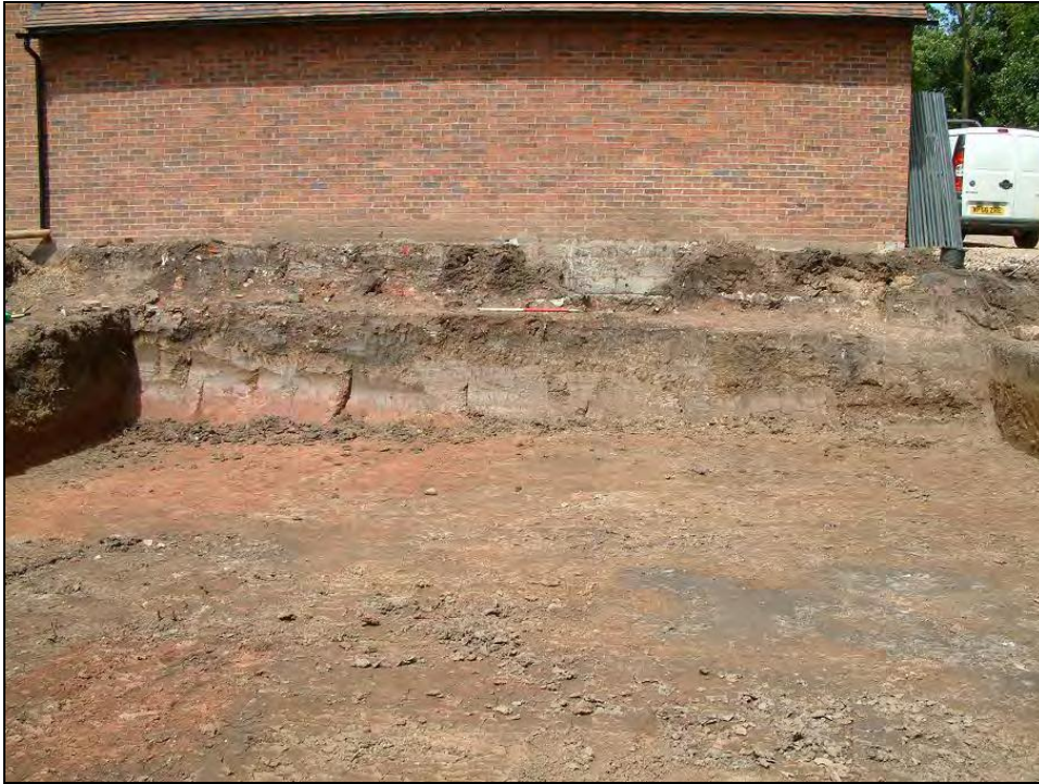
Plate 13, General view north of north baulk and full depth of excavation
