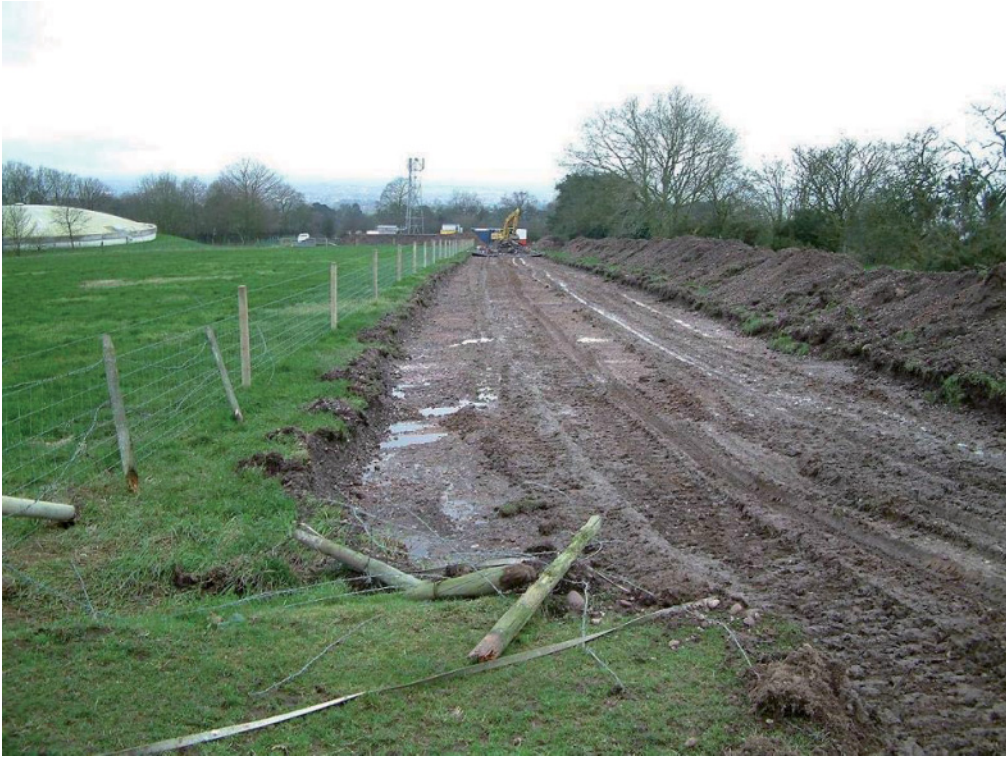
Plate 8: Trench 5, access track from Trench 4 to sewage pipeline, looking southwest
