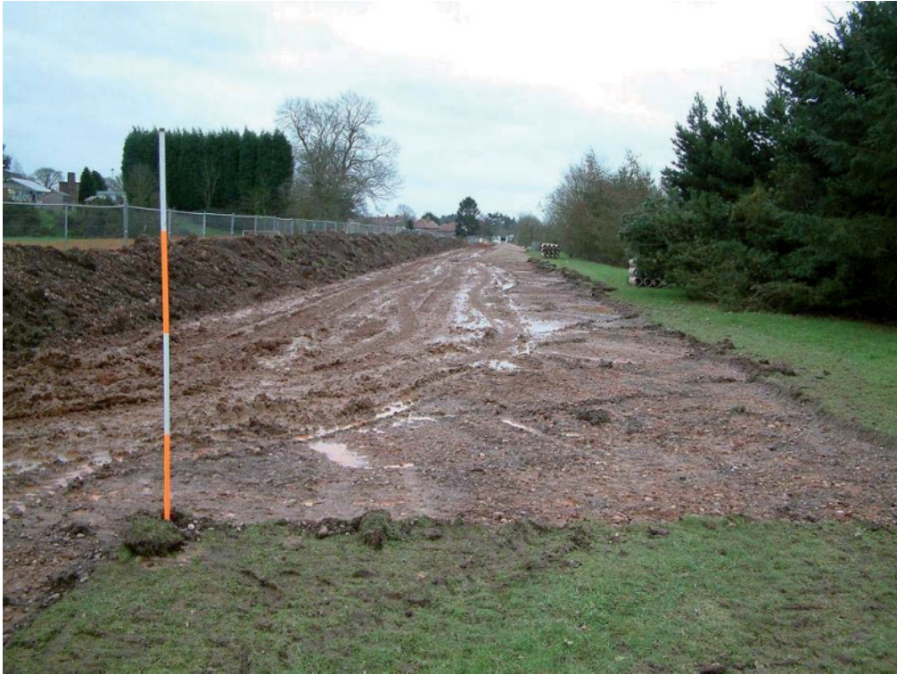
Plate 10: Trench 7 in school playing field, looking southeast
