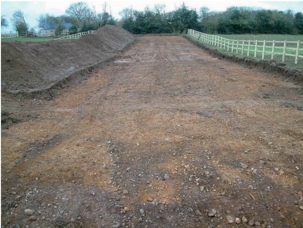
Plate 9: Trench 6, looking northwest
