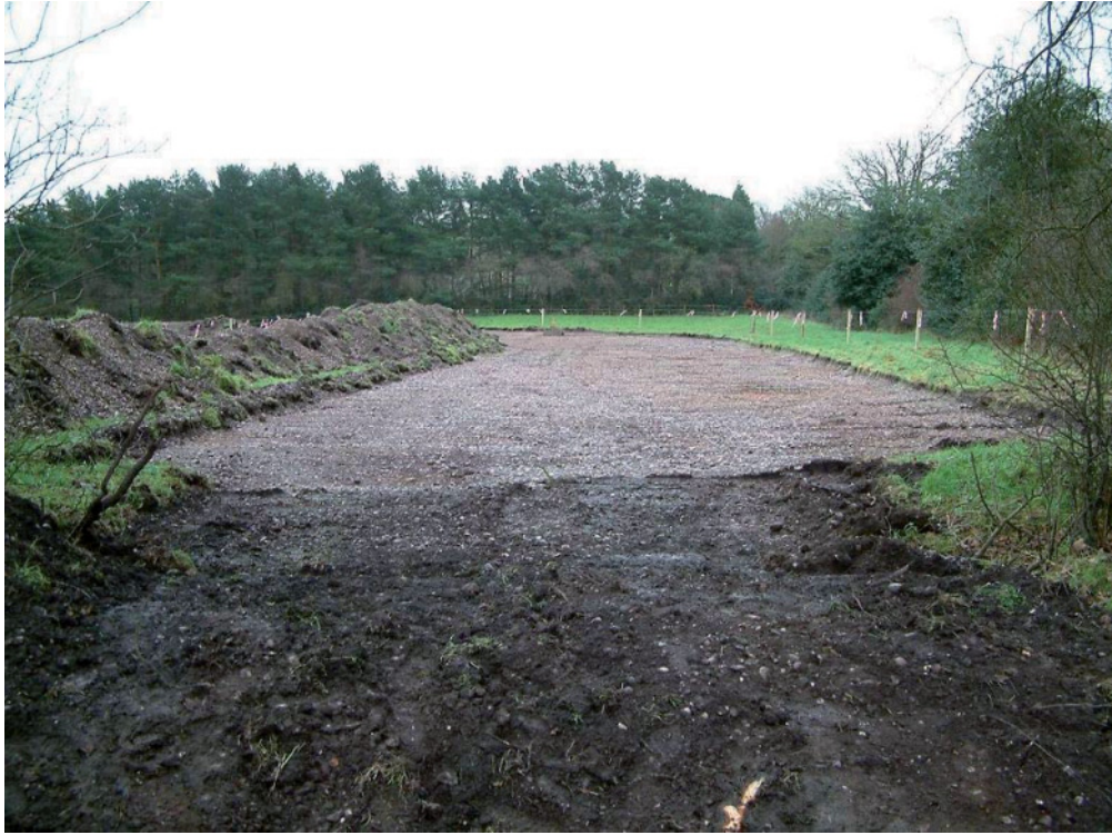
Plate 3: Trench 2, looking east southeast
