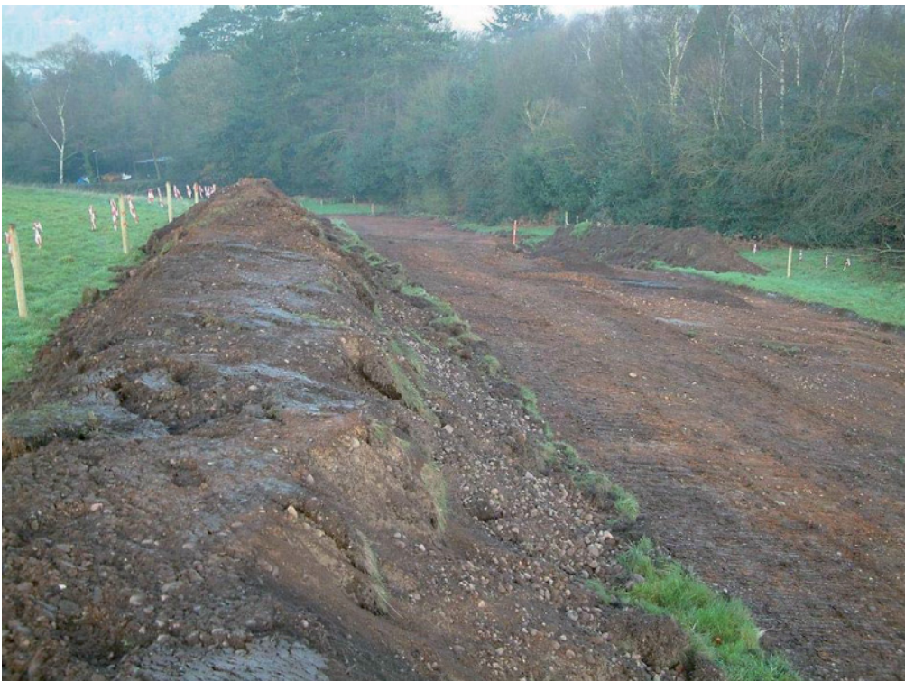
Plate 2: Trench 2, looking northeast
