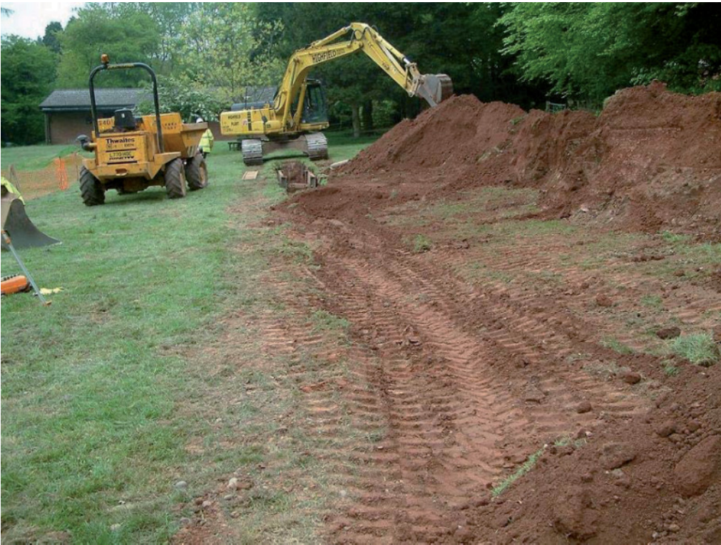
Plate 15: Excavation of the pipe trench in Trench 10 looking northeast.
