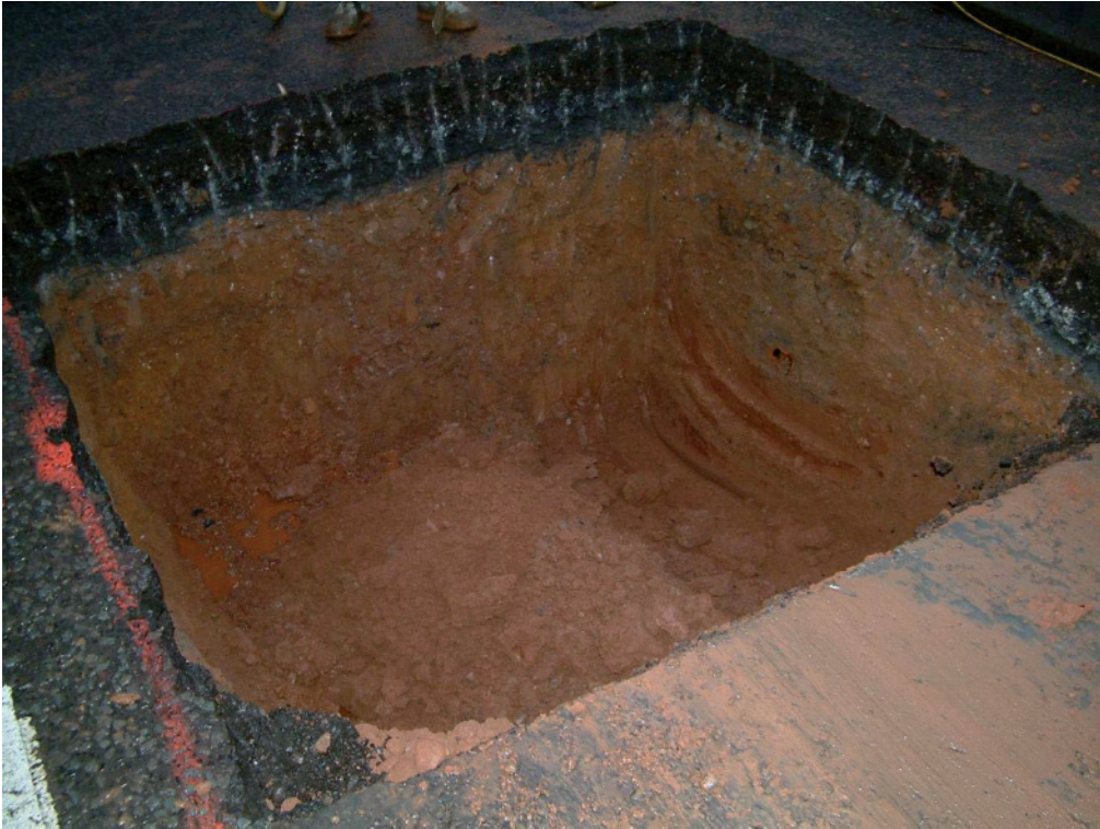
Plate 6: Trench 3 in Old Birmingham Road, looking northeast
