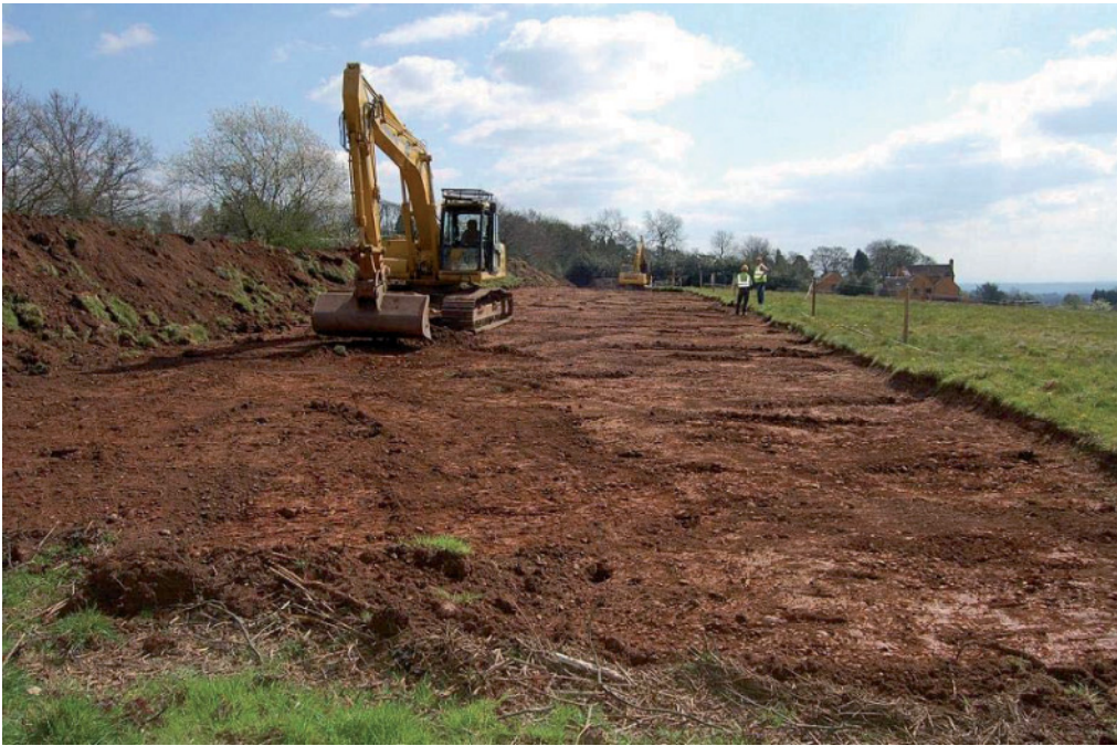
Plate 14: Stripping the easement in Trench 9, looking southeast
