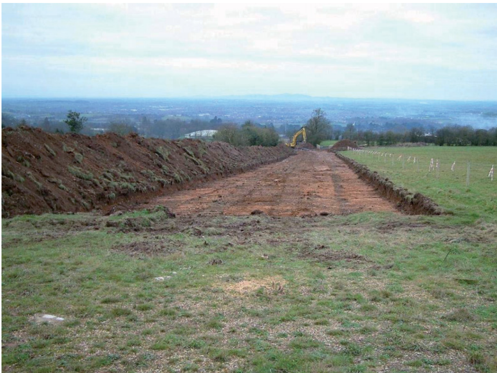
Plate 13: Trench 9 looking southwest
