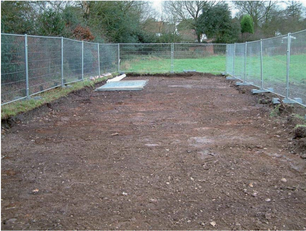
Plate 1: Trench 1 off Monument Lane after soil stripping, looking northwest
