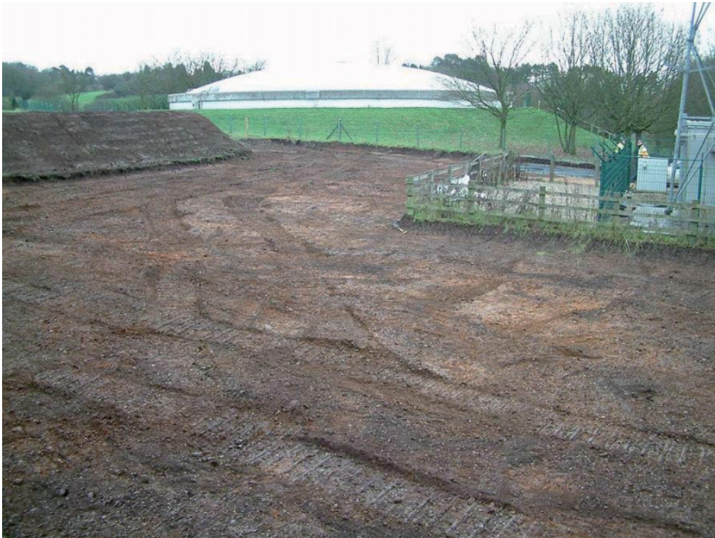
Plate 7: Trench 4, compound off Alvechurch Highway, looking east
