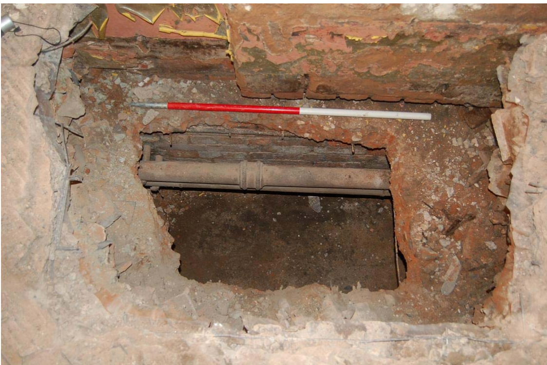
Plate 2 Service duct, test pit 1
