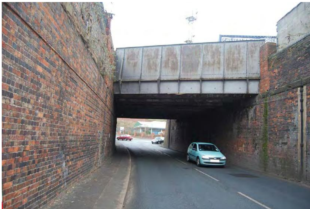
Plate 10. The west side of the bridge from street level. Looking east.
