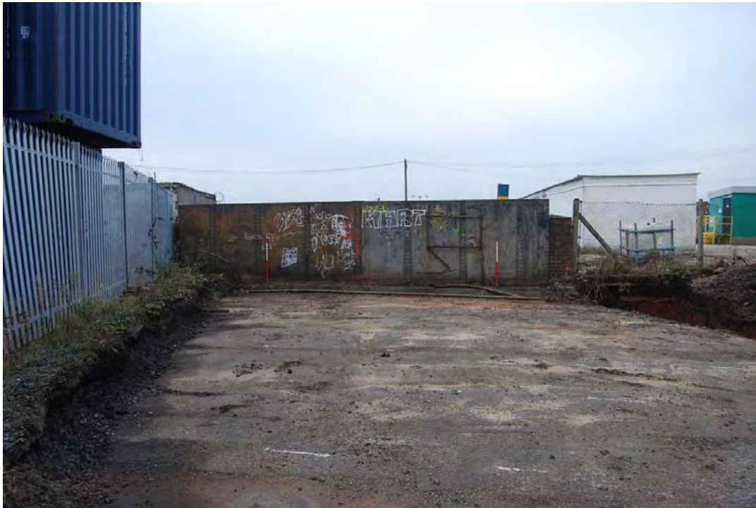
Plate 8. Showing the top of the western side of the former railway bridge. Looking west.
