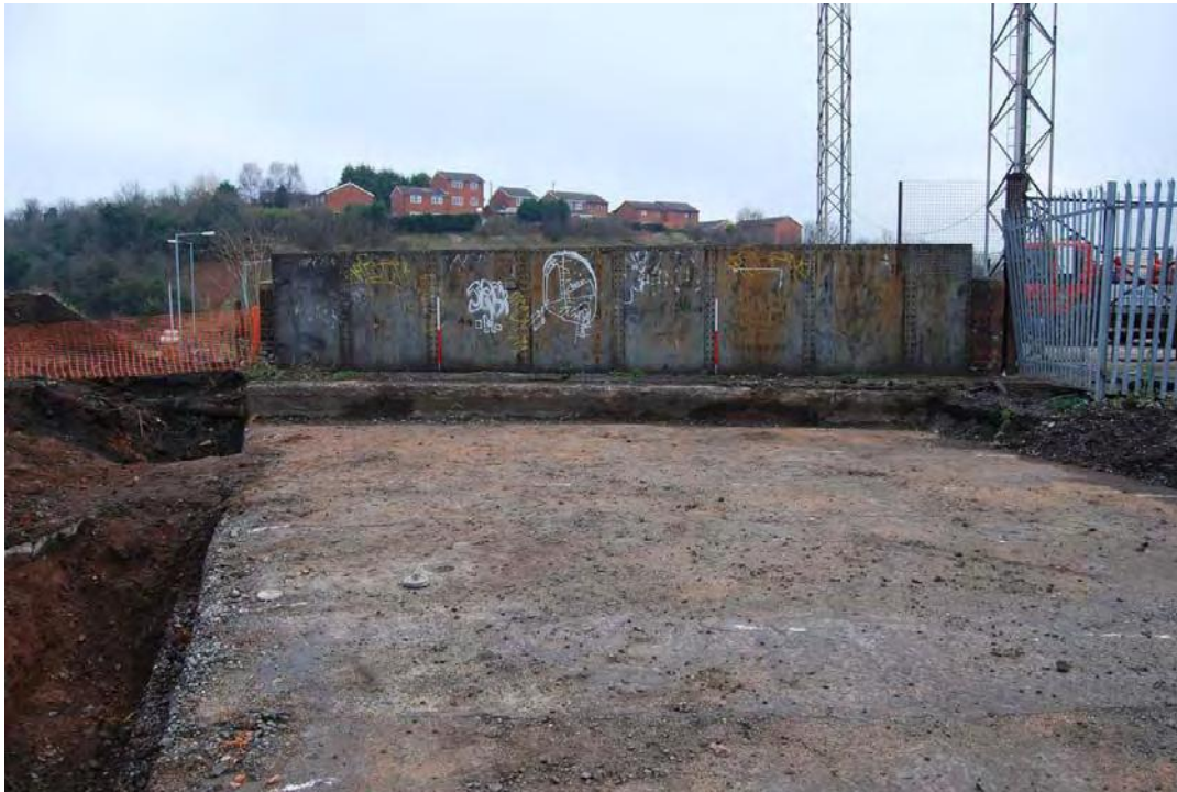
Plate 6. Showing the top of the eastern side of the former railway bridge. Looking east
