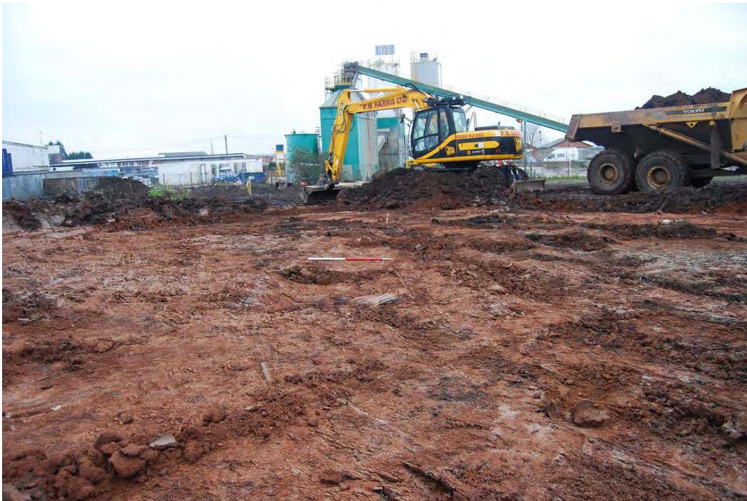
Plate 2. Stripping of the access road. Looking southwest.
