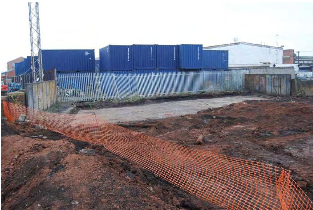
Plate 9. Showing the top of the former railway bridge with its steel sides and concrete deck. Looking southwest.
