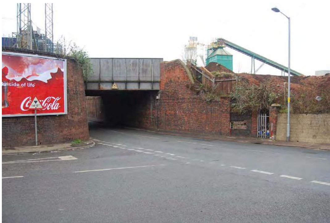
Plate 14. The eastern side of the bridge with its retaining wall.
