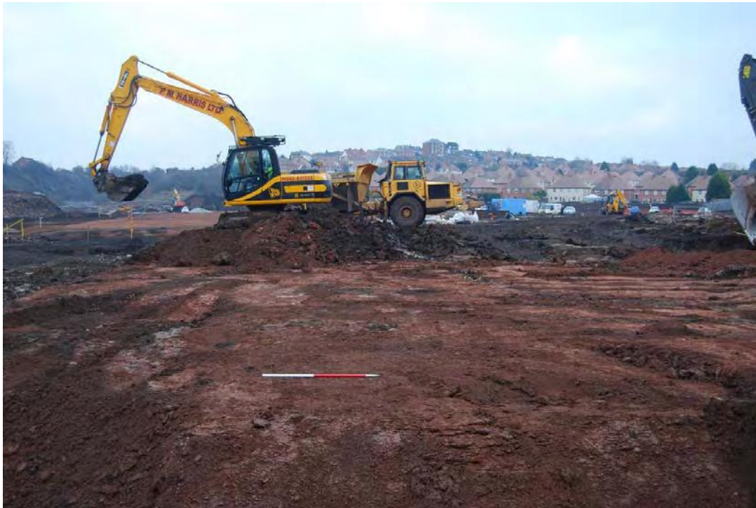
Plate 3. Further stripping of the access road. Looking north.
