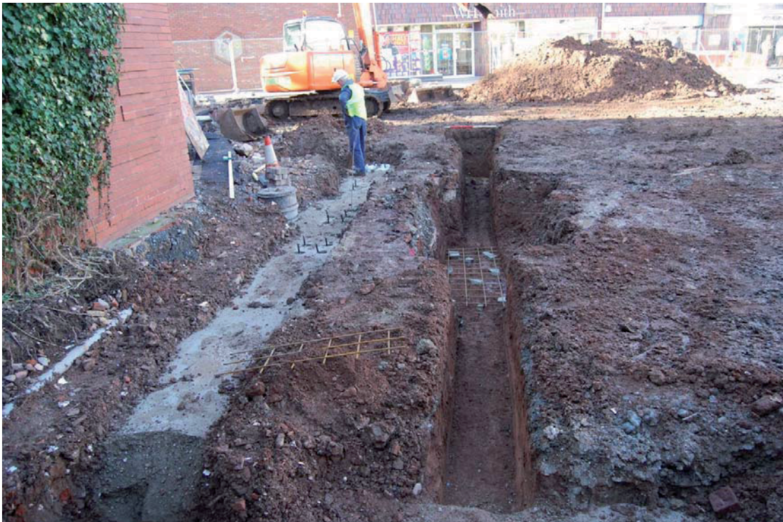
Plate 5. Area 2: Foundations to the southwest of the site; looking northwest
