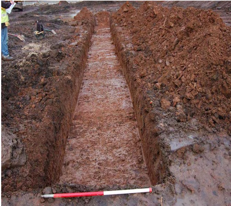
Plate 3 Trench 1 looking north-west
