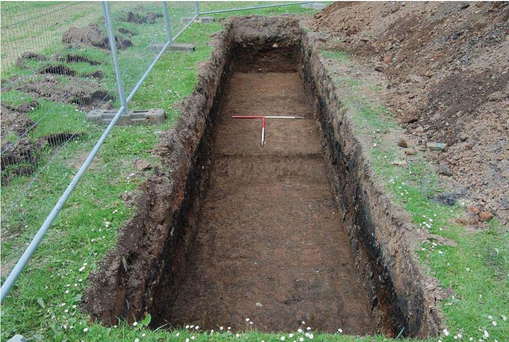
Plate 1, Trench 2, general view northwest
