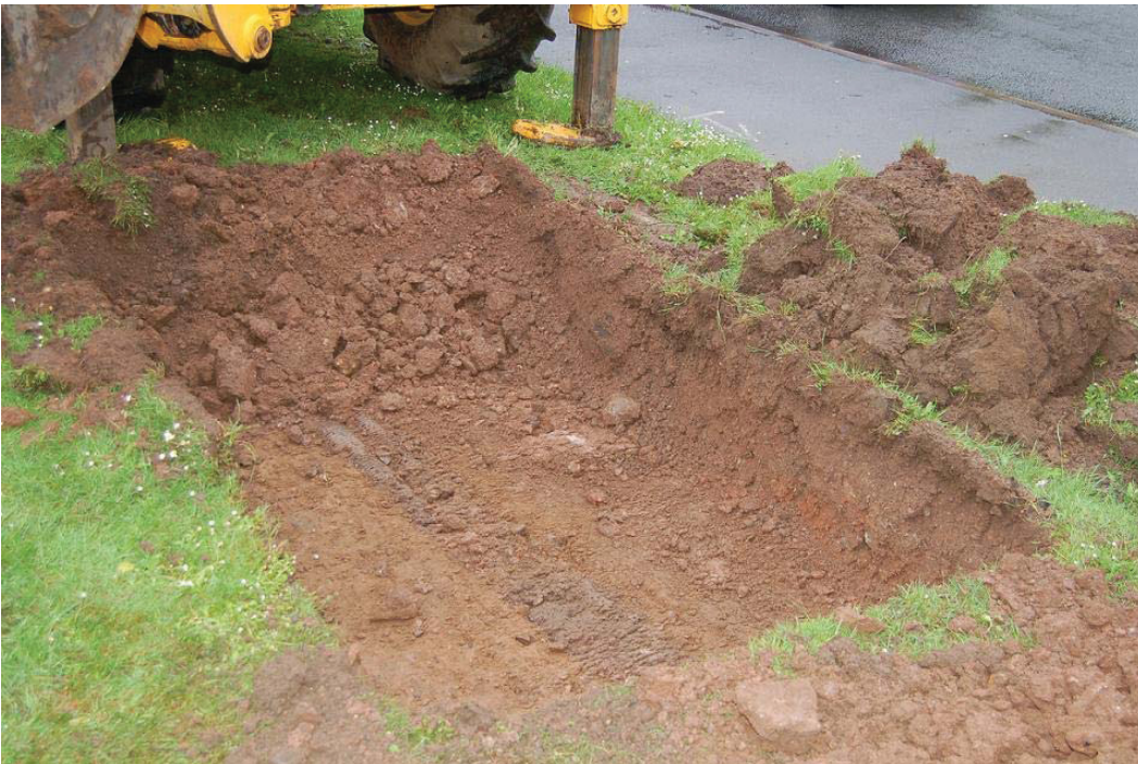
Plate 6, Trench 5, excavation in progress, view south showing live services
