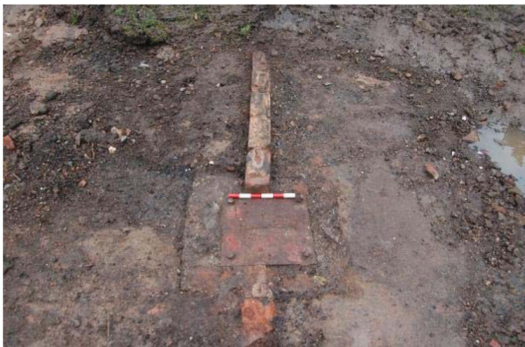
*Plate 3: Trench 1, concrete pillar base 115, with imbedded metal plate and bolts, view northeast*
