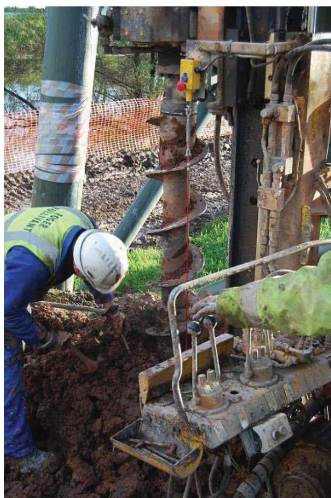
*Plate 24: Drilling of the pile foundations for retaining wall, view southeast*
