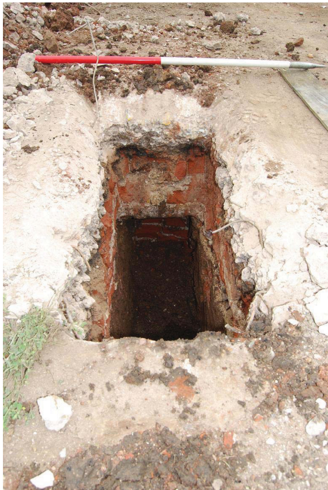
Plate 4, Test Pit 2, brickwork 202, view south west
