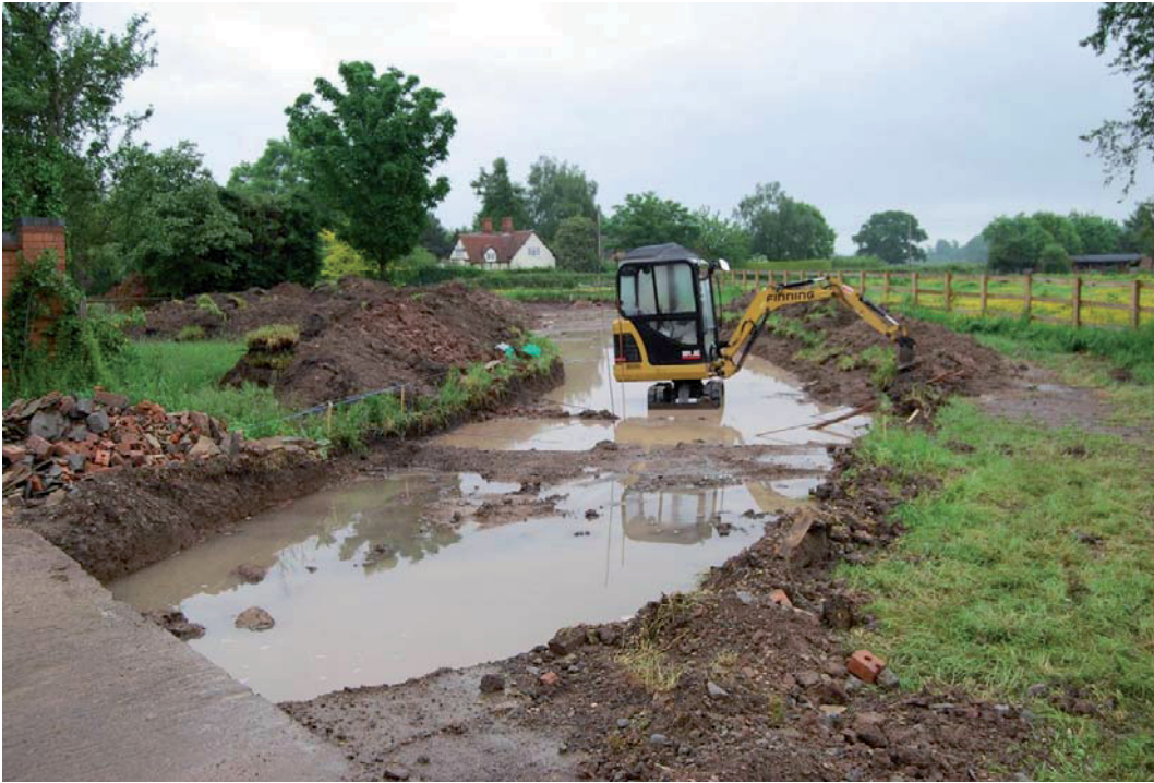
Plate 1 Looking north-east showing southern end of site flooded after site strip
