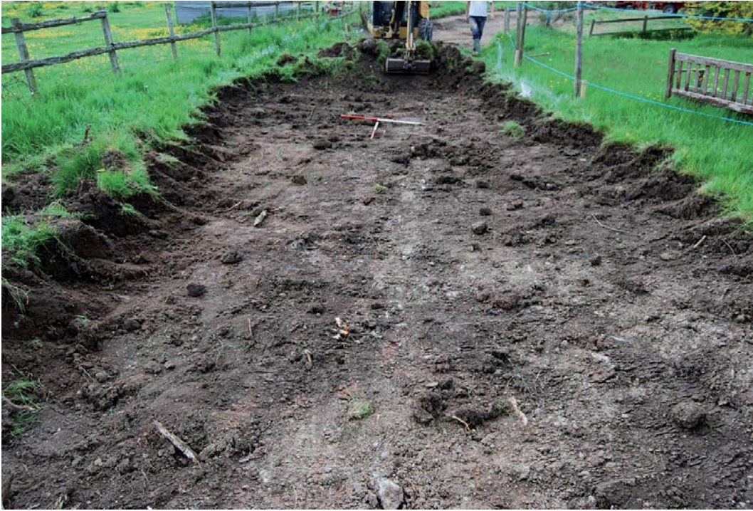
Plate 4 Looking south, northern part of site strip showing layer (106)
