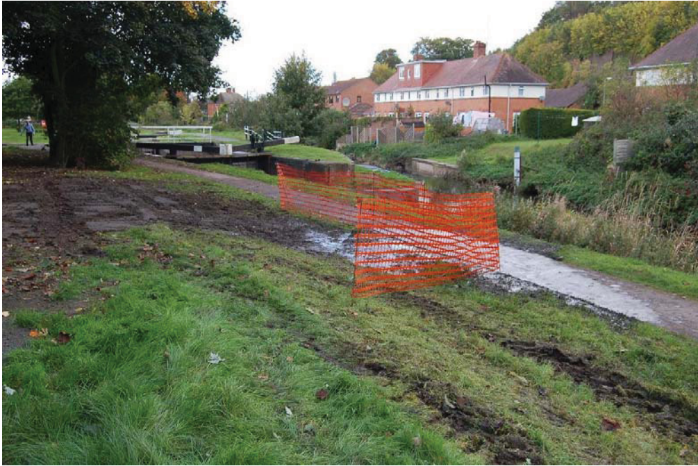
Plate 5 Trench as backfilled, view west-north-west
