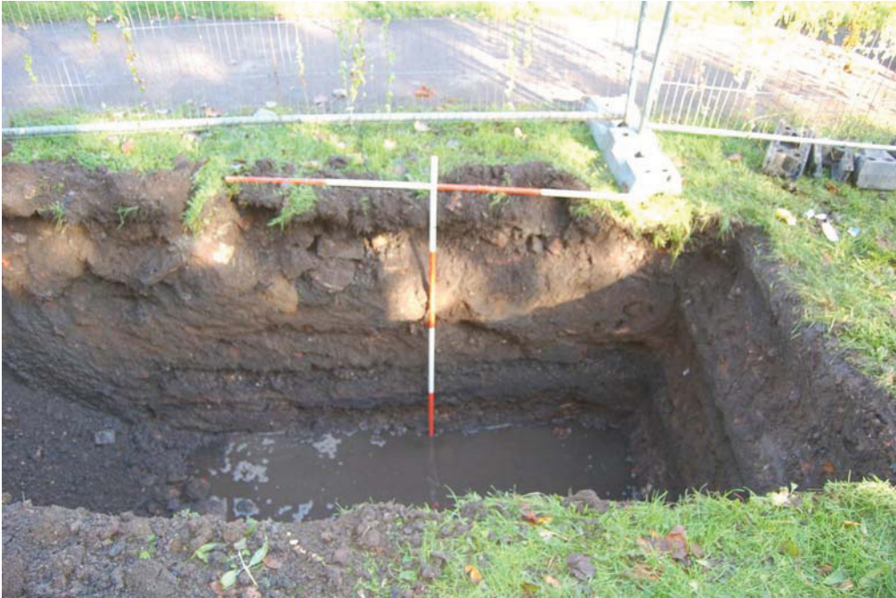
Plate 1 General view of north section of trench
