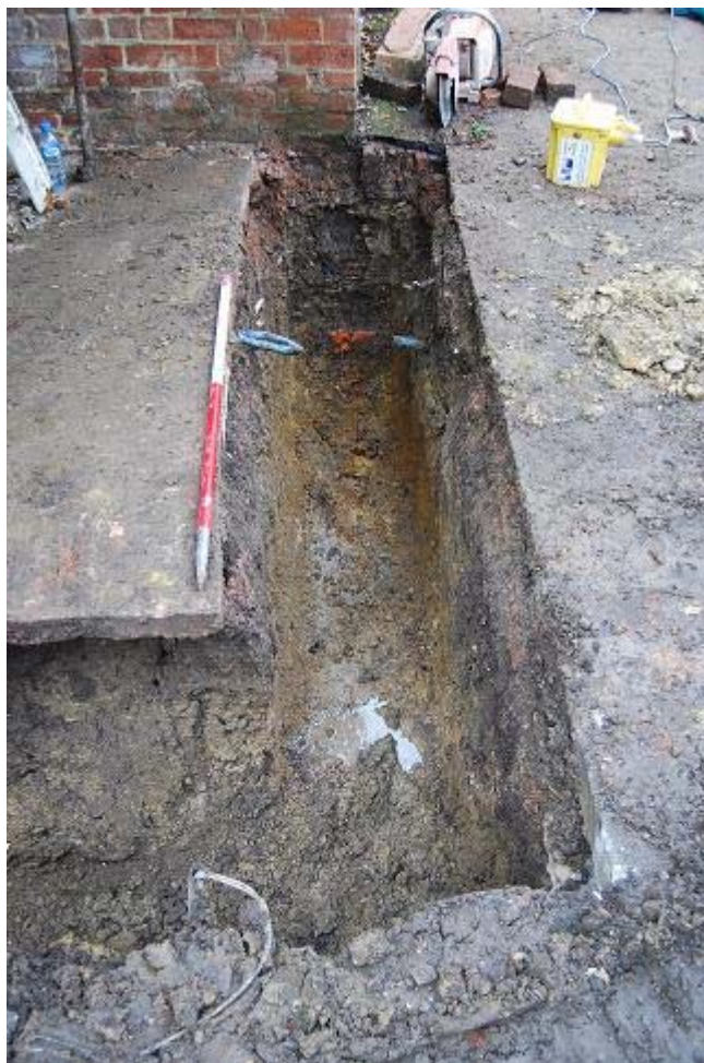
Plate 11: Trench 7, looking west.
