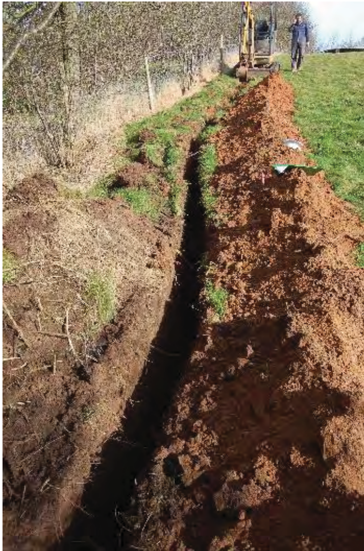
Plate 2: Overview of trench one, facing north east.
