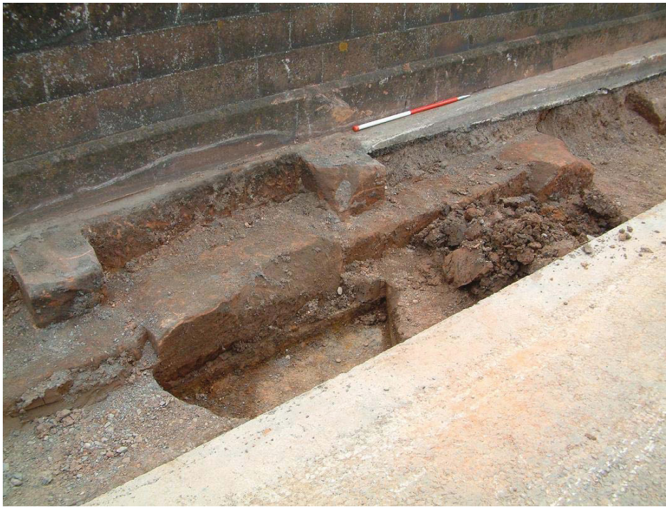
Plate 9, Detail of parapet foundation 1018 and decking plates 1021 over south arch, view south
