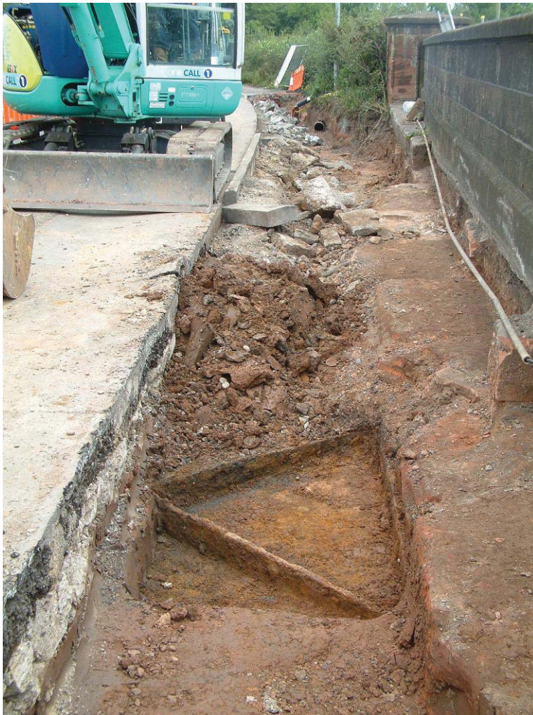
Plate 7, Decking plates 1020 in southwest footpath over north arch, view northeast
