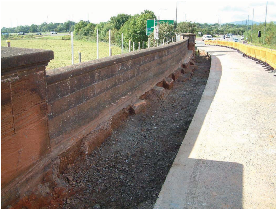
Plate 6, Parapet foundations 1018 to southwest of main arch, view southwest
