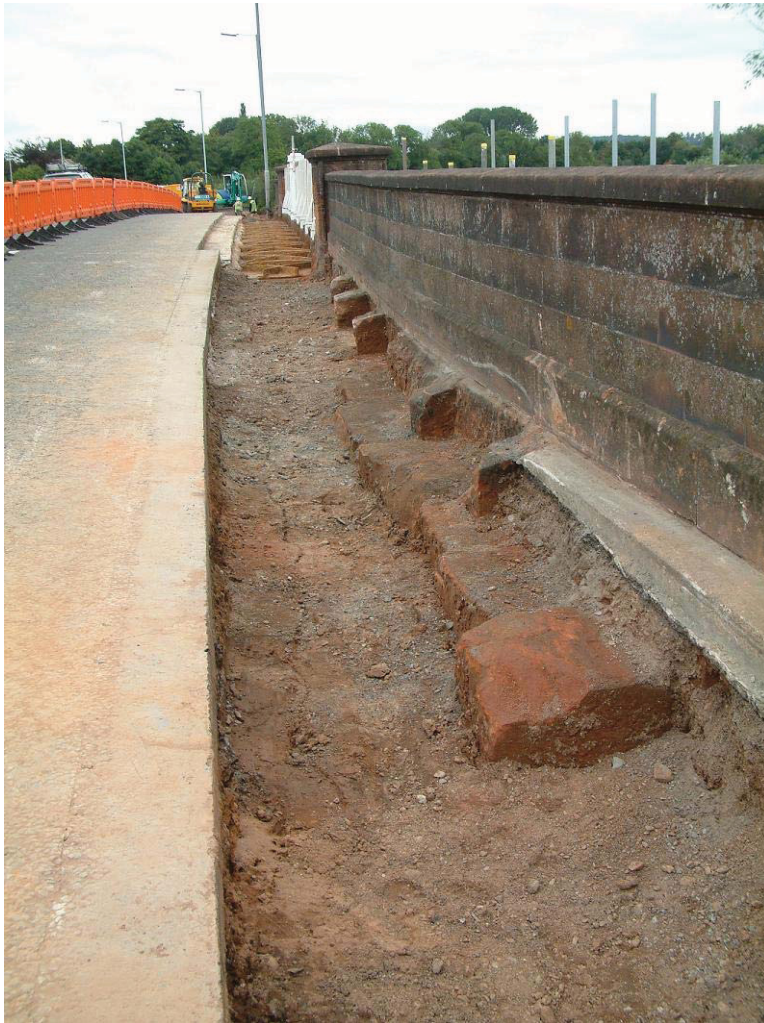
Plate 8 Parapet foundations 1018 to southwest of main arch, view northeast
