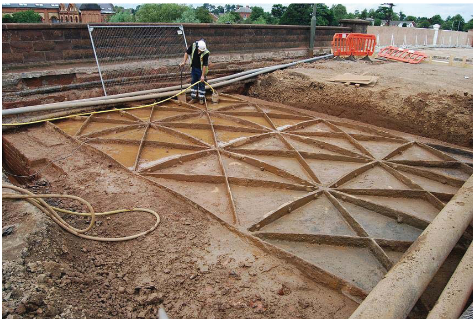
Plate 12, Decking plates 1021 in Trench 6 over south arch, view north
