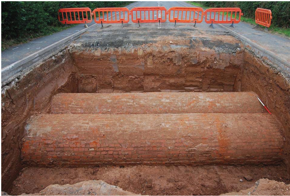
Plate 16, Culverts 2007 and 2008 in Trench 3, view north northeast
