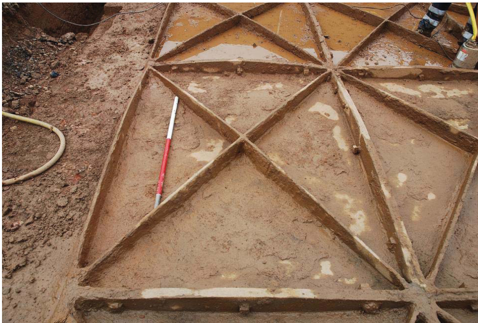
Plate 14, Detail of decking 1021 in Trench 6 with brick pier 1025 partially exposed to left
