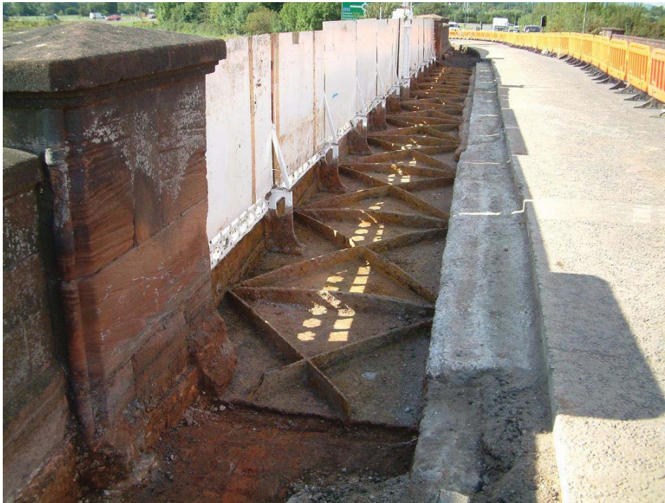
Plate 5, Decking plates 1022 in southwest footpath over main arch, view southwest
