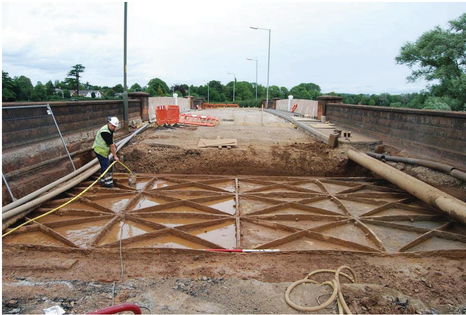
Plate 13, Decking plates 1021 in Trench 6 over south arch, view northeast
