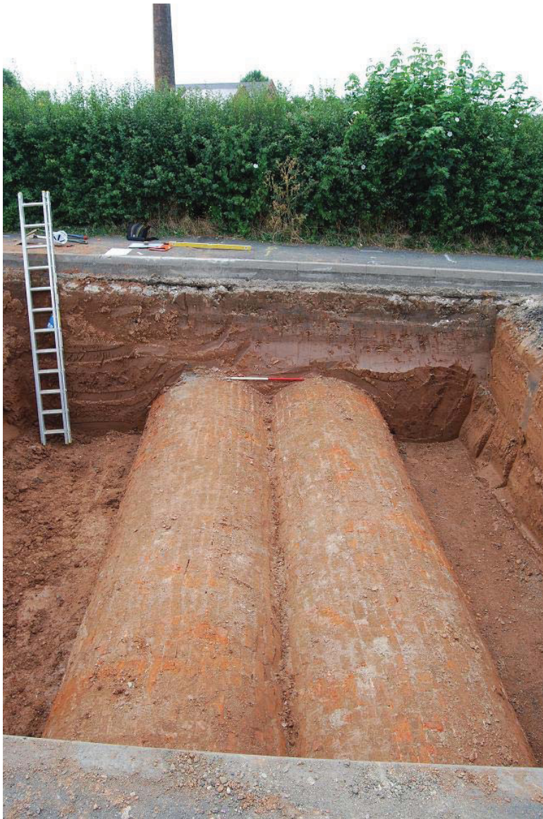
Plate 15, Culverts 2007 and 2008 in Trench 3, view west northwest
