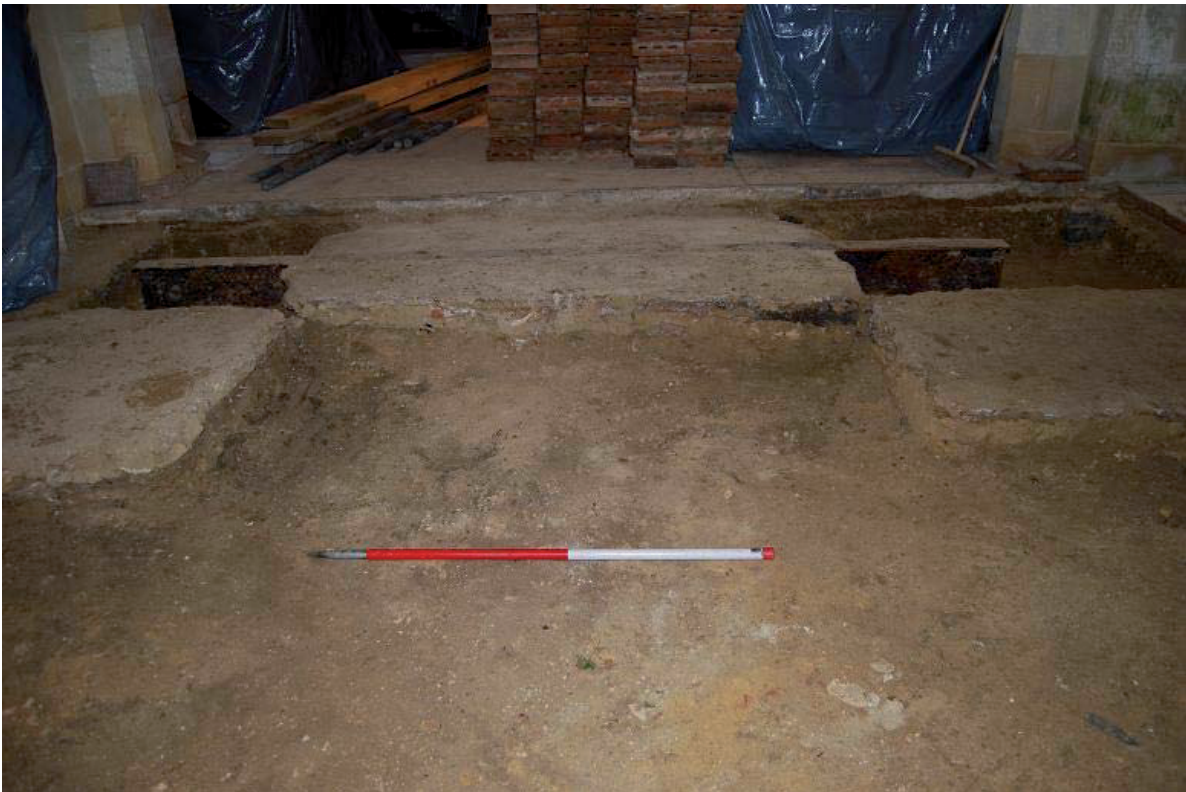
Plate 10 Concrete bases 10012 and steel 10013, facing east
