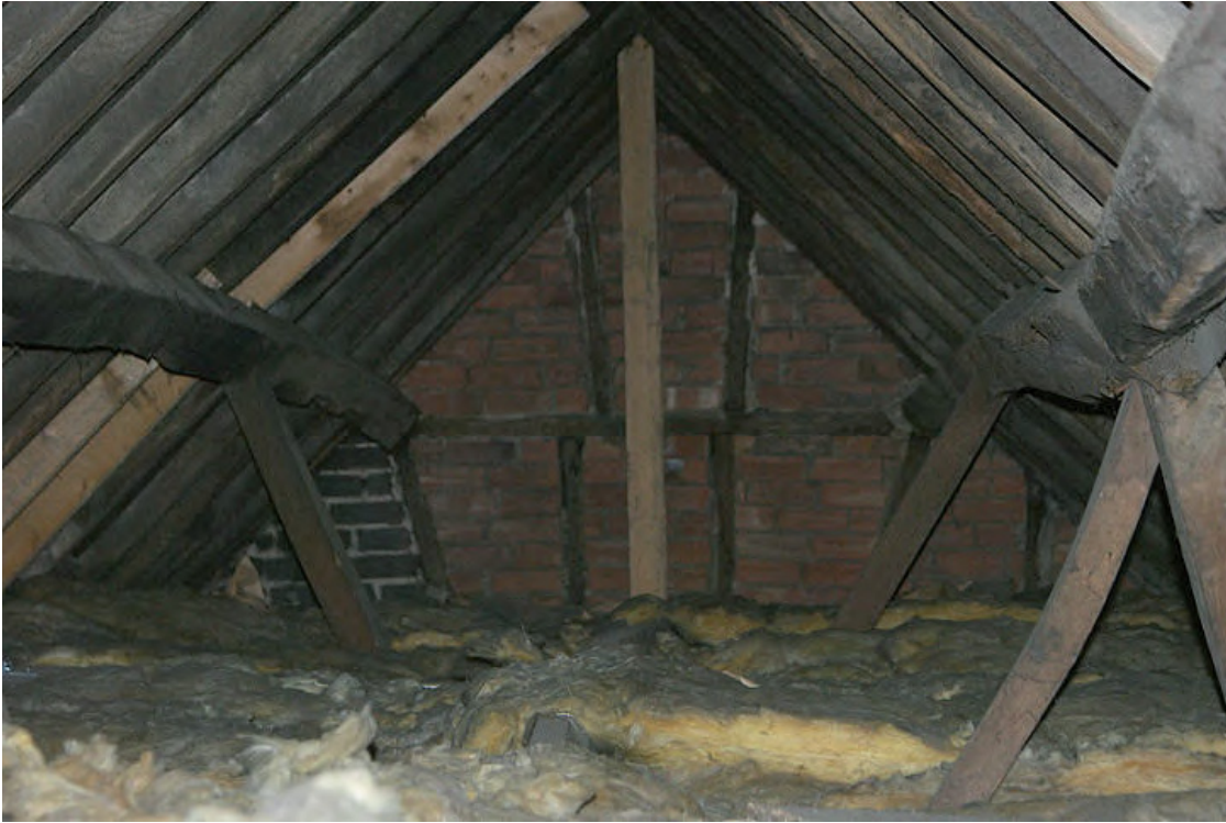
Plate 19: Timber frame wall in roof space of 38, Cowl Street
