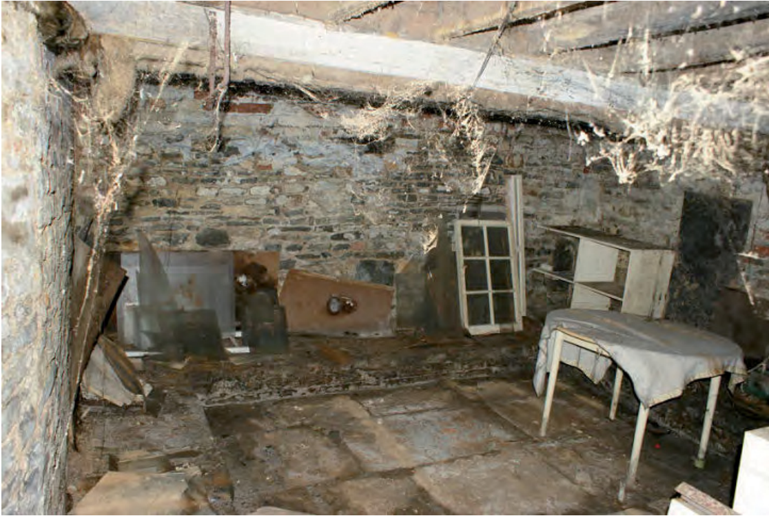
Plate 16: Stone cellar of 33, Cowl Street
