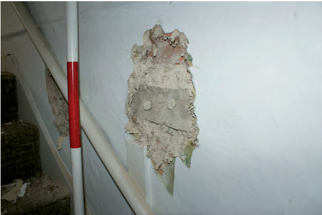
Plate 17: Part of timber frame wall in 36, Cowl Street
