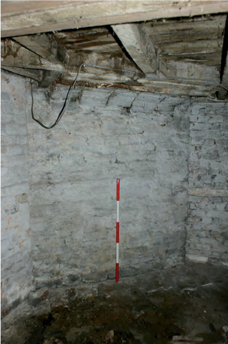
Plate 15: Medieval stone pier in the cellar of 38, Cowl Street
