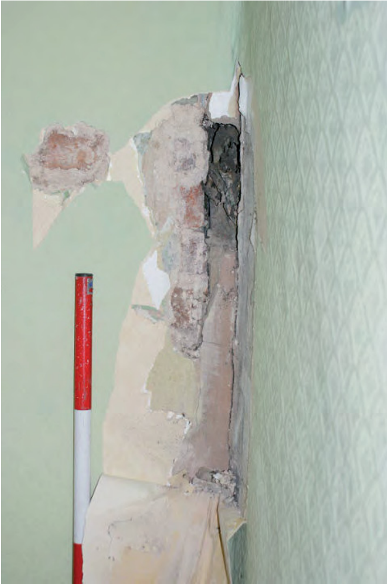
Plate 22: Detail of frontage wall (on right) and 17 th century internal wall, with gap between the two (sample comparable in each of 35-38, Cowl Street)
