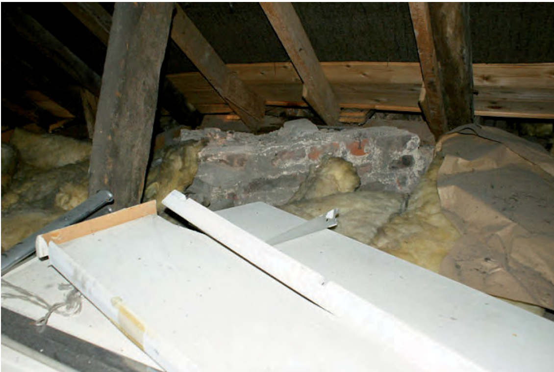
Plate 24: Top of brick chimney stack in roof space of 35, Cowl Street
