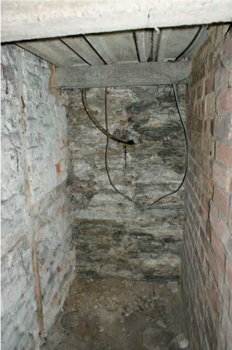
Plate 14: Cowl Street frontage, medieval stone wall in cellar of 38, Cowl Street
