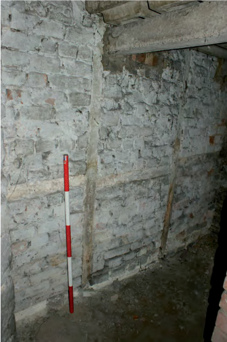
Plate 18: 17 th century timber-frame in cellar of 38, Cowl Street
