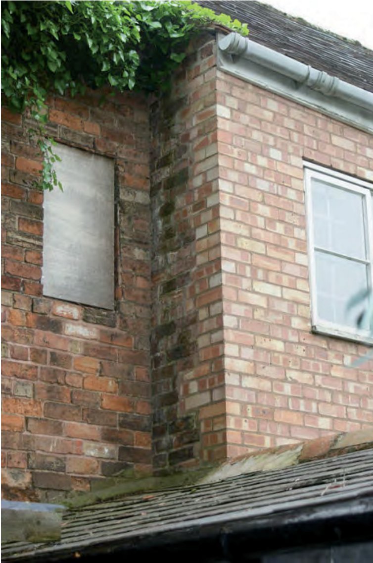
Plate 20: External gable showing early bricks in 35, Cowl Street
