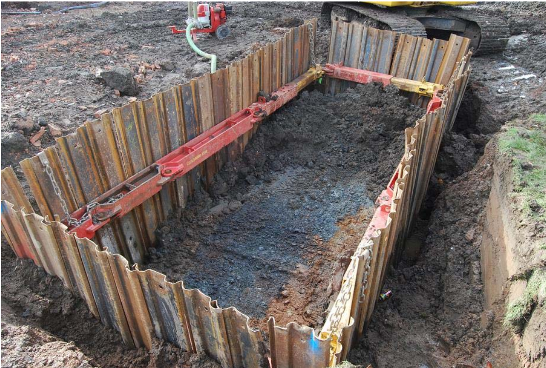
Plate 1 Trench 2 showing base of layer 202 View south-west
