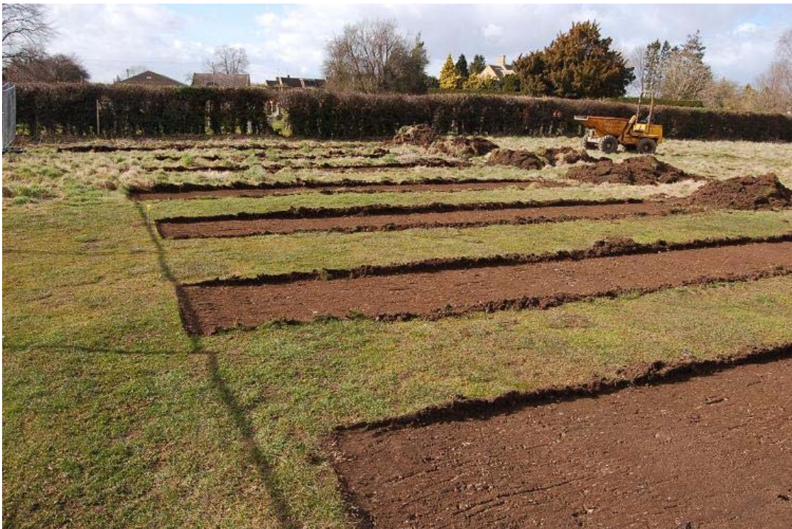
Plate 2: Interim site strip, view north west.
