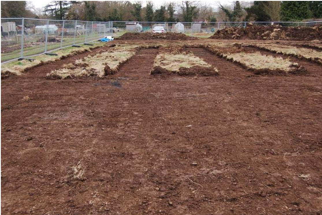
Plate 4: Interim site strip, view south west
