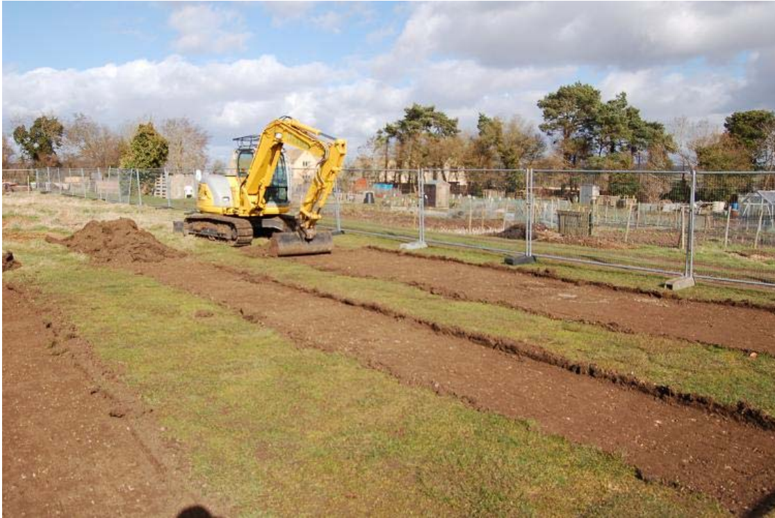
Plate 3: Interim site strip, view north west
