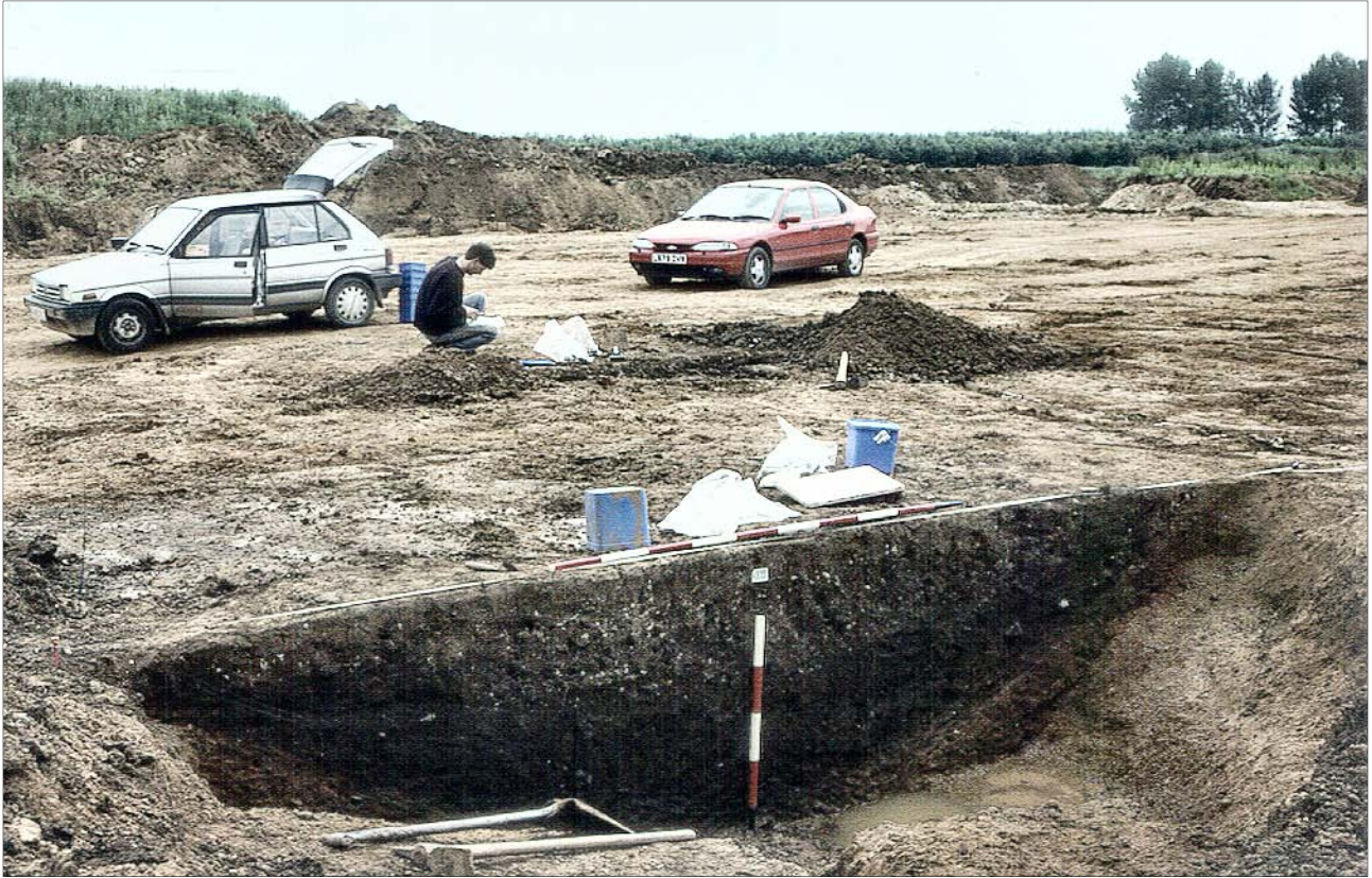
North facing section of Waterhole CG7 prior to machine excavation of lower fills
