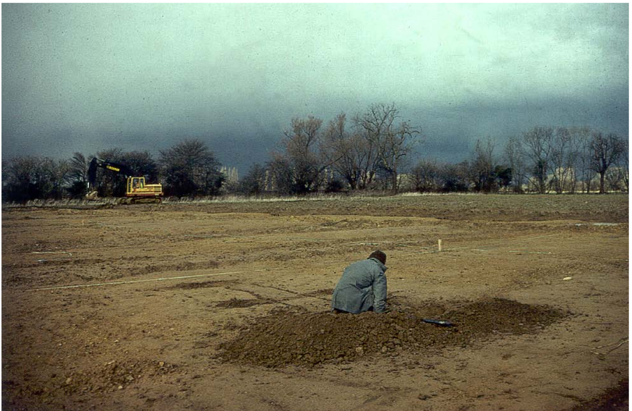
View showing typical conditions following topsoil stripping
