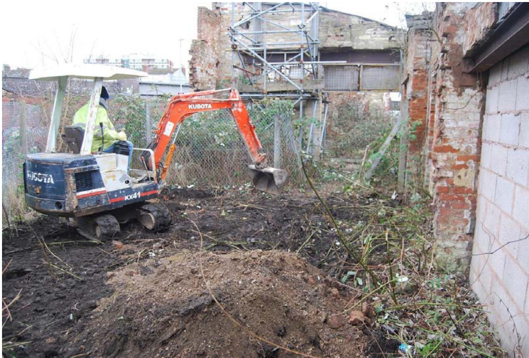
Plate 1 The western part of the site with Tanners' Hall in the background. Location of Trench 1 behind excavator. View from the west.
