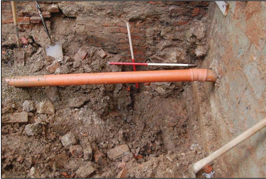
Plate 5 Platform for girder footings in the Western corner of courtyard showing building rubble and natural clay
