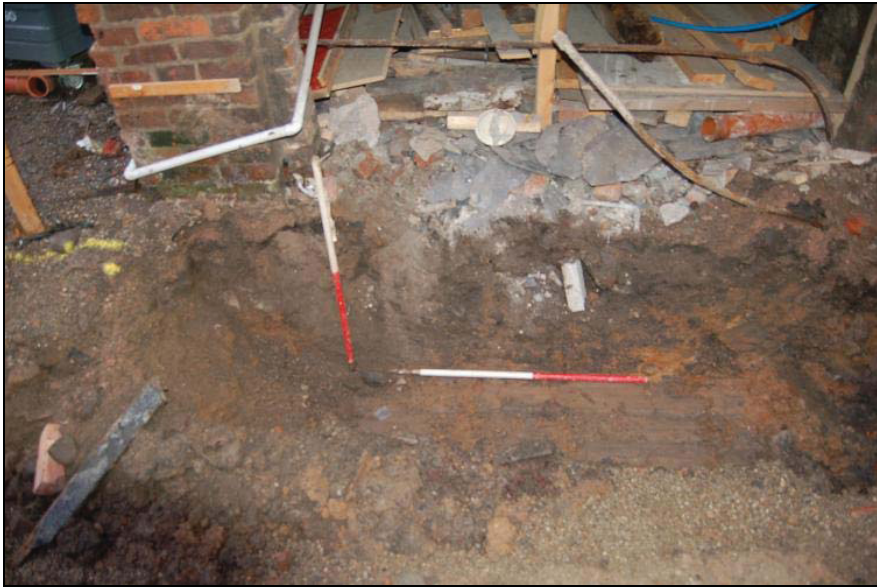
Plate 9 East facing section of foundation trench
