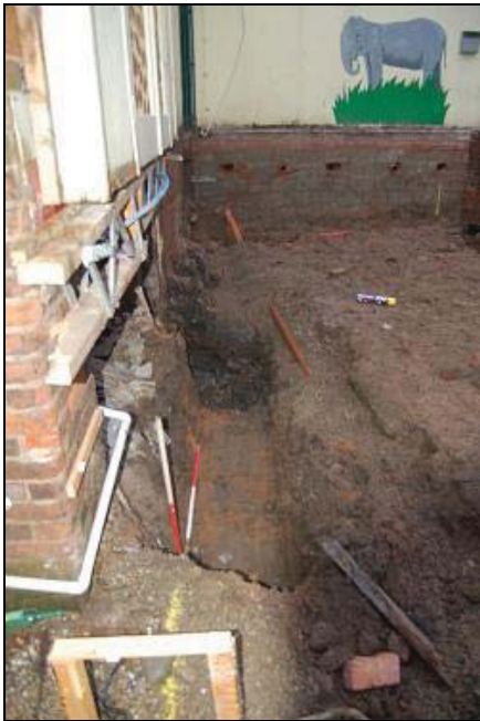
Plate 6 Northwest trench general view and new services connections
