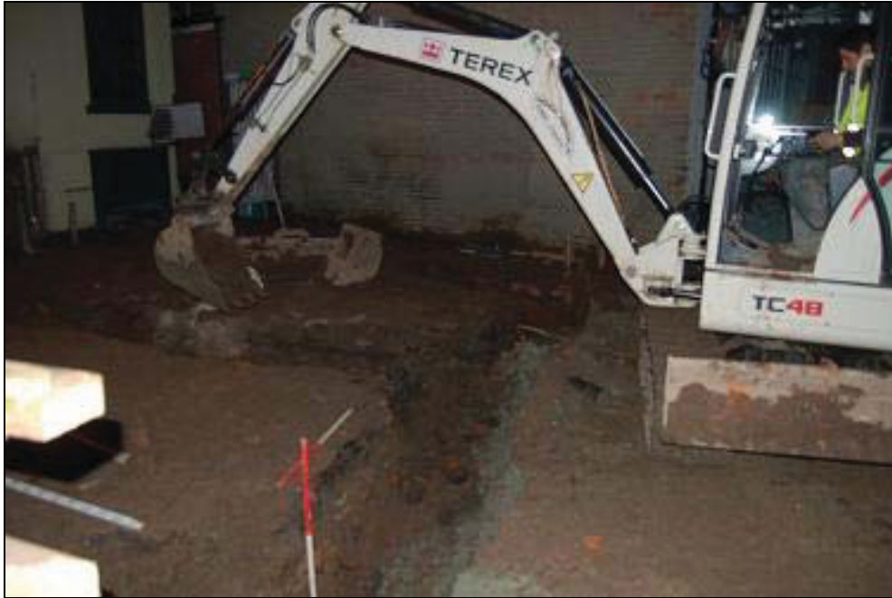
Plate 11 Overall trenches being completed
