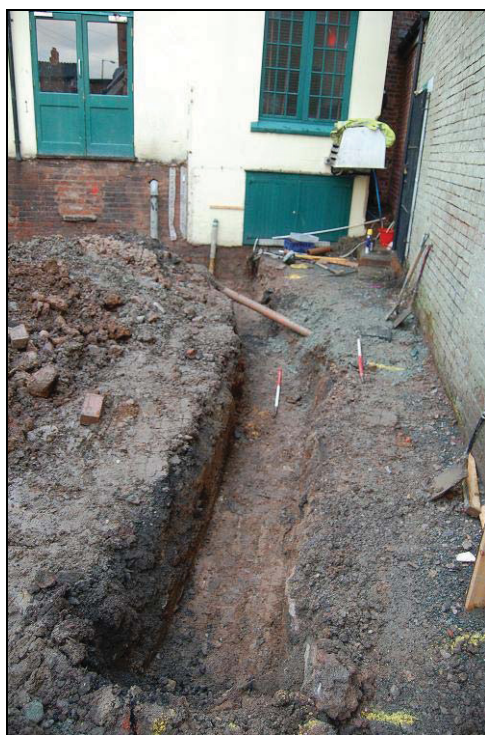
Plate 4 Northeastern trench completed looking north
