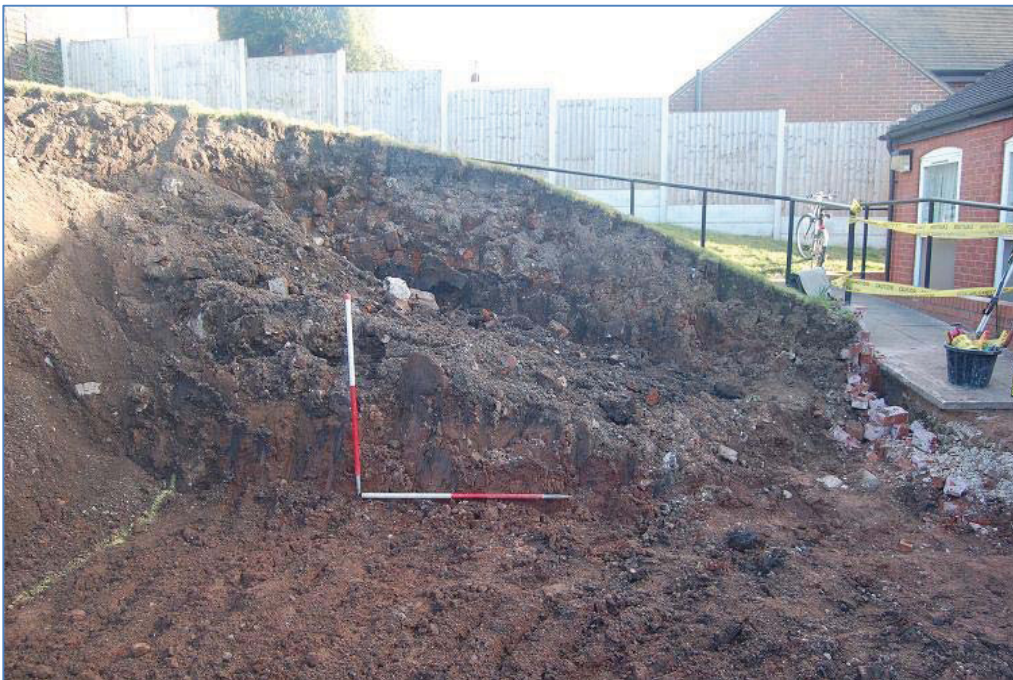
Plate 12 General view of Trench 2 during excavation looking southwest
