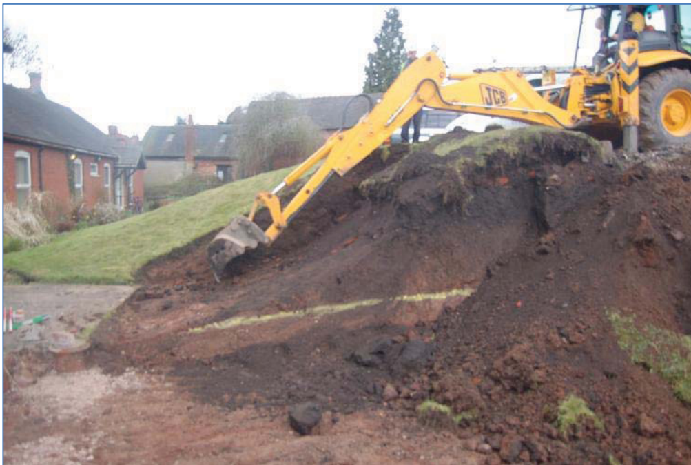
Plate 14 Trench 3 area for steps during excavation looking southwest
