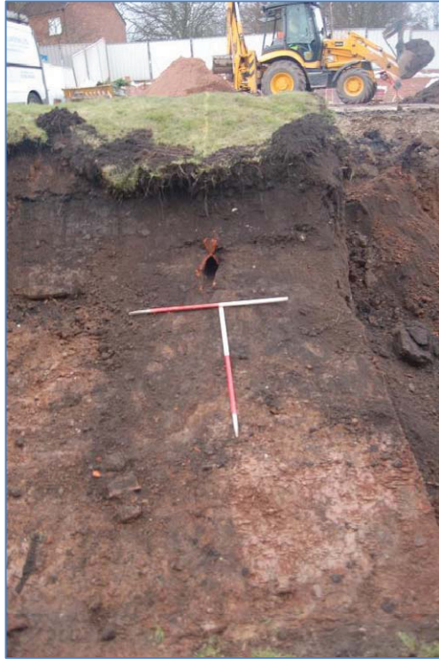
Plate 15 Modern ceramic land drain at the base of 302 in trench 3 during excavation looking north
