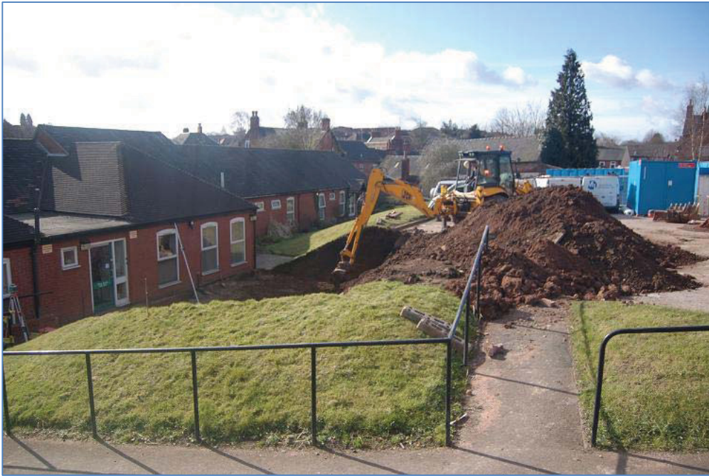
Plate 7 General view of Trench 2 during excavation looking southwest
