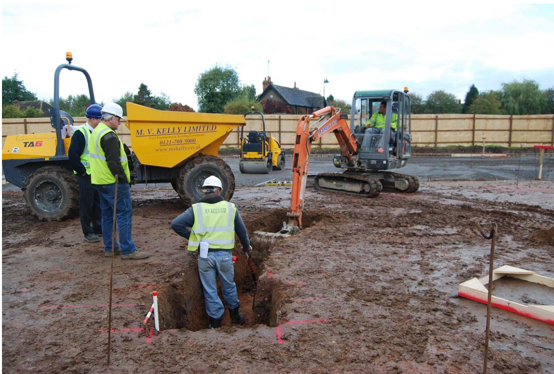
Plate 6: Trench 3 during excavation, from the south
