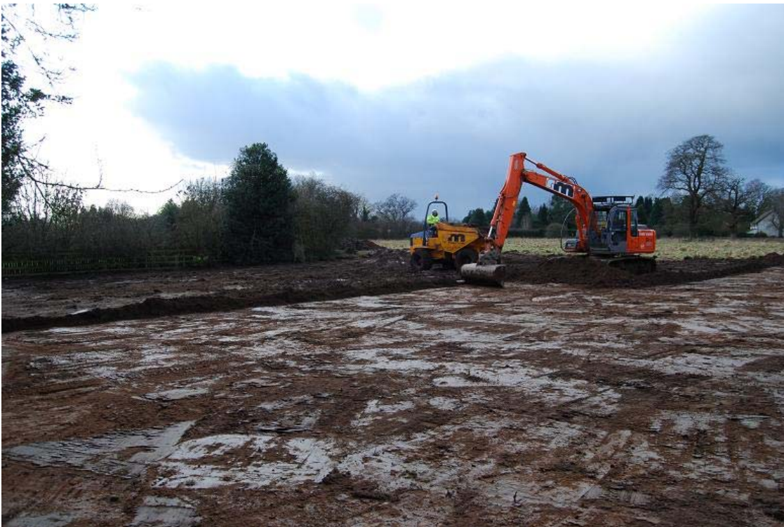
Plate 2: General shot Trench 1, from the south west
