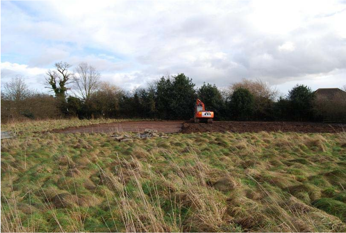
Plate 1: The site from the north east
