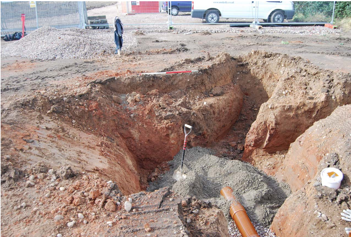
Plate 4: Trench 2, from the south east
